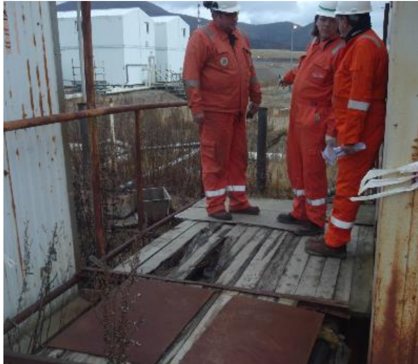
Photo 1. Derelict structures in close proximity to operation STP facilities
