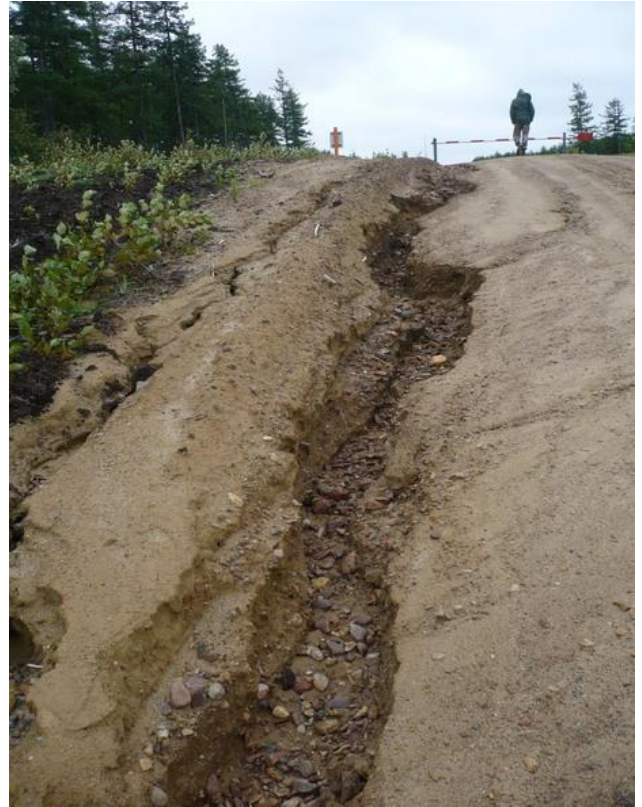
Photo 4 – View of erosion along access road to BVS.
