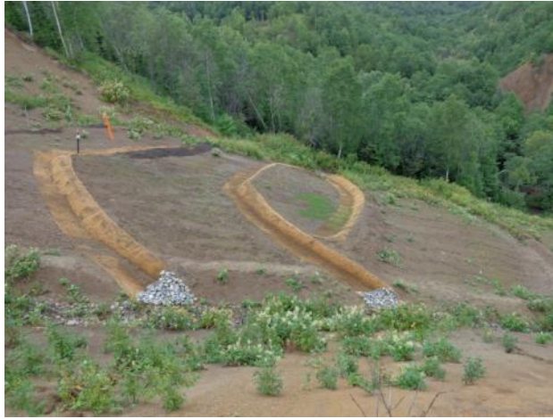
Photo 3 – View of the central portion of the southern slope shows area of recent repair with new slope breakers.
