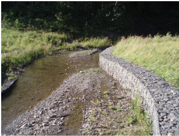
Photo 1 – View downstream showing Reno matting, gabion walls and the dense vegetation.
