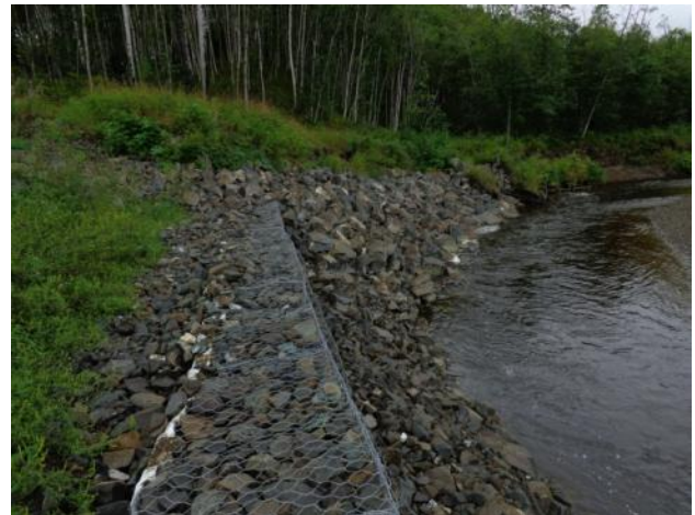
Photo 4 – View to the downstream direction showing the fortified south bank and silted and overgrown north bank.
