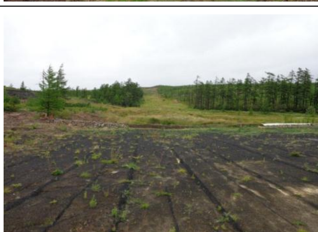
Photo 3 (left) – View to the south from the north slope showing fortified northern slope and a repaired slope breaker.
