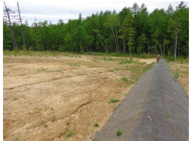
Photo 2 – View of poor vegetation cover and a misaligned slope breaker with erosion rills parallel to the breaker.
