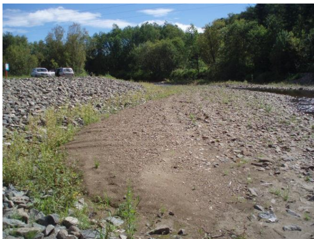
Photo 3 – Riprap on northern bank of river
