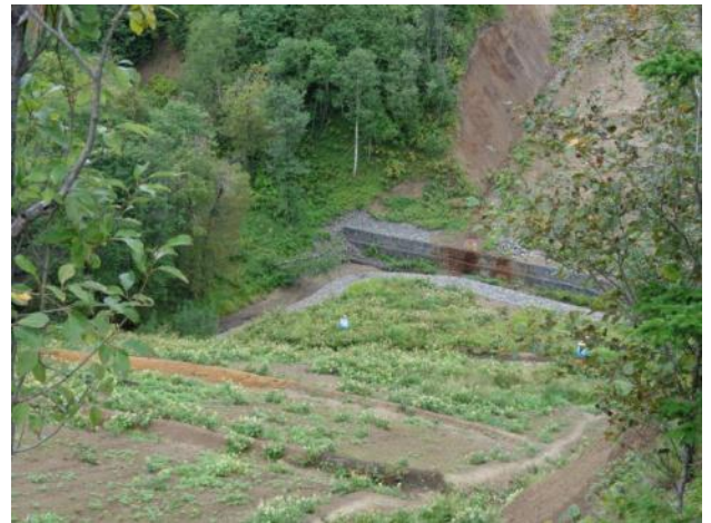
Photo 2 – View of southern slope with spotty vegetation at the bottom part and with slope breakers.
