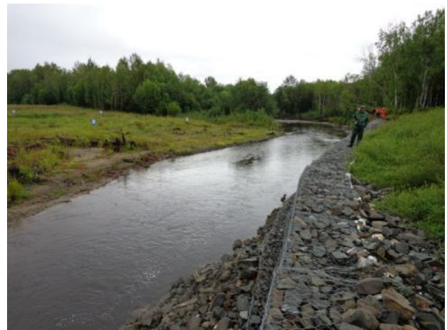
Photo 4 – View to the downstream direction showing the fortified south bank and silted and overgrown north bank.
