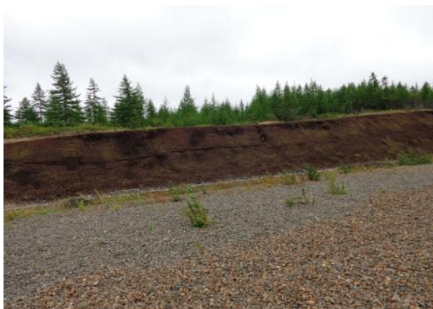
Photo 3 – View of north facing side cut with a horizontal failure of the geonetting.
