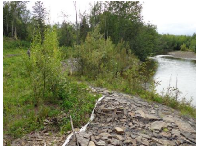
Photo 2 – View of the southern bank showing Reno mats with vegetation breaking through and a depression above the oil pipe trench.
