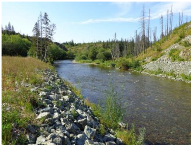
Photo 3 – View downstream showing well protected banks with heavy riprap on the west bank.
