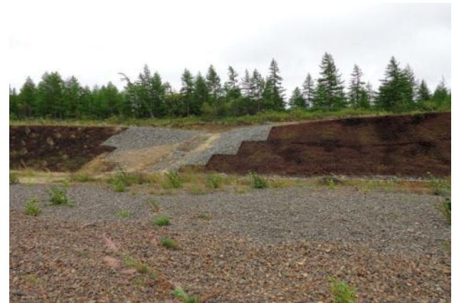
Photo 4 – Failed geonetting on side cut.
