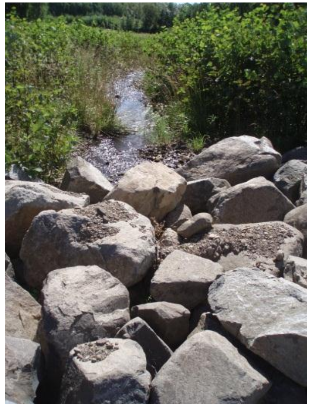
Photo 2 – View of the overflow channel riprap
