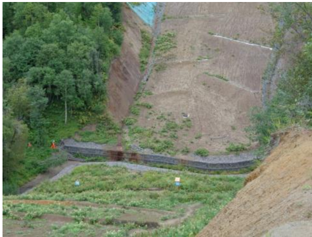
Photo 1 – View to the north across the river showing gabion walls and the north slope with very little vegetation cover. Note sediment flow over the gabion wall.
