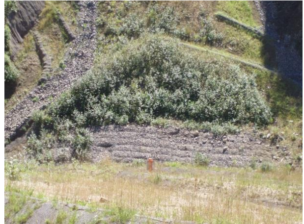
Photo 4 – View of southern slope showing tree growth above reno matting and also minor failure of the reno
