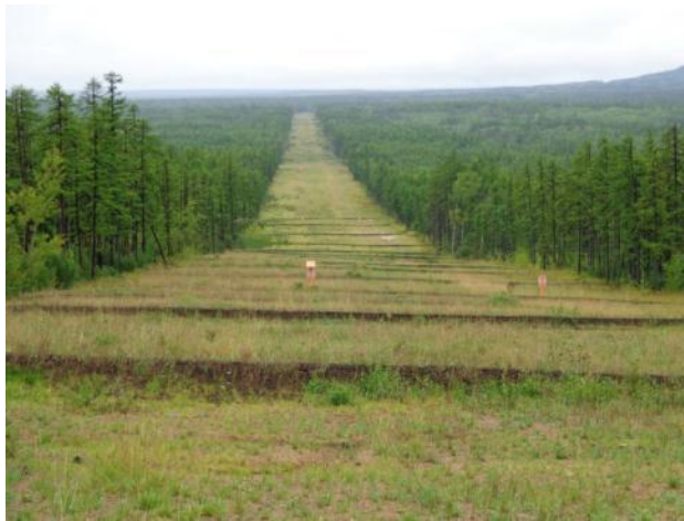
Photo 1 – View to the north showing good vegetation cover and good slope protection.
