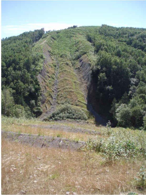
Photo 3 – View of southern slope showing more limited re-vegetation on lower portions and side cuts
