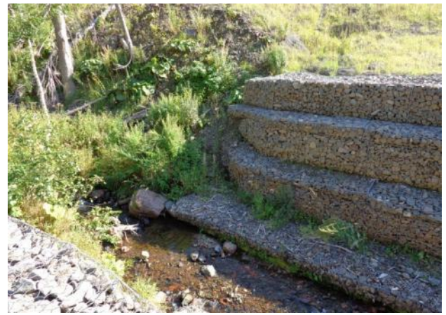
Photo 4 – View to the upstream showing the toe of the gabion wall at the impact point of the stream.
