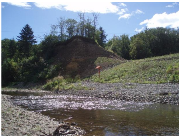
Photo 3 – Riprap on northern bank of river
