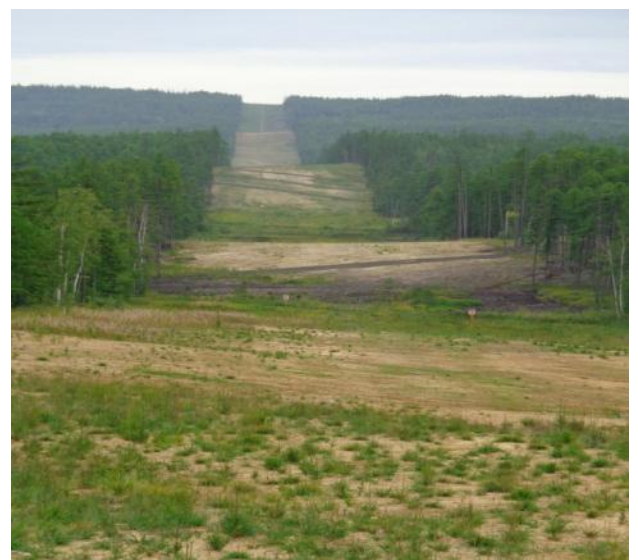
Photo 3 (right) – View to the south showing partially vegetated RoW with poor coverage on the upper elevations and better coverage on the lower elevation.
