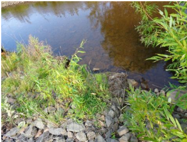
Photo 3 – View of the toe of the Reno mats at the upstream with damage at the leading edge.
