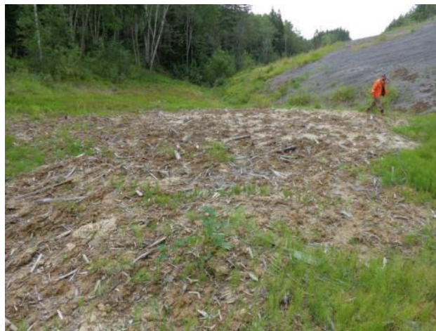
Photo 3 (right) – View to the south from KP 182 showing the side slopes with geojute and no vegetation cover.
