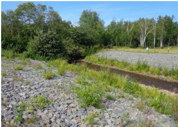
Photo 3 – View of the toe of the Reno mats at the upstream with damage at the leading edge.
