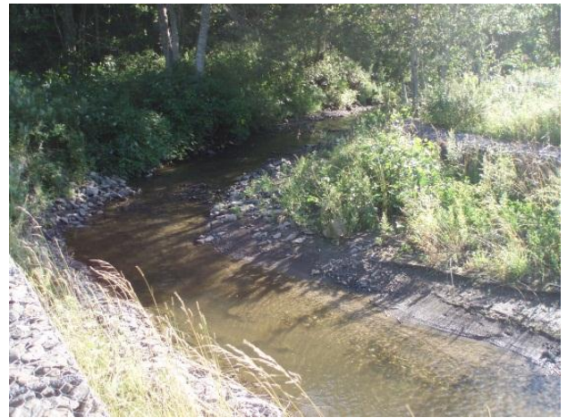
Photo 2 – View to the upstream showing Reno matting and gabion walls.
