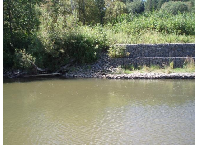
Photo 4 – Minor damage to downstream portion of gabion wall
