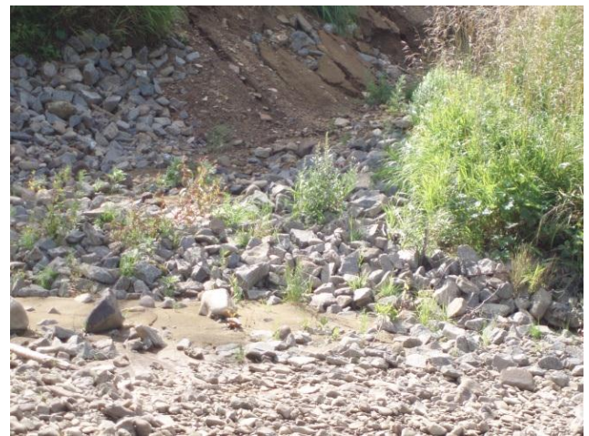
Photo 2 – Erosion around drainage channel on southern bank
