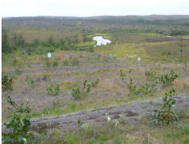
Photo 1 – View to the south showing the slope south of the crossing with slope breakers and good vegetation cover.
