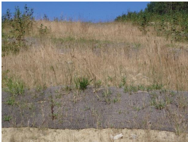
Photo 1 – View northern slope with vegetated RoW with fortified slope breakers.
