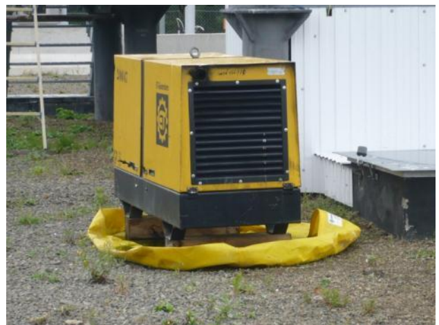
Photo 4 – Groundwater protection – generator at MOB-6
