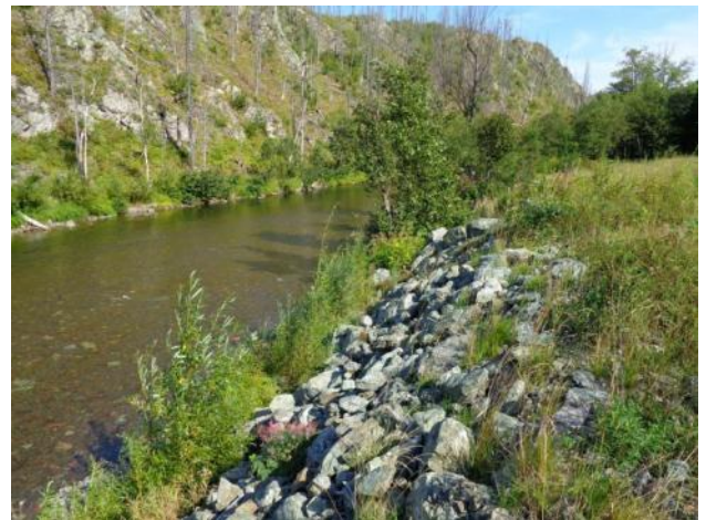
Photo 4 – View to upstream showing riprap and vegetation growing on the bank and through the rocks.
