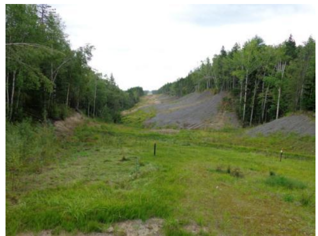
Photo 3 (right) – View to the south from KP 182 showing the side slopes with geojute and no vegetation cover.
