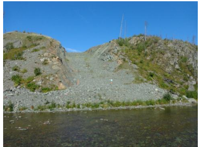
Photo 4 – View to upstream showing riprap and vegetation growing on the bank and through the rocks.
