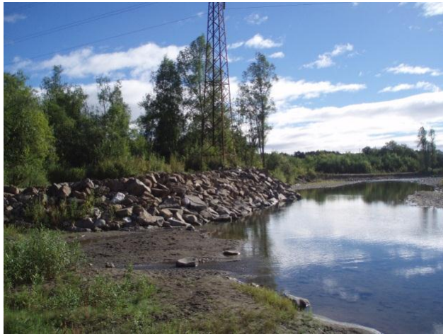
Photo 3 – Riprap protection around power pylon
