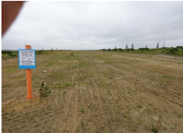
Photo 1 – View of the re-seeded RoW with scarified surface.
