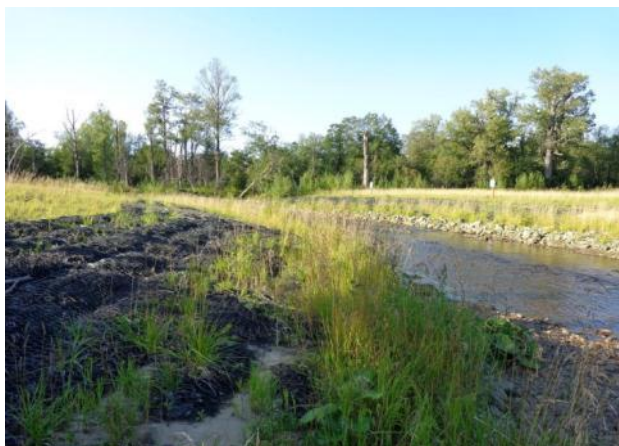
Photo 3 - View to the upstream showing protected banks and vegetation coming through the Reno mats
