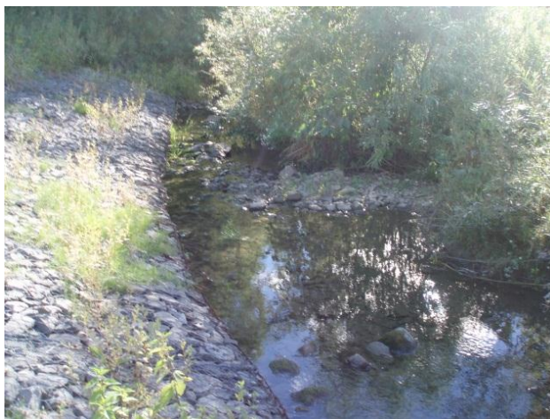
Photo 1 – View of the Reno mats on the north bank of the northern channel.
