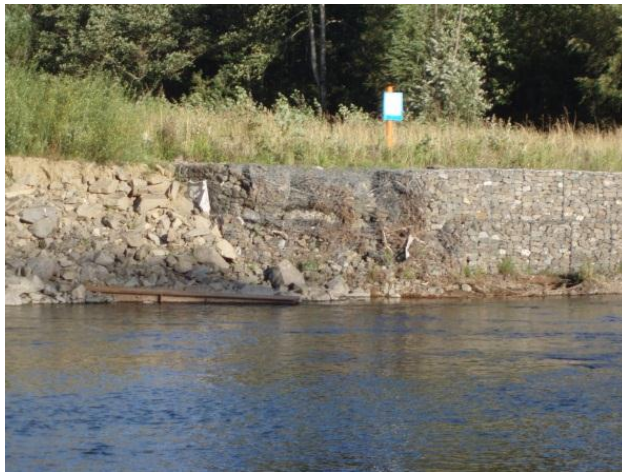
Photo 1 – View to upstream showing damage to the north bank gabion wall and good vegetation behind.
