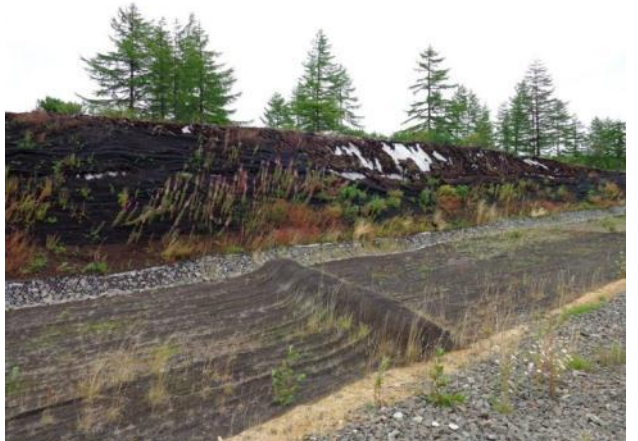
Photo 4 – Failed geonetting on side cut.
