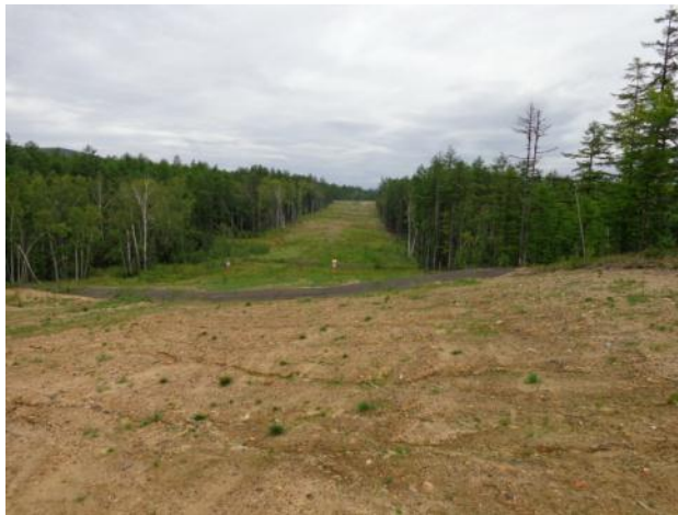
Photo 3 (right) – View to the south showing partially vegetated RoW with poor coverage on the upper elevations and better coverage on the lower elevation.
