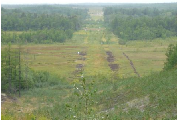
Photo 1 – View to north across the river crossing showing partially recovered wetlands and vegetated slope and side cut.
