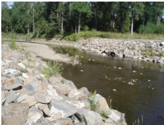
Photo 3 – Riprap on northern bank of central stream
