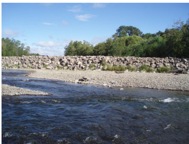
Photo 3 – Riprap on northern bank of central stream
