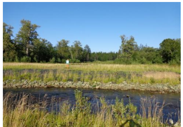
Photo 4 – View across the river to the south Showing well protected river bank with riprap and Reno mats.
