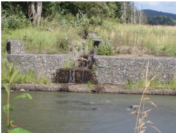
Photo 3 – View of Drainage ditch with northern bank gabion wall.
