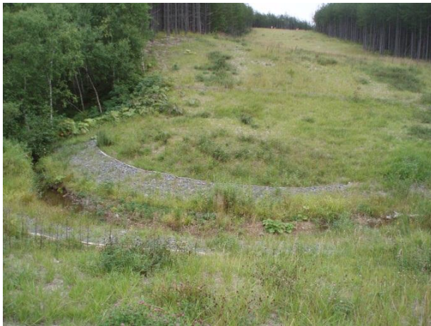
Photo 3 – Showing slopes with slope breakers but some areas of patchy re-vegetation
