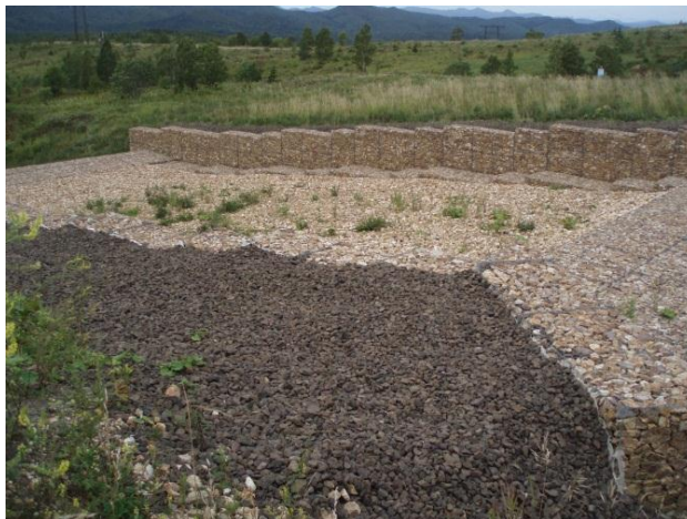
Photo 5 – Hard engineering of ephemeral drainage channel
