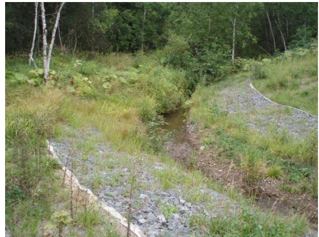
Photo 2 – Reno matting on the riverbanks with vegetation growth through.
