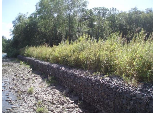
Photo 2 – View of southern bank gabion walls.
