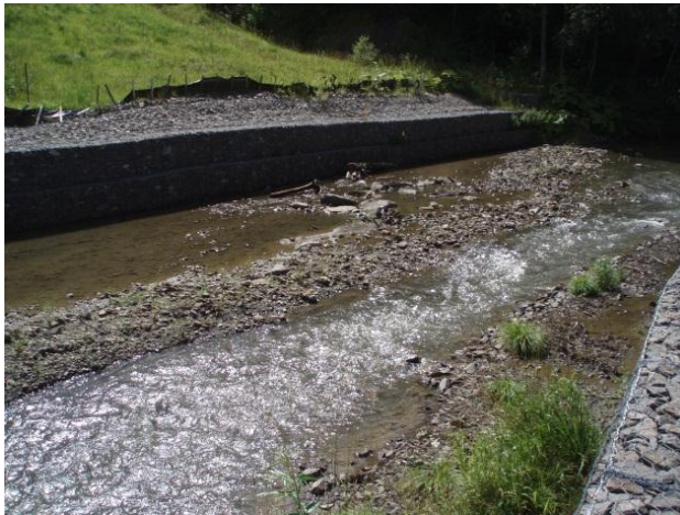
Photo 3 – View south showing the south slope with generally good vegetation cover, but bare side slopes and silt fencing in need of repair.
