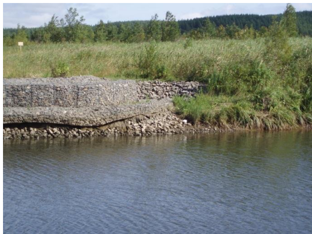
Photo 5 – Gabion on north slope with minor slumping
