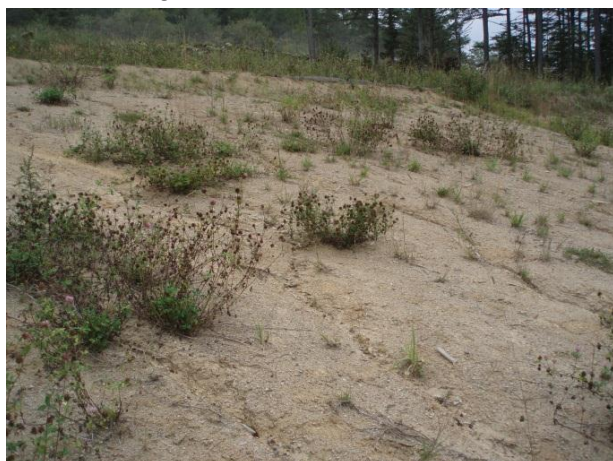
Photo 3 – View of erosional rill development and lack of grass cover.
