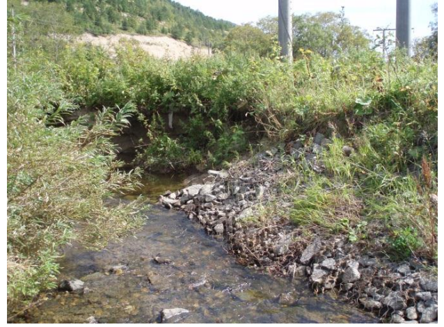
Photo 4 – Minor damage to reno matting
