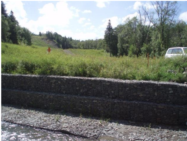
Photo 1 – View to the downstream showing gabion walls and Reno matting. Good re-vegetation on RoW.
