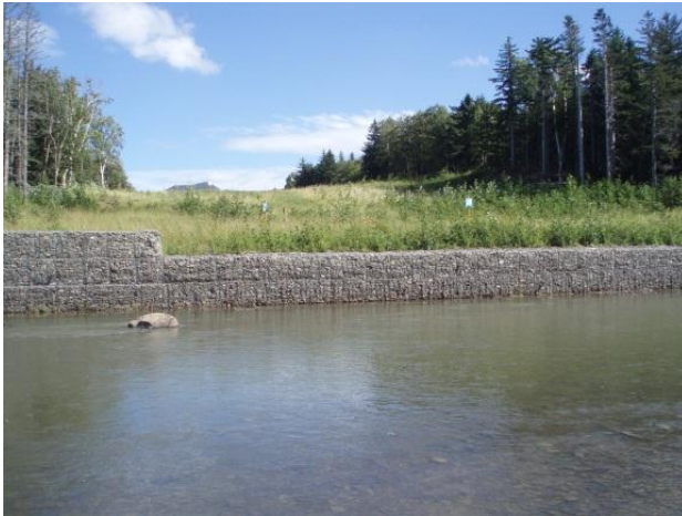
Photo 3 – Erosion and gabion damage on the northern bank
