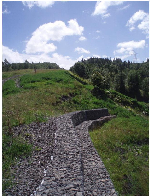
Photo 2 – View of gabion wall
