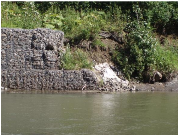
Photo 3 – Erosion and gabion damage on the northern bank
