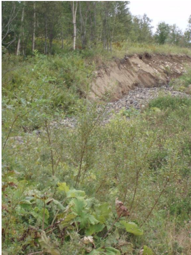
Photo 5 – Hard engineering of ephemeral drainage channel
