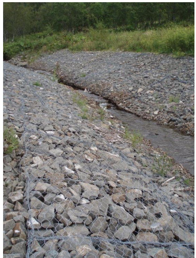
Photo 2 – Reno matting on the main stream leading to narrowing of the channel.
