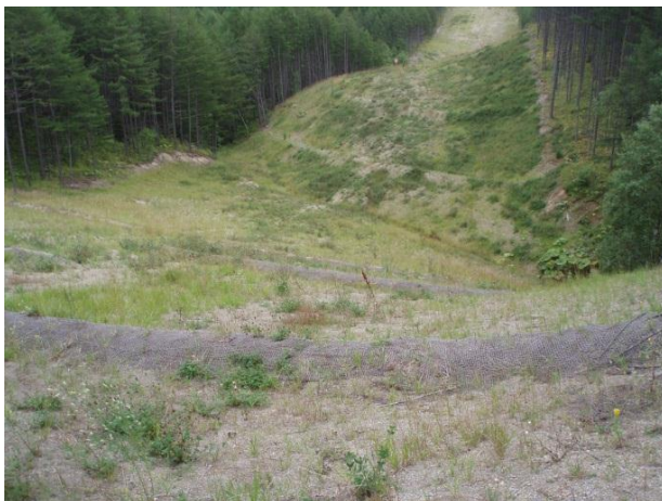
Photo 3 – Showing slopes with slope breakers but some areas of patchy re-vegetation
