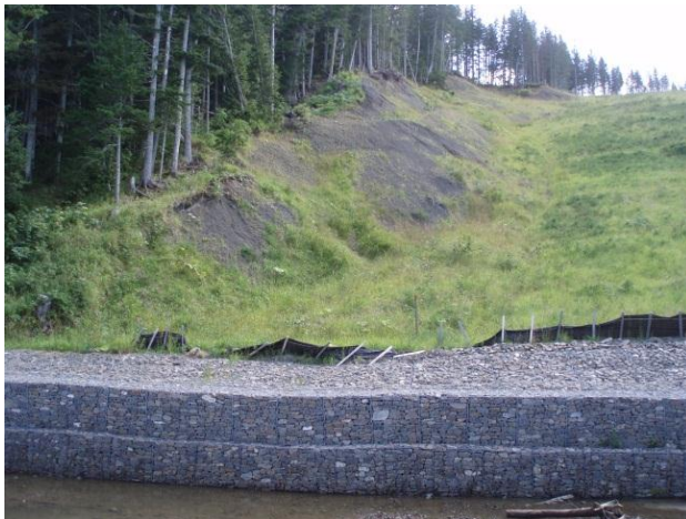
Photo 3 – View south showing the south slope with generally good vegetation cover, but bare side slopes and silt fencing in need of repair.
