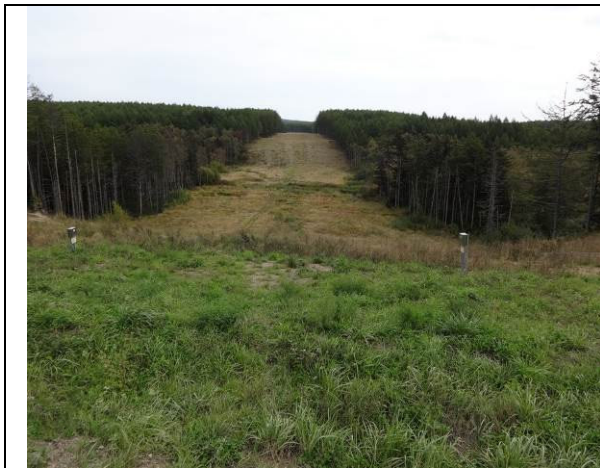
Photo 1 – View south across the river showing good vegetation cover and slope breakers on the slopes.
