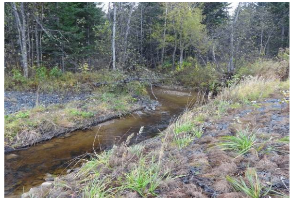
Photo 2 – View to the upstream showing stable banks and ground cover on the Reno mats.
