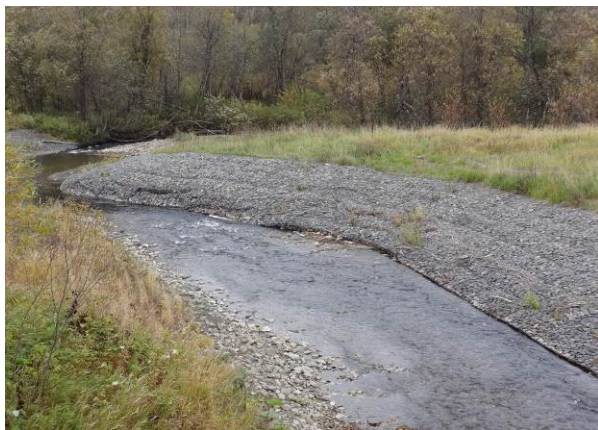
Photo 1 – View downstream showing damaged Reno matting on the west bank.
