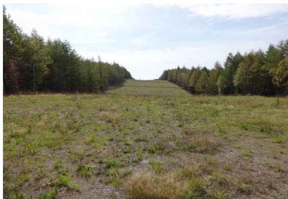
Photo 1 – KP 607 - View to the north of good vegetation cover and slope breakers
