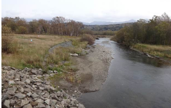
Photo 1 – View downstream showing Reno matting on the north and slightly undercut matting on the south.
