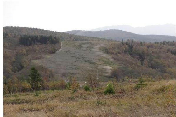
Photo 2 – View to the south past MOB 17 showing RoW slope with good slope breakers but with poor vegetation cover.
