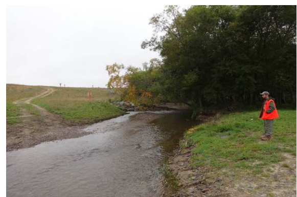
Photo 2 – View to the upstream showing the south bank partially damaged by driving up the Reno mats.
