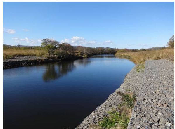
Photo 2 – View upstream showing gabions and vegetation on the bank.
