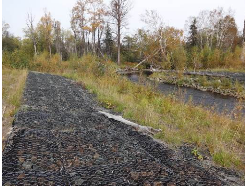
Photo 4 - View to the downstream showing protected banks and vegetation coming through the Reno mats
