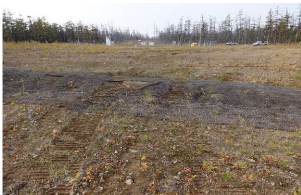
Photo 3 – (to left) View of damaged slope breaker by an unknown activity of tracked vehicle.
