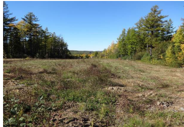
Photo 2 – View of fully deforested RoW. Note disturbed soil by the use of heavy equipment for the tree cutting.
