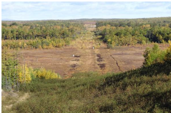
Photo 1 – View to north across the river crossing showing partially recovered wetlands and vegetated slope and side cut. Note the dense population of Alder on the slope leading to the valley.
