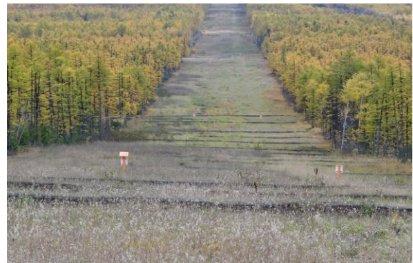
Photo 2 – View to the south showing sandy slopes with grass cover and good slope breakers.
