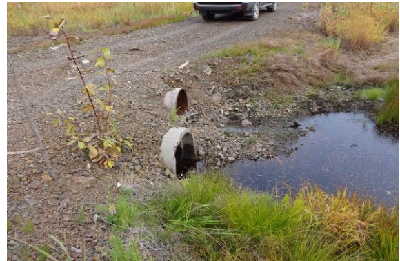
Photo 6 – View of repaired flume pipe(s) in the wetlands across the access road to NOB 24.
