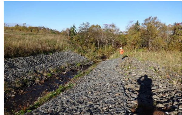
Photo 4 – Hard engineering of seasonal drainage channel and good vegetation cover
