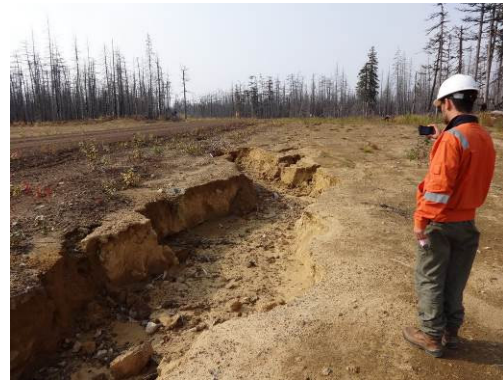
Photo 3 – (to left) View of damaged slope breaker by an unknown activity of tracked vehicle.
