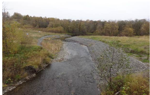
Photo 2 – View to the down stream showing Reno mats on both banks and well vegetated RoW.
