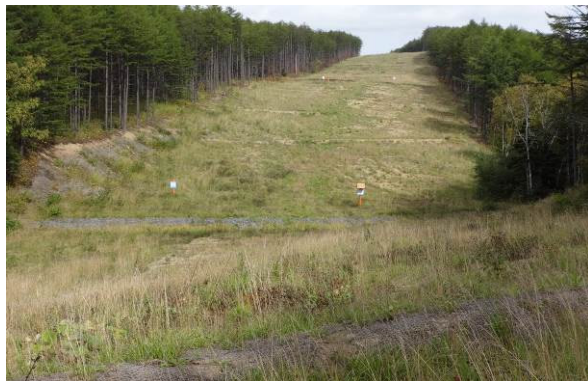
Photo 1 – View to the south showing the river crossing and slope protected with slope breakers.
