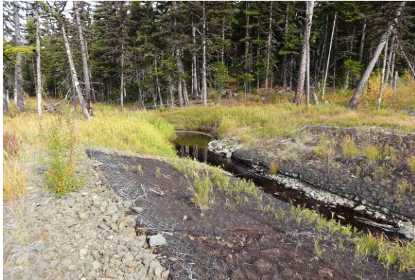
Photo 3 – View to the downstream showing the river banks with Reno mats.
