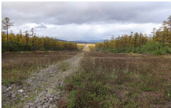
Photo 1 – View to the north showing good vegetation cover and a central drainage channel to improve drainage on the slope.
