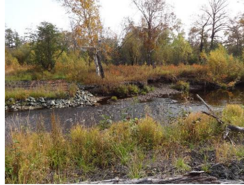
Photo 5 – View across and upstream of the river showing stable vegetated banks with Reno mats.
