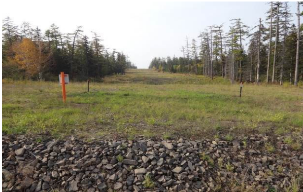
Photo 1 – View to the southwest showing stable road cut, good slope breakers and good vegetation cover.
