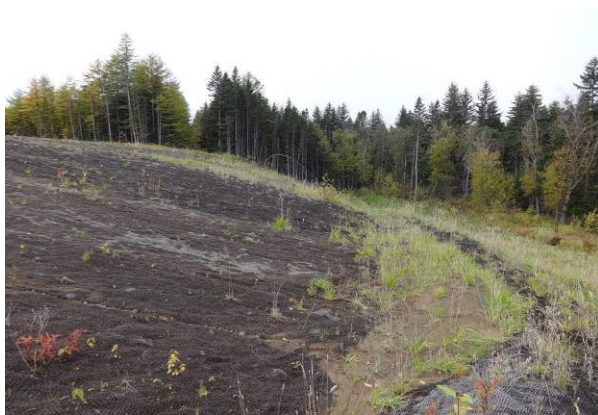
Photo 5 (left) – View of the very top of the slope next to the access road showing slope protection with Geojute but mostly without vegetation.
