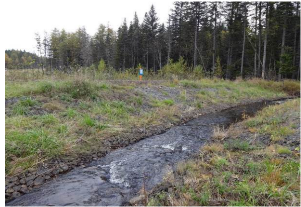
Photo 4 – View to the north showing the RoW slope towards the access road with good ground cover and slope breakers.
