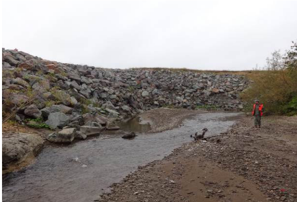
Photo 3 – View upstream from the RoW showing bank protection with large riprap.
