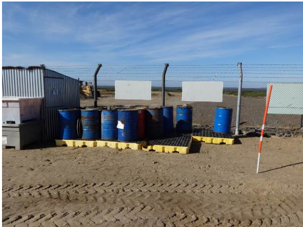
Photo 3 – View of drum storage on top of drip trays.
