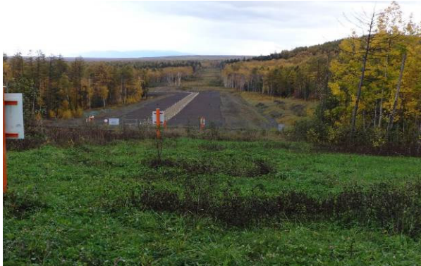
Photo 1 – View to the south showing fault crossing with good vegetation surrounding the trenches and good ground cover on the RoW.
