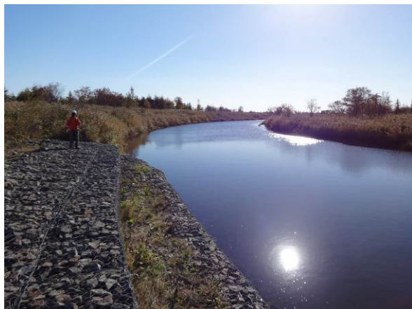
Photo 1 – View downstream showing gabion wall on the north bank
