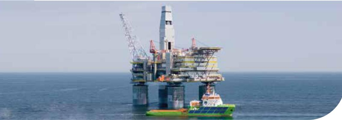
The Piltun-Astokhskoye-B (PA-B) offshore oil and gas platform is the largest platform built under the Sakhalin-2 project. It was installed in 2007 in Piltun area of the Piltun-Astokhskoye field 12 km from the shore at the depth of 32 m and 80 km to Okha.
