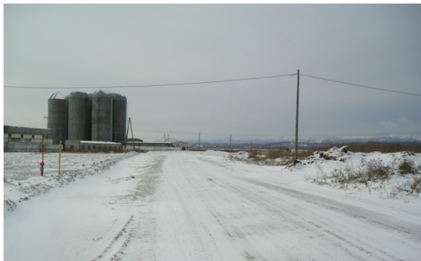
Road from the camp to the construction site
