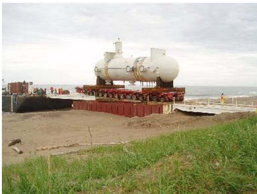
Figure 14.4 Transfer of gas/liquid receivers over dock barge and ramp using Self-propelled Motorised Transport
