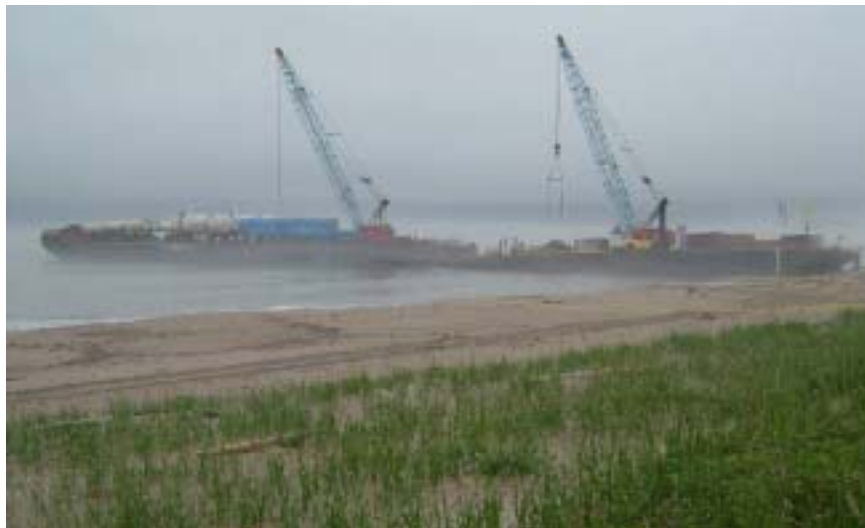
Figure 14.3 Side view of barges at BLF
