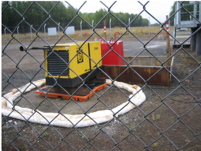
Photo 12 Temporary diesel generator and fuel day tank at block valve station PGB4
