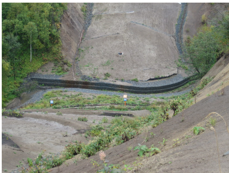
Photo 4 Example of damaged and missing silt fence on a slope with little or no vegetation – Kormovaya River (KP – 351)
