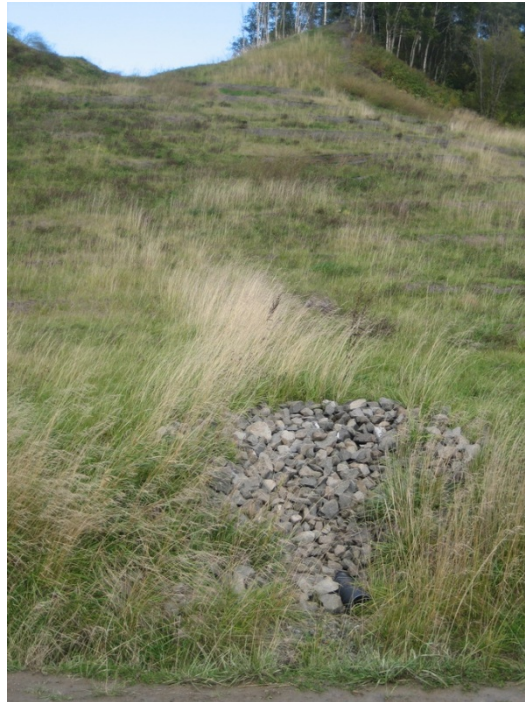
Photo 5 Sovetskoy Ridge example of internal drain
