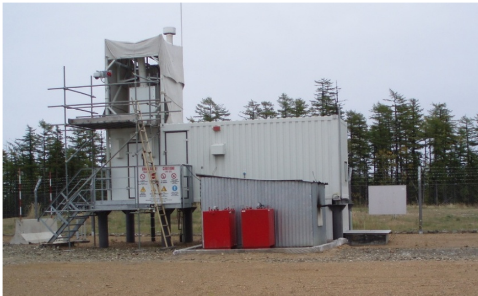
Photo 13 Temporary diesel generator and fuel day tank at block valve station NOB17
