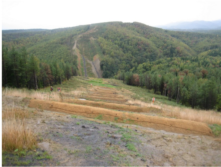
Photo 1 Repaired slope breakers on access road in Gar River slope
