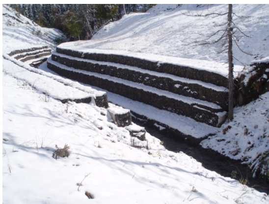
Photo 10 Gabion wall in good condition at the R. Vstrechny
