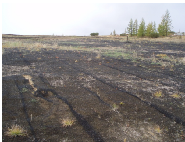
Photo 3 Use of geotextile on sandy slope near the R. Khandusa
