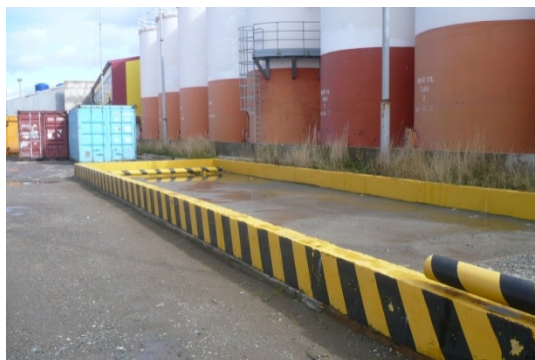
Photo 20 Bunded tanker loading area
