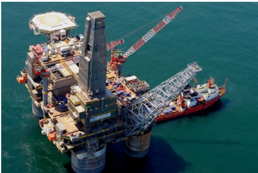
Figure 1 Photo of LUN-A Platform
