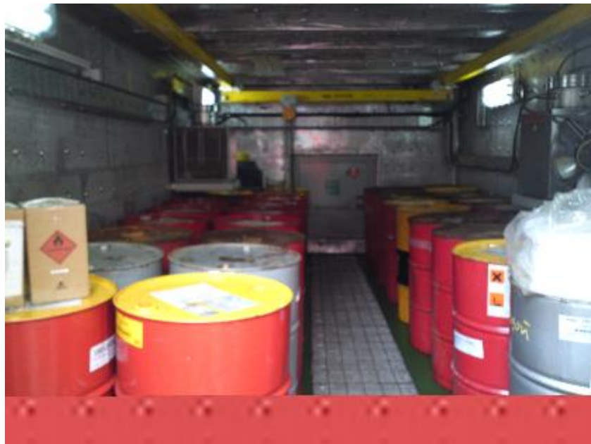
Photo 4. Dedicated lube oil storage container (installed 2014)
