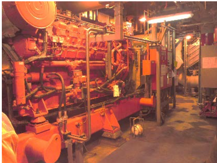
Photo 12. One of two fire water pumps (diesel-fired)
