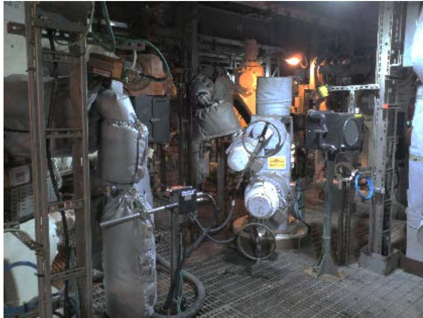
Photo 9. Cuttings Re-Injection Well (currently not in use – under assessment)
