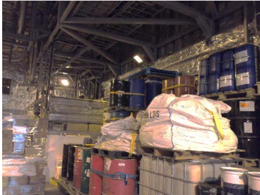
Photo 13. Chemical storage area in Drilling Module (chemical drums on wooden pallets stacked three high and two deep)
