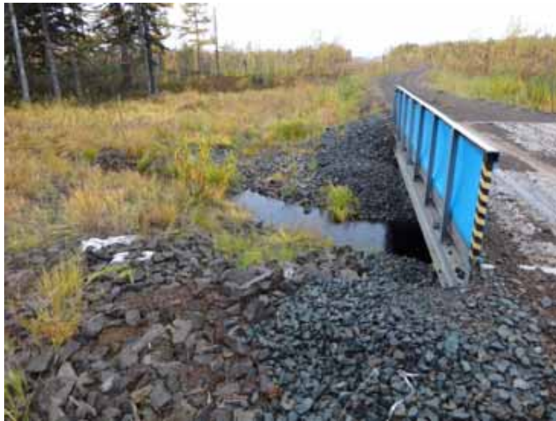
Photo 4. View of protected drainage with riprap and good vegetation cover.
