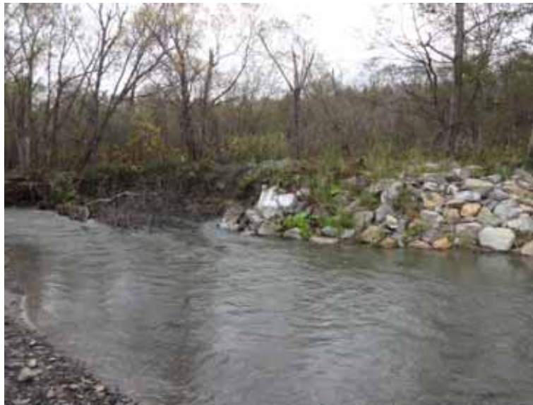
Photo 2. View of the north bank where the current is cutting into the bank behind the riprap protection layer.
