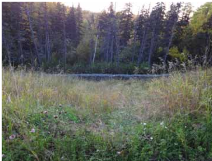
Photo 3. View to the side of the RoW showing gabion wall to stabilise slope.
