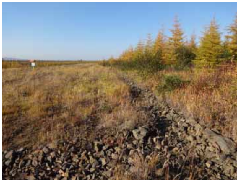
Photo 1. Showing rip rap lined cut off channel with a junction of a cross channel
