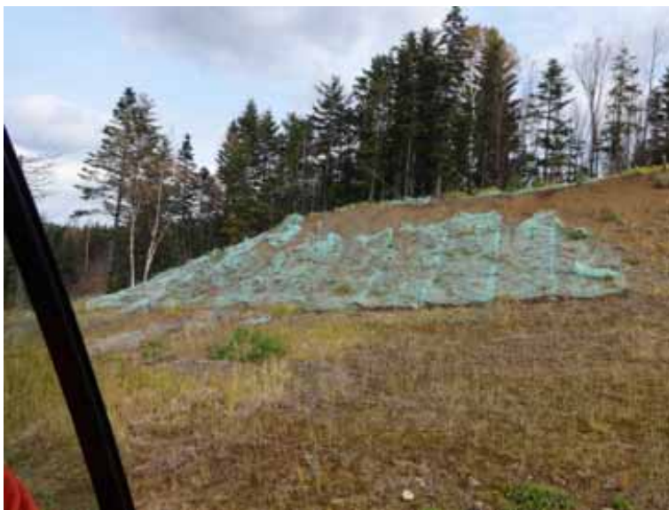
Photo 3. View of a RoW side cut with trees cut on the slope itself, and additionally failing geojute.
