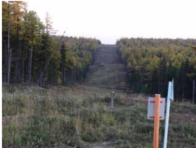
Photo 1. View of RoW showing good vegetation cover on the slopes
