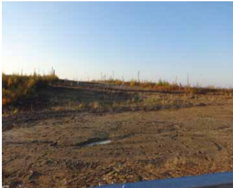
Photo 2. View to the north showing poorly vegetated sandy slope with slope breakers at the upper portion.
