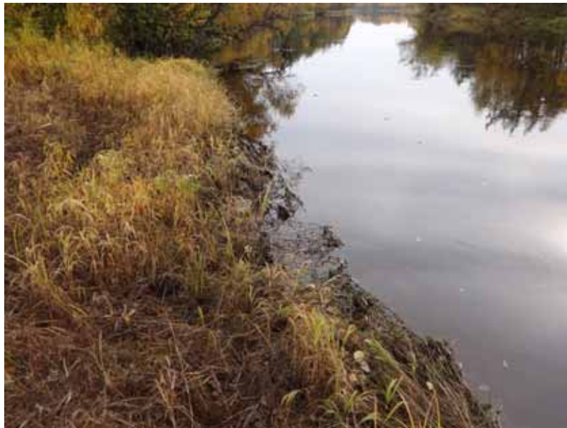
Photo 5. Close up view on the north bank of the river showing deterioration of Reno matting.
