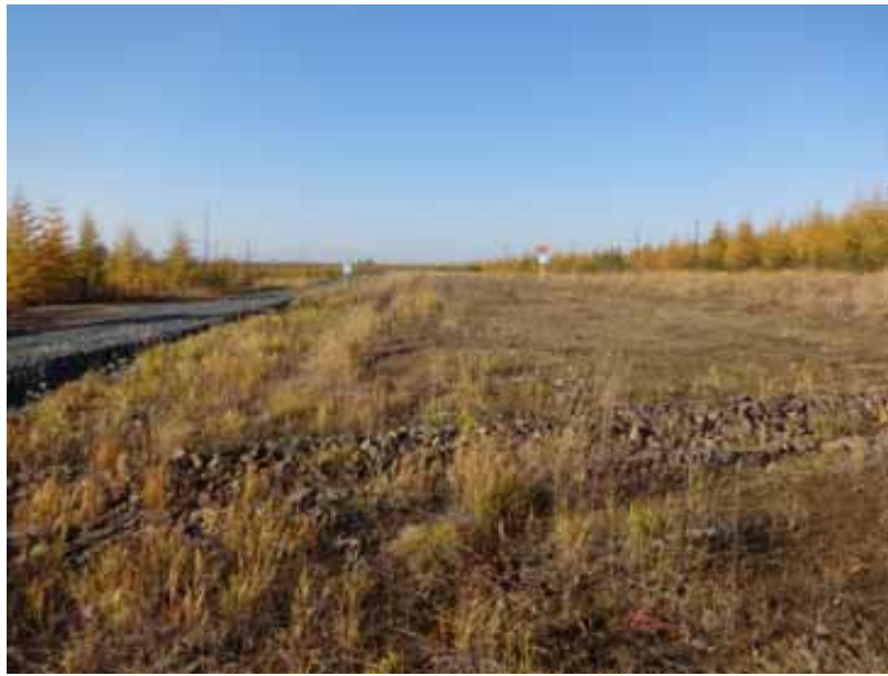
Photo 2. Showing cross channel leading to culvert under the access road
