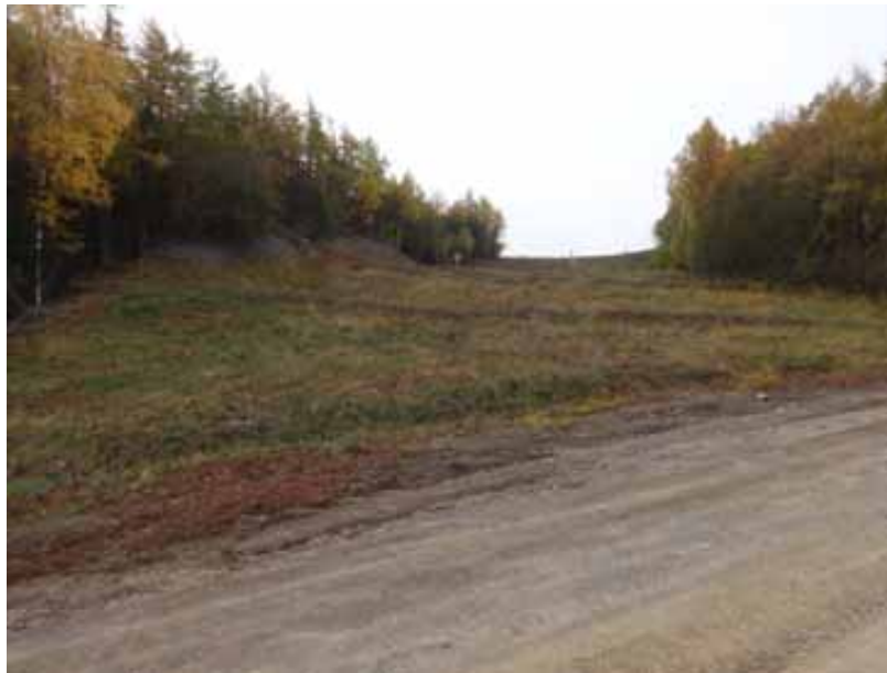
Photo 2. View to the south showing vegetated slope with slope breakers and removed tree saplings.
