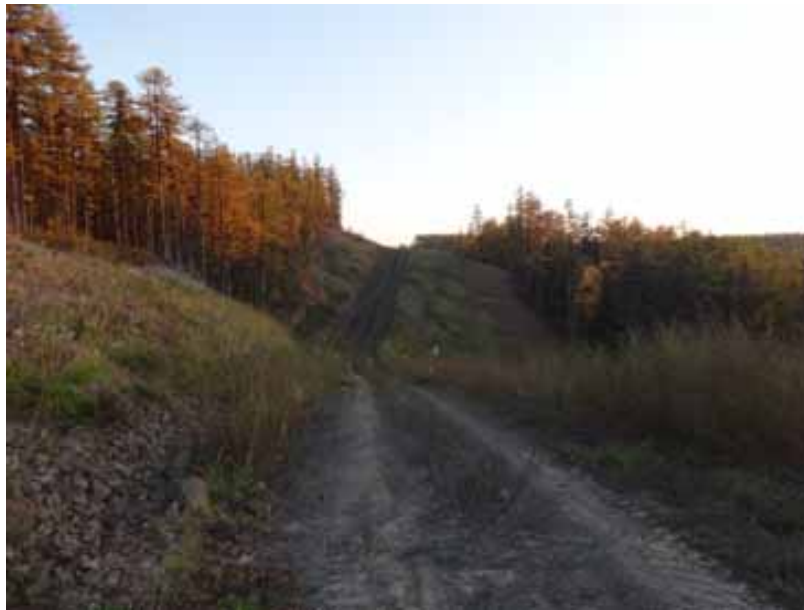
Photo 2. View of RoW showing slope protection and good vegetation
