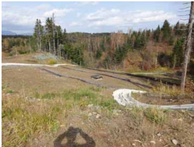
Photo 1. View from the RoW to the east of a repaired landslide area.
