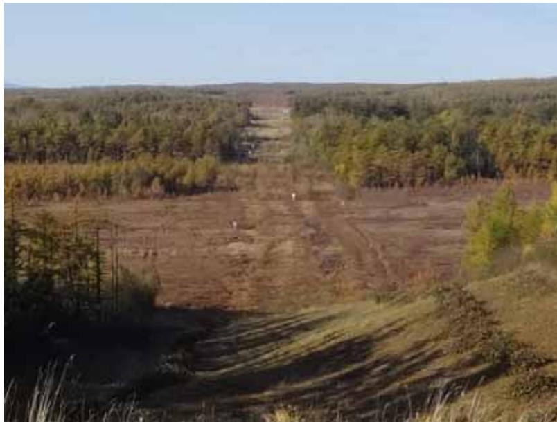
Photo 2. Oct 2014 View to the north at the Dagi River wetland.
