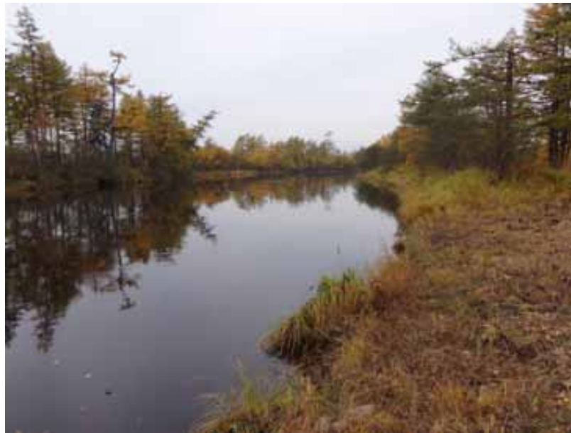
Photo 4. View to the upstream showing riverbanks with reno mats.
