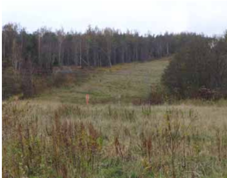
Photo 4. View to the south showing RoW and slope with good vegetation cover and slope protection.
