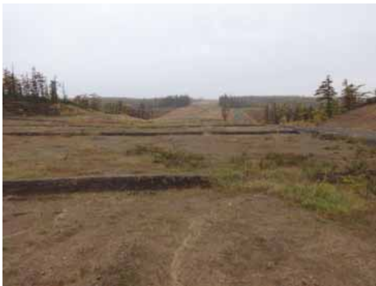
Photo 2. View west along the RoW showing vegetation and slope breakers.
