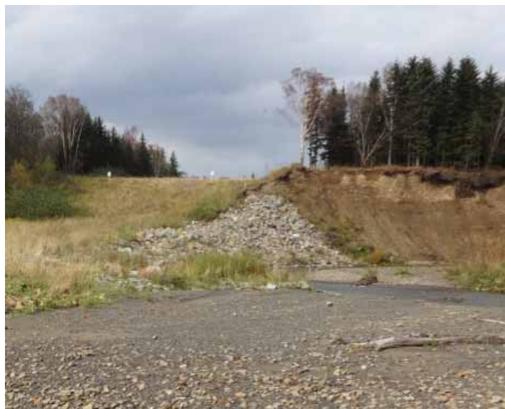
Photo 1. View of the repair of the riverbank at the band.
