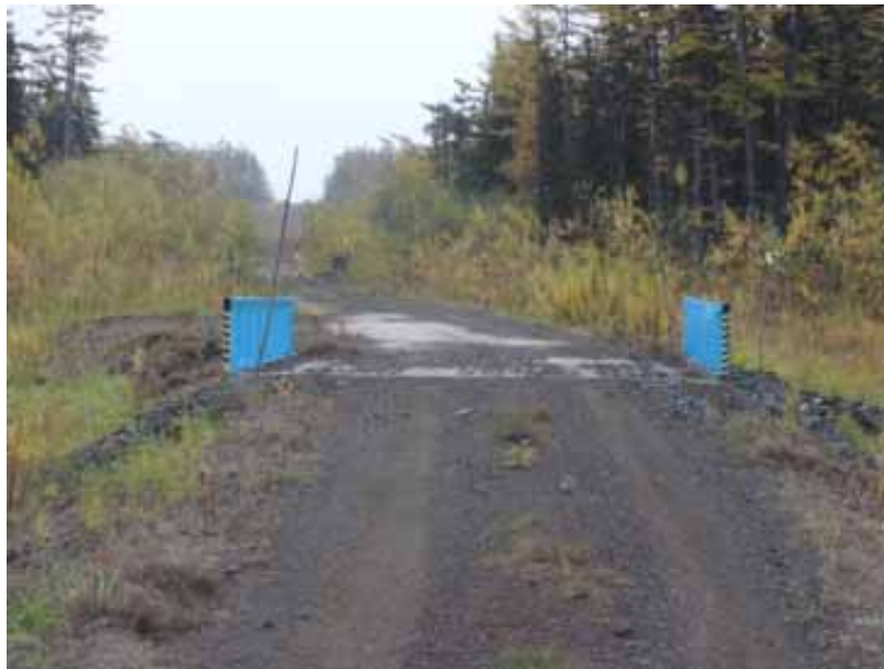
Photo 3. View of bridge and silt fence. Note the sapling rich area behind the bridge.
