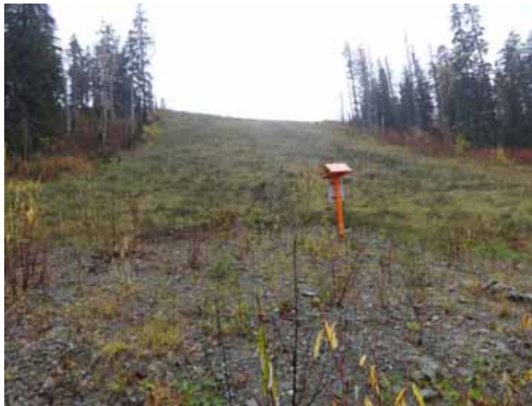
Photo 1. View to the south showing a steep slope of the RoW with good vegetation cover and slope protection.
