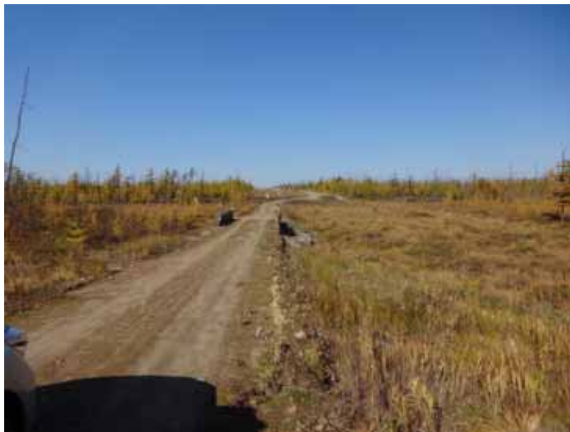
Photo 3. View to the north of a RoW on wetland and a bridge on a tributary of the Tomi River
