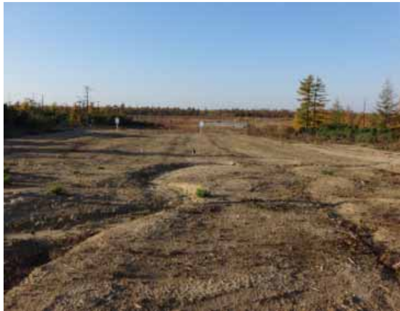
Photo 2. Showing erosion channel.
