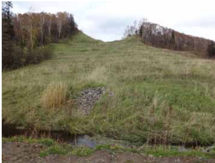
Photo 1. View of the slope to the north showing good vegetation cover. Note the outlet of a subsurface drain at the bottom of the slope.
