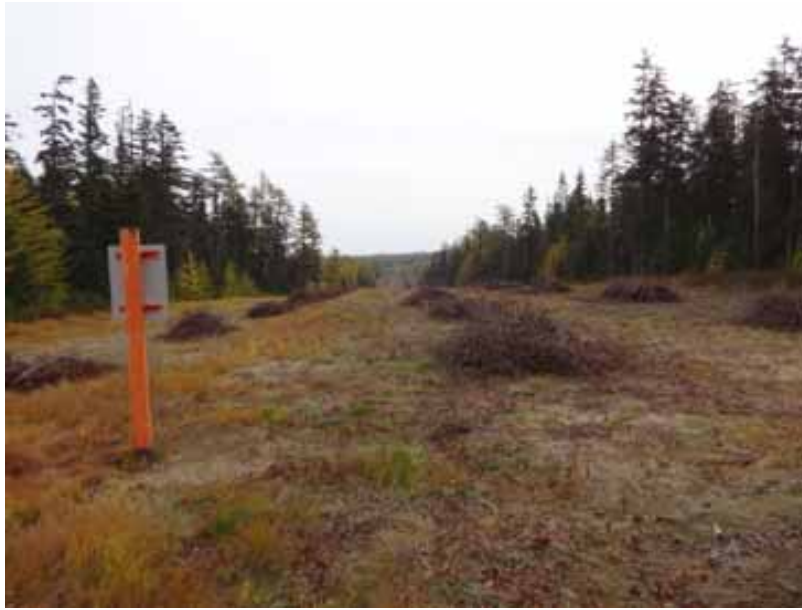
Photo 2. Close-up of effective tree sapling removal with grass left intact. Note the piles of cuttings awaiting mulching.
