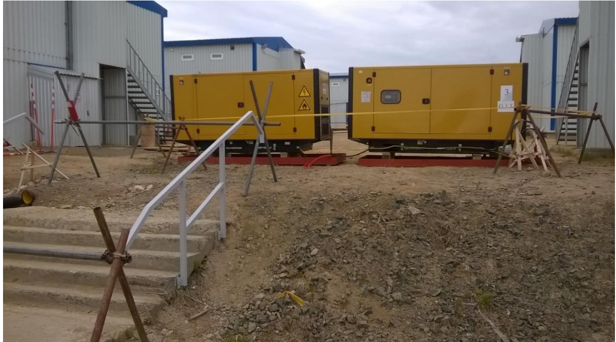
Photo 8 Generators with drip trays
