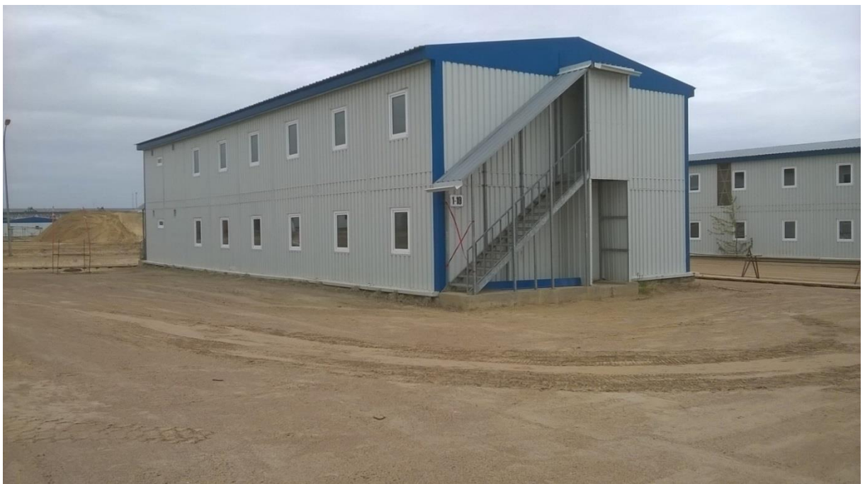
Photo 2 Building not being refurbished due its current condition – note red tape blocking entrance
