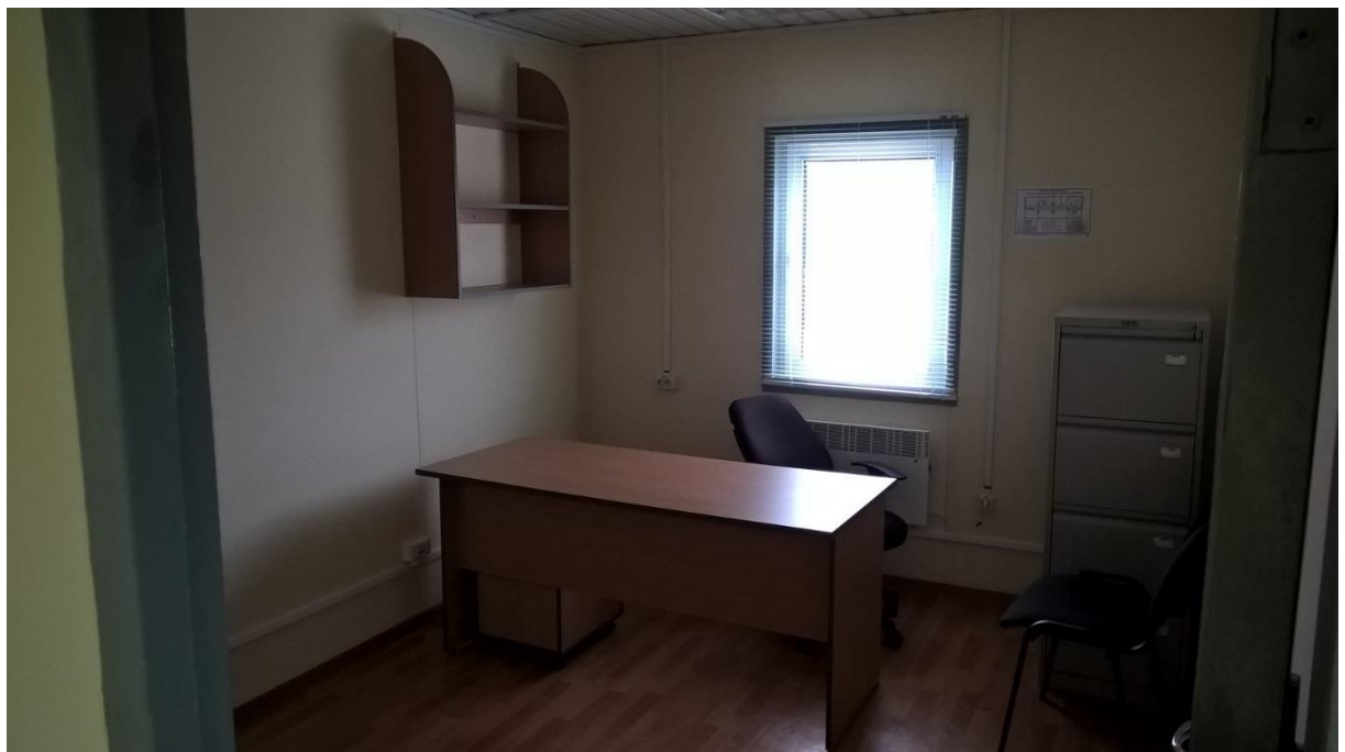
Photo 4 Refurbished office in building
