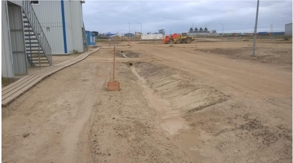
Photo 6 Fly camp drainage channel with new culverts
