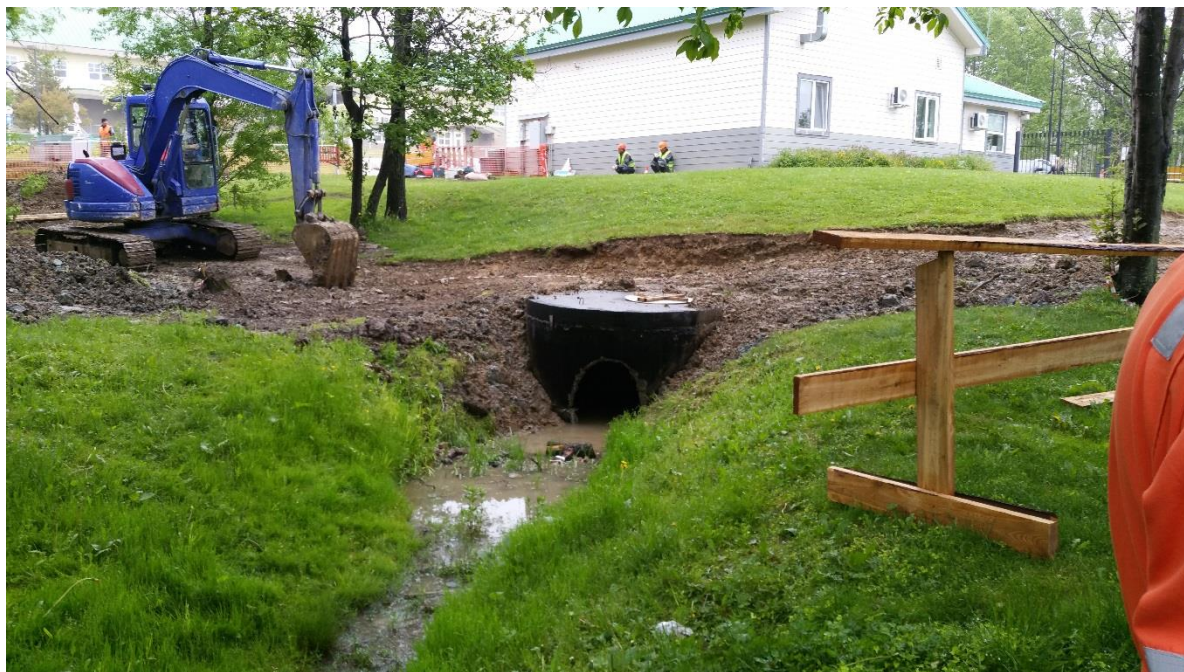
Photo 21 Construction works to redirect the Zima STP discharge to the Pravy brook leading to sediment runoff.
