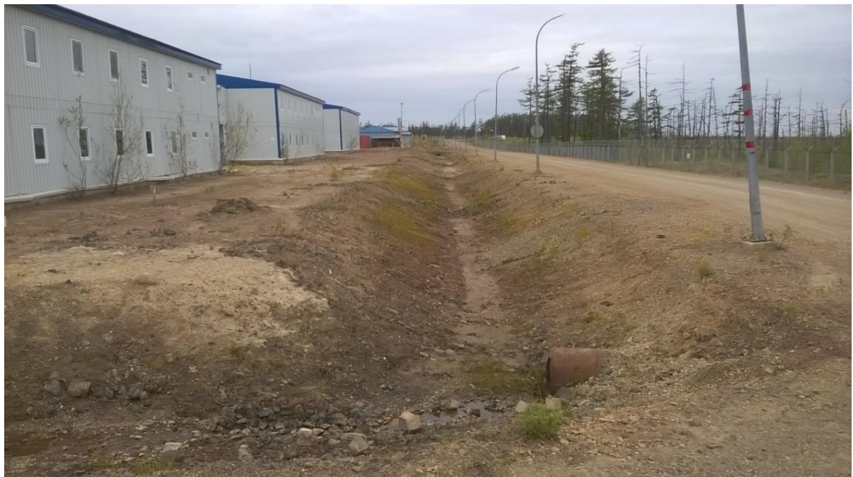
Photo 7 Northeast corner of site where drainage channels join outflow pipe to take water off-site
