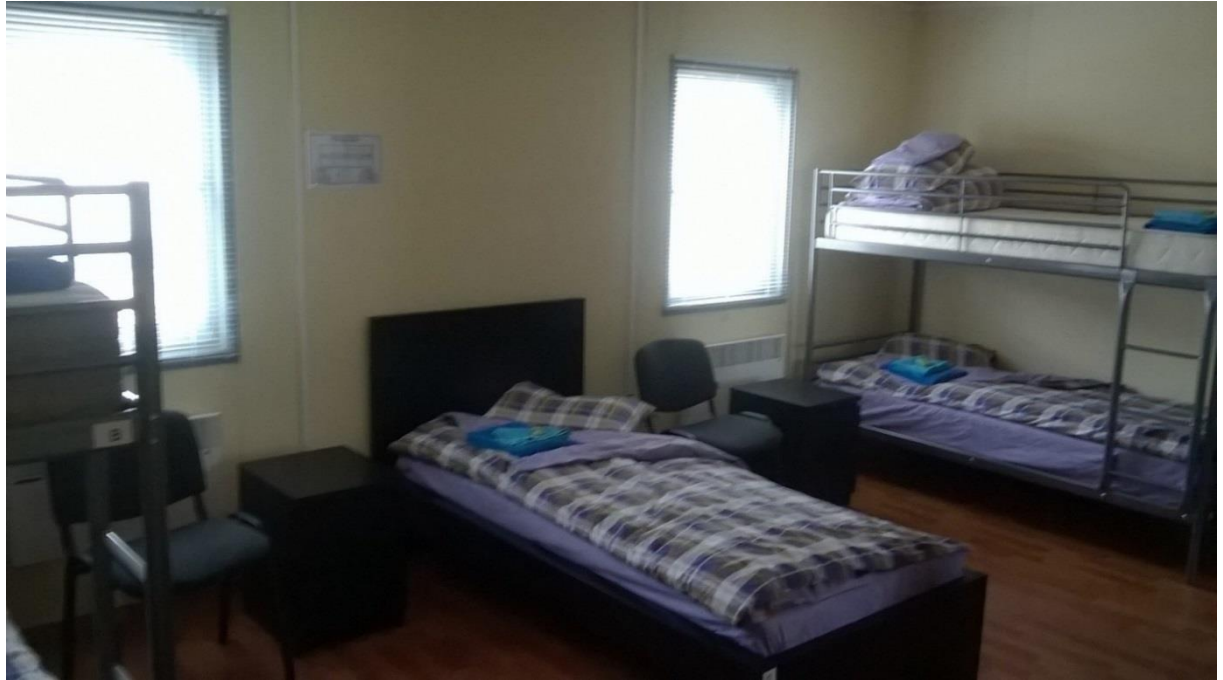
Photo 3 Interior of refurbished accommodation building
