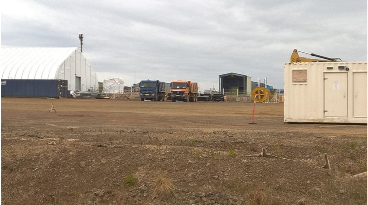
Photo 12 Laydown area. Note drip trays under parked up vehicles
