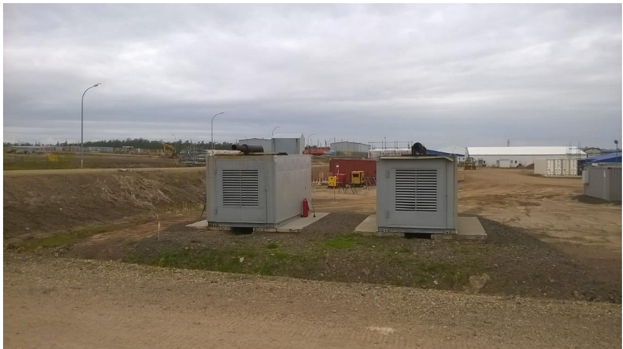
Photo 9 Main camp generators, contained and with measures to prevent ground contamination
