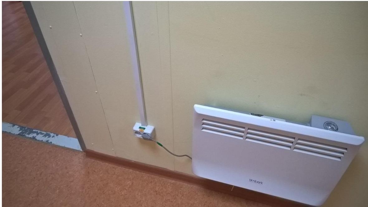
Photo 5 New heating in accommodation. Note electrical colour coding to ensure equipment is tested and up to date
