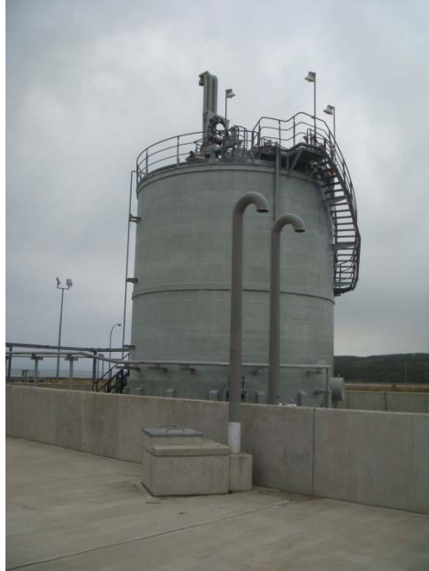
Photo 7: Heat transfer fluid storage
