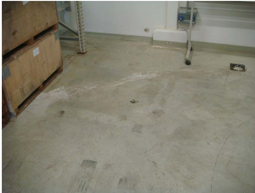
Photo 9: Concrete staining in the alkaline store
