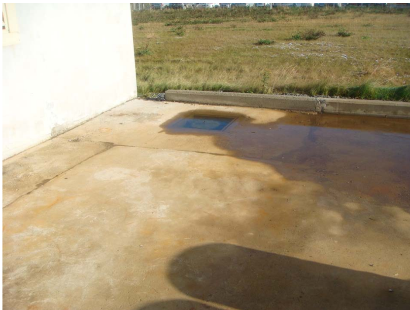
Photo 2: Hole in bund wall around external waste compound
