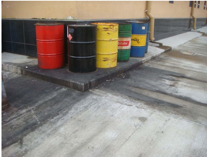
Photo 5: Concrete staining around unlabelled drums containing waste cooking oil
