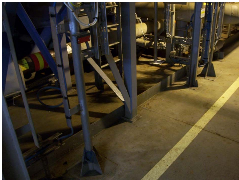
Photo 16: Bunding in design – location is 1st oil separator
