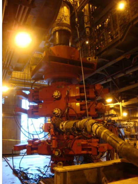
Photo 19: Emergency planning - blow out preventer
