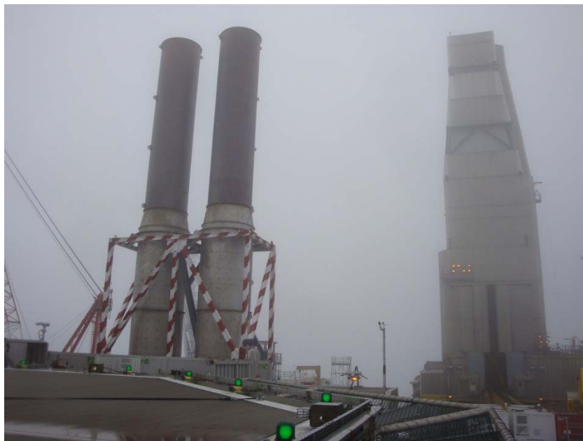
Photo 6: Compressor exhausts in the foreground
