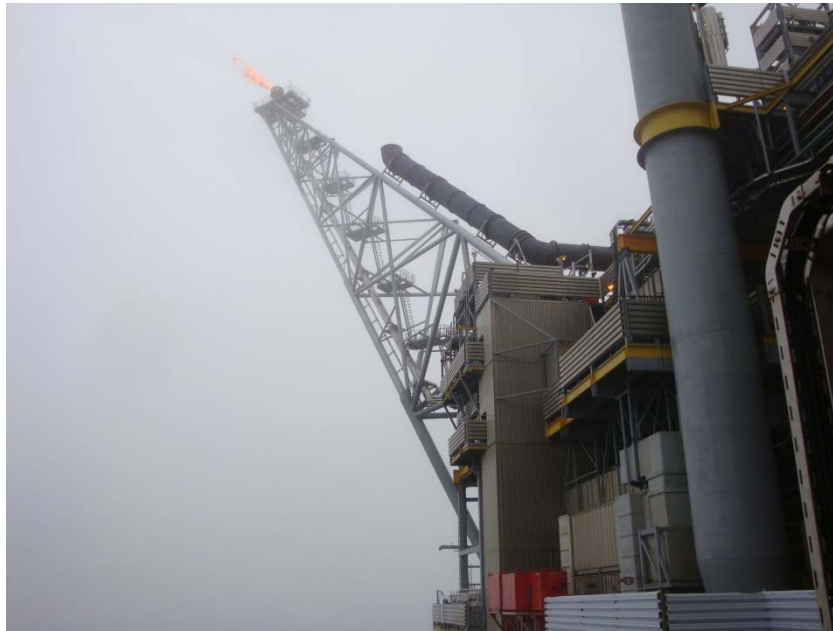
Photo 7: Generator exhaust (attached to flare tower)
