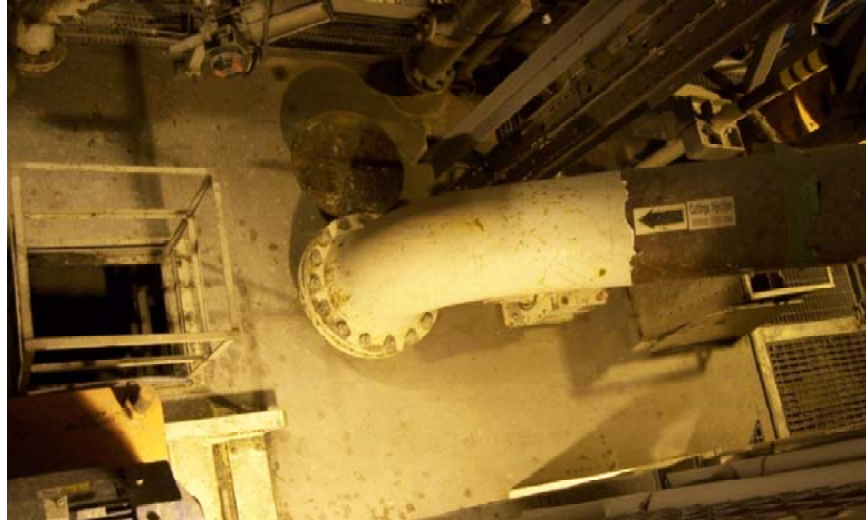
Photo 13: Cuttings reinjection facility (CRI)
