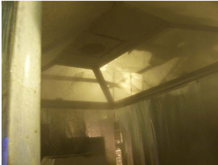
Photo 5: Shale shakers retrofitted with screens and local extraction to reduce dust and aerosols
