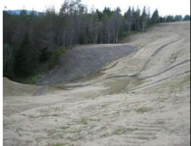
Photo 4 – South slope with soil movement and sparse ground cover
