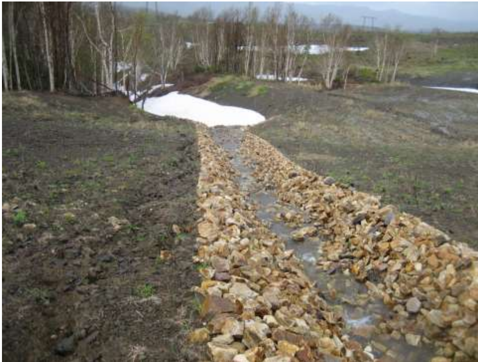
Photo 14 KP 434.9 slope on tributary to the Travyanaya River – use of riprap to line a drainage channel
