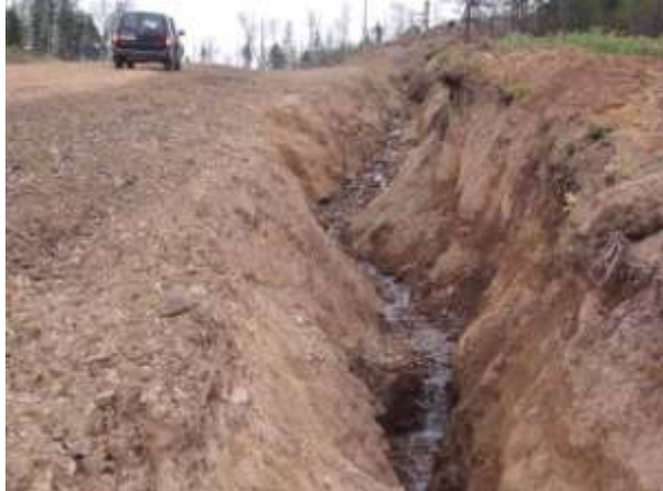
Photo 3 – Access road subsidence
