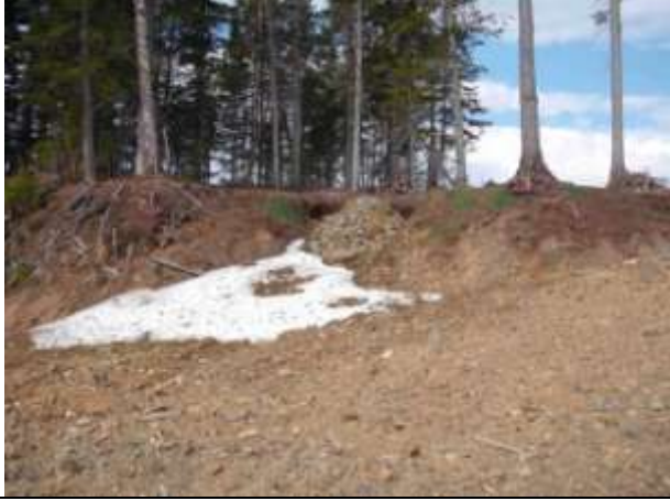
Photo 5 – Undercut tree roots, West bank
