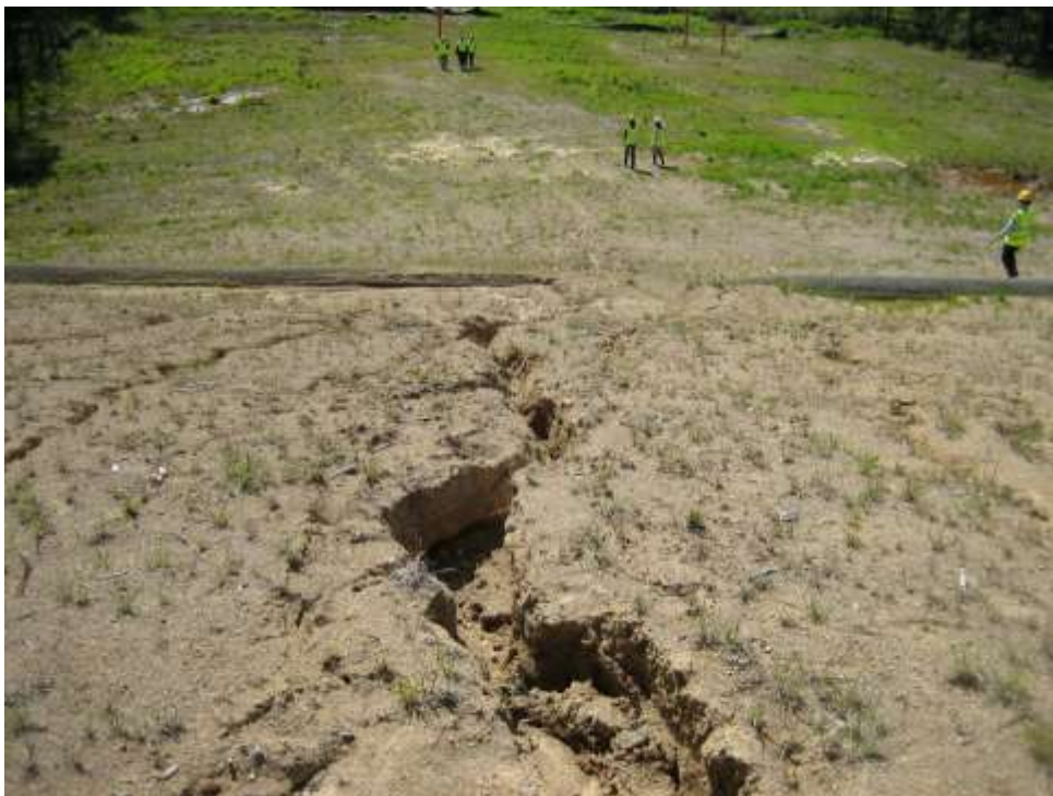
Photo 9 Slope on Korsakov River showing soil erosion between slope breakers
