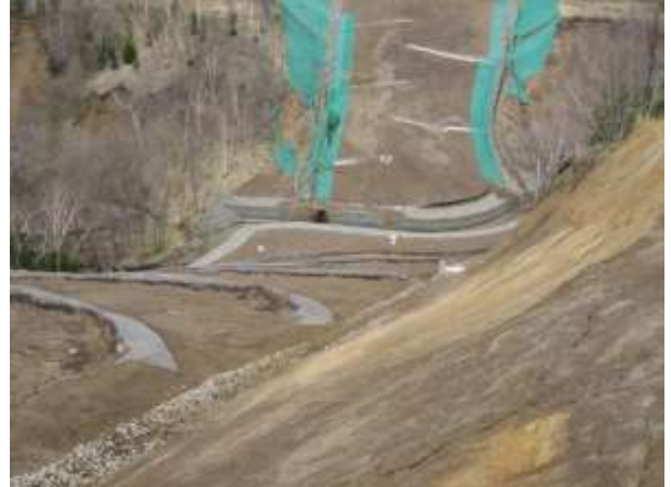
Photo 4 – View of the slopes and gabions on river banks
