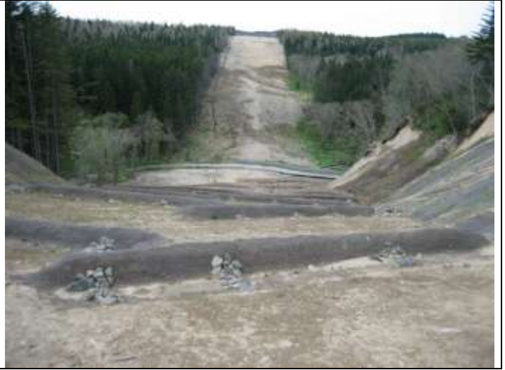
Photo 5 – View of south slope protected with slope breakers but with sparse grass cover. North slope with minimal slope protection and grass cover.
