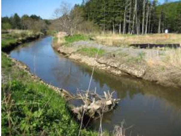
Photo 3 – View to north bank on gas pipe crossing showing Reno mats and some vegetation
