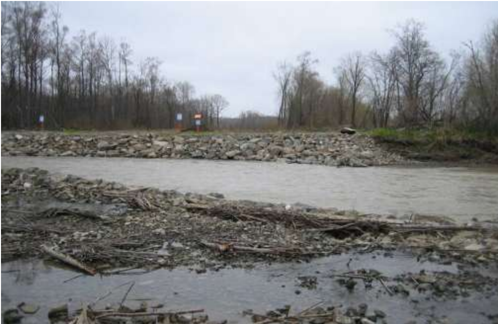
Photo 1 Nitui River - KP 326.6 – View of large riprap on opposite bank
