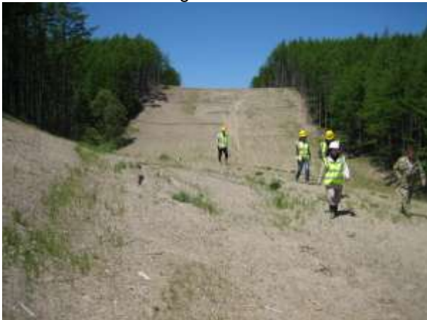
Photo 3 – Showing slopes with drainage control but with little to no vegetation
