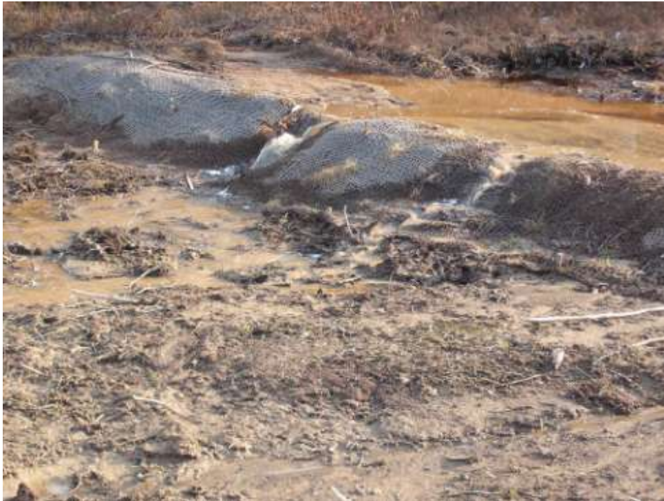
Photo 8 Over-topping of slope breaker near Orkunie River
