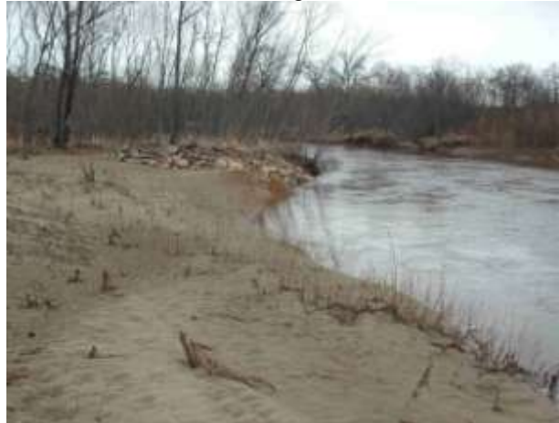
Photo 3 – North bank silting of Reno mats
