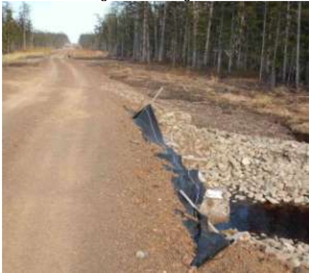
Photo 7 – Damaged silt fencing
