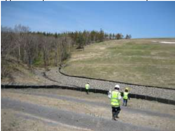
Photo 3 – View south at the RoW with poor bio-restoration and soil movement on the far slope.
