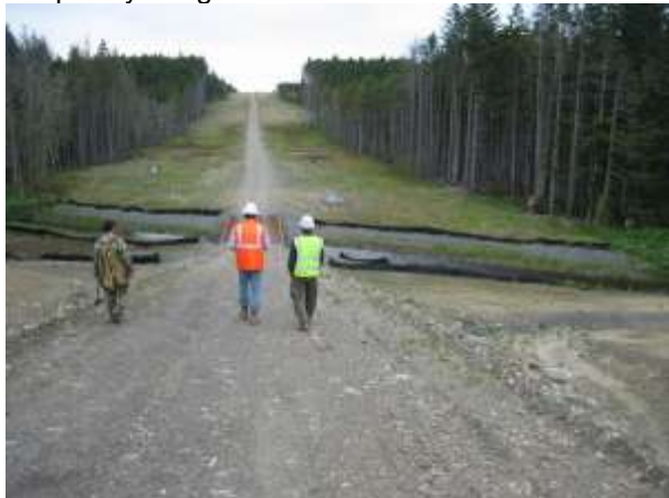
Photo 1 – View north showing river crossing and temporary bridge
