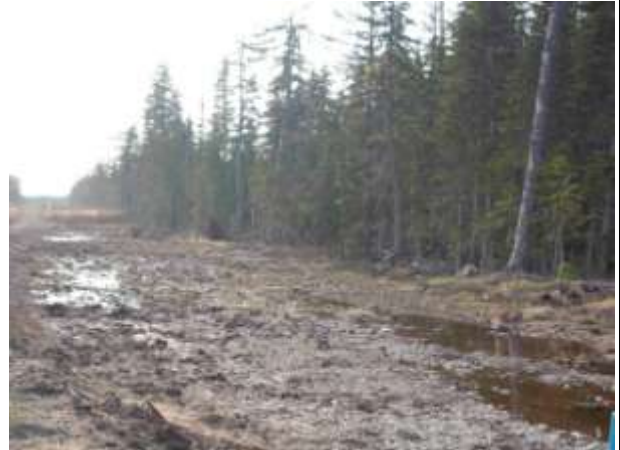
Photo 2 – North road RoW wet
