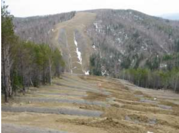
Photo 3 – View of northern slope - slope breakers
