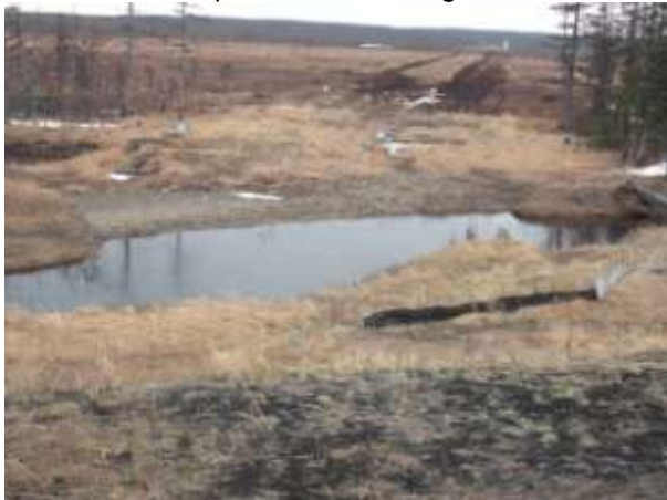
Photo 3 – Silt fencing overwhelmed
