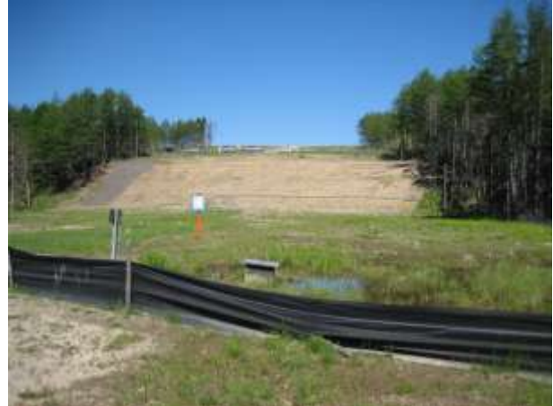
Photo 2 – View to the north showing river valley with good vegetation but slope without vegetation.
