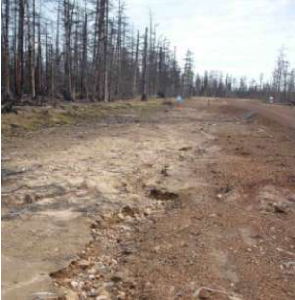
Photo 5 – Blocked drains on access road
