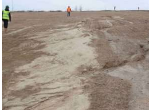
Photo 3 – Erosion runs from east to west across RoW
