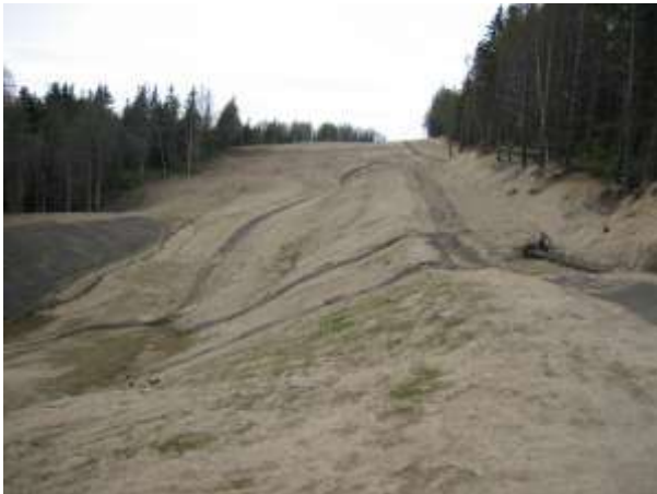
Photo 3 – RoW with sparse ground cover and erosional rills
