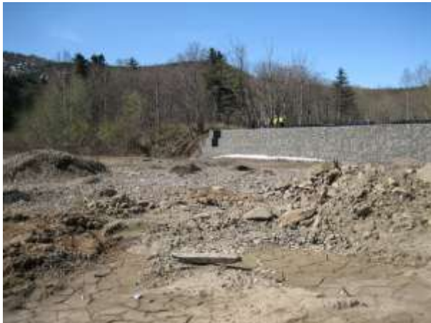
Photo 3 – South bank gabion wall and construction debris
