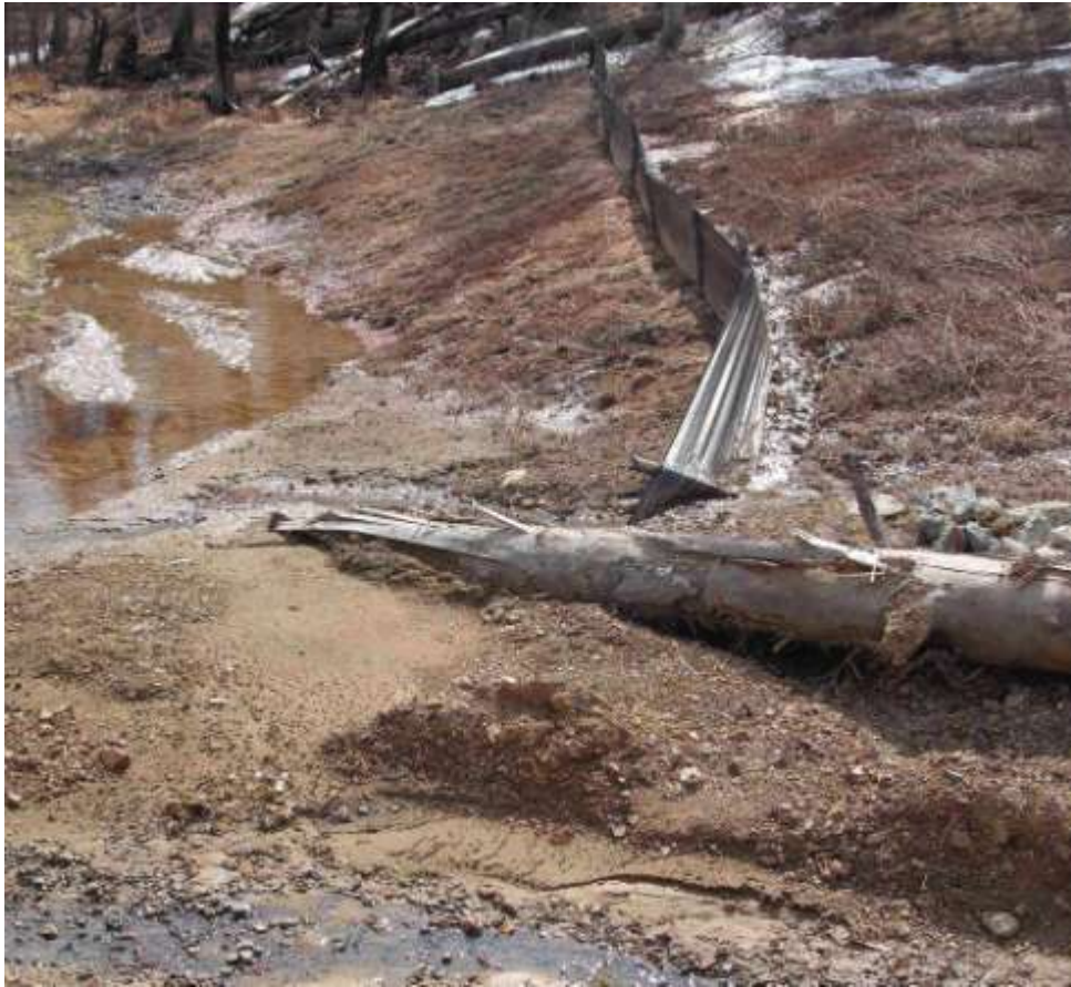
Photo 16 KP15 Failed silt fencing
