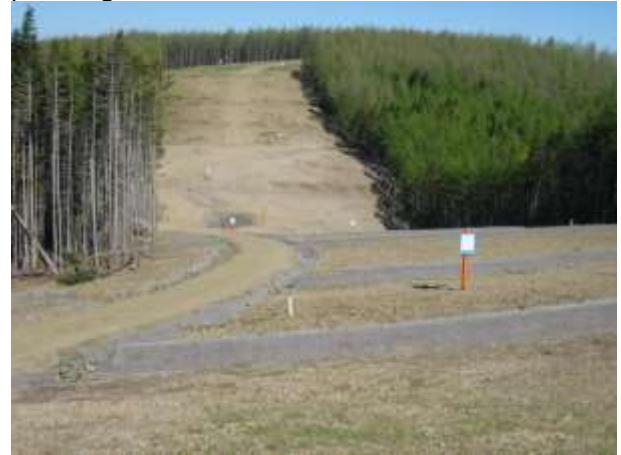
Photo 2 – View of RoW north of the BVS showing poor vegetation cover.
