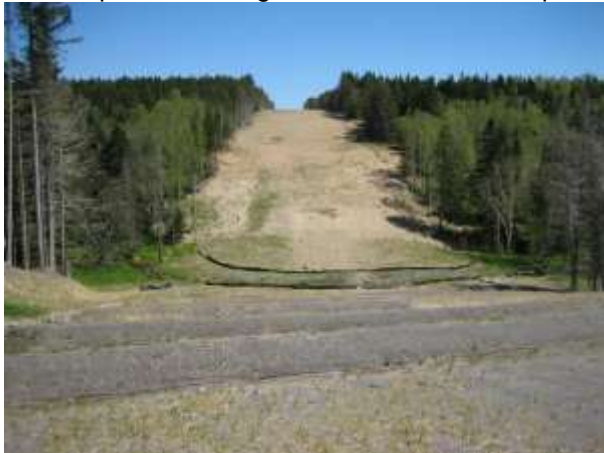
Photo 3 – Slope protection and vegetation on the near slope, lack of vegetation on the north slope
