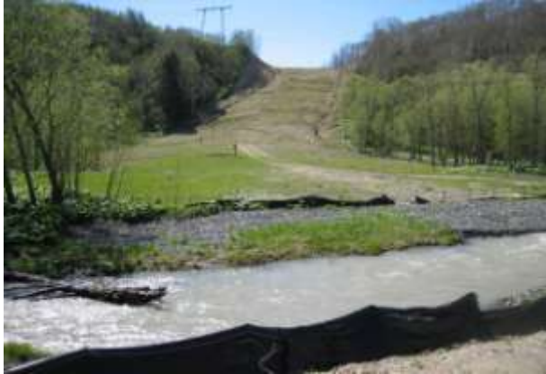
Photo 1 – View of the crossing with Reno mats, and the RoW and south slope with good vegetation.
