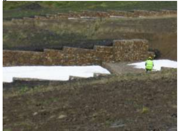
Photo 2 – View of cascading Reno mats and gabion wall construction
