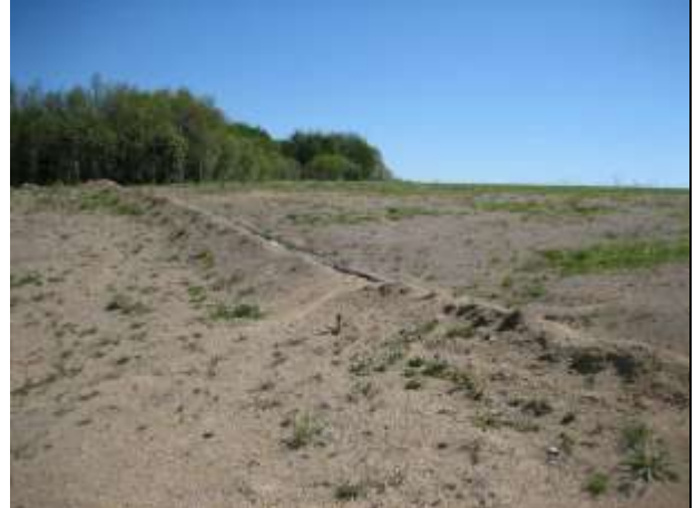
Photo 4 – Slope breaker on the south slope with minimal vegetation.
