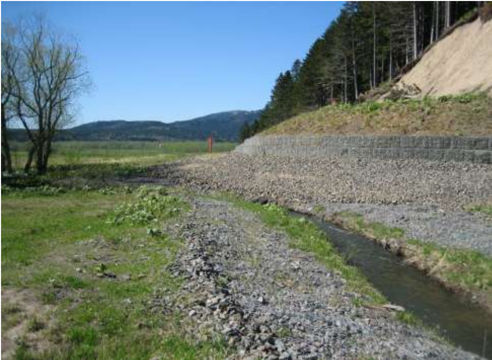
Photo 5 Side cut buttressed by a multi level gabion wall and soil backfill – KP 490.3
