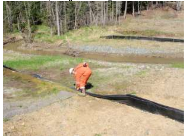
Photo 4 – Repairing silt fencing
