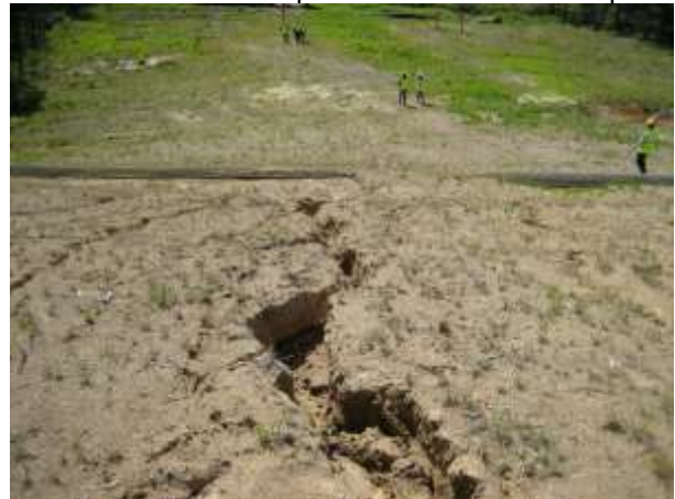
Photo 4 – View of deep erosional rill at mid slope
