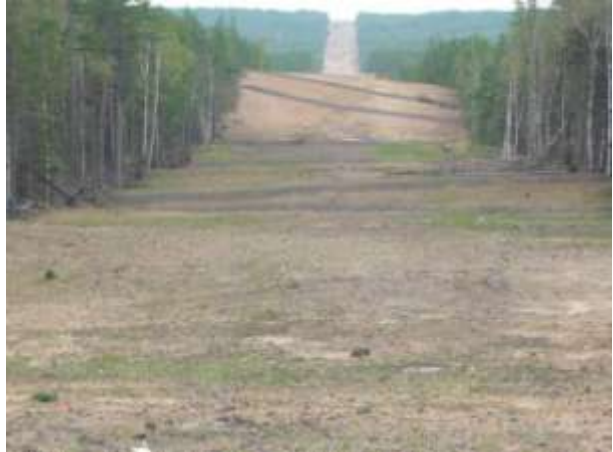
Photo 4 – Silting of slope breaker
