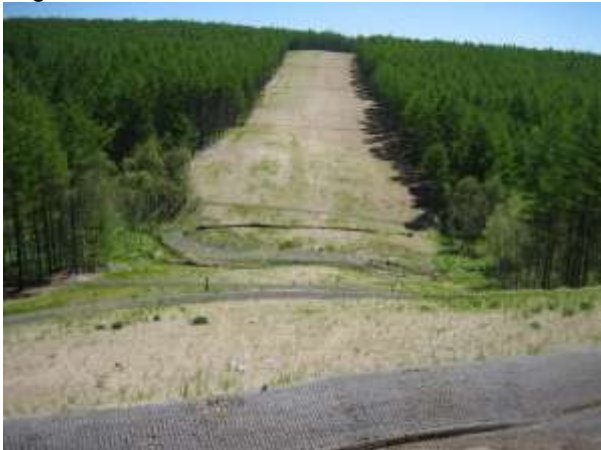
Photo 1 – View south showing river crossing and slopes with slope breakers and very little vegetation
