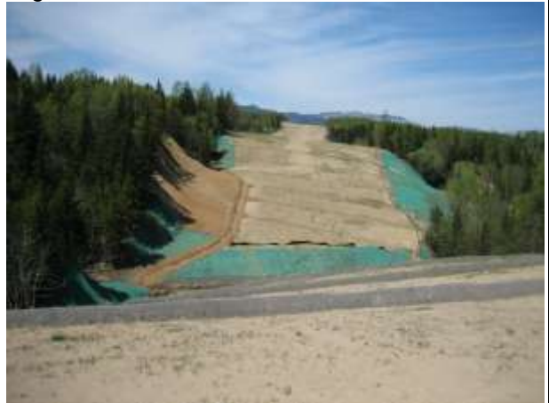
Photo 4 – RoW with erosion control but without vegetation
