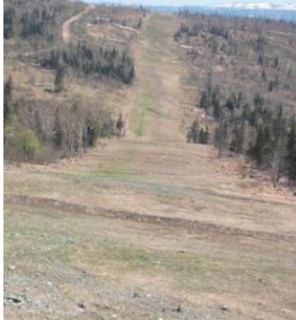
Photo 1 – KP45.5 looking south west
