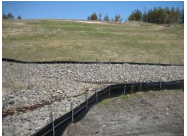
Photo 2 – View of riprap and silt fencing on banks
