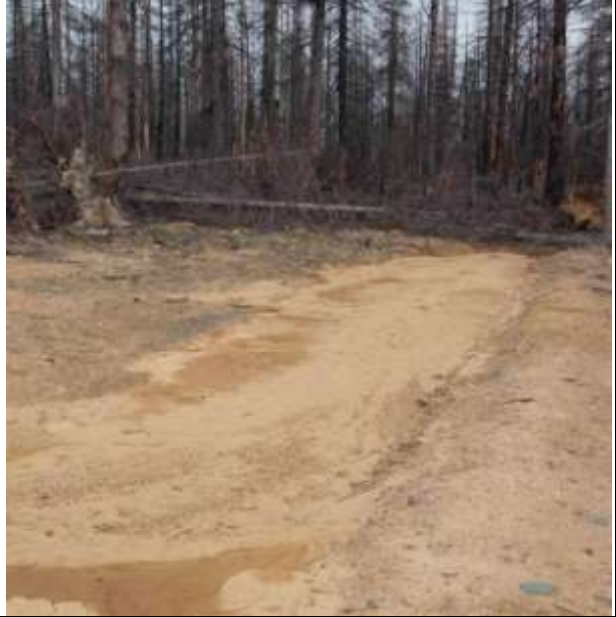
Photo 6 – Damaged silt fencing KP 20
