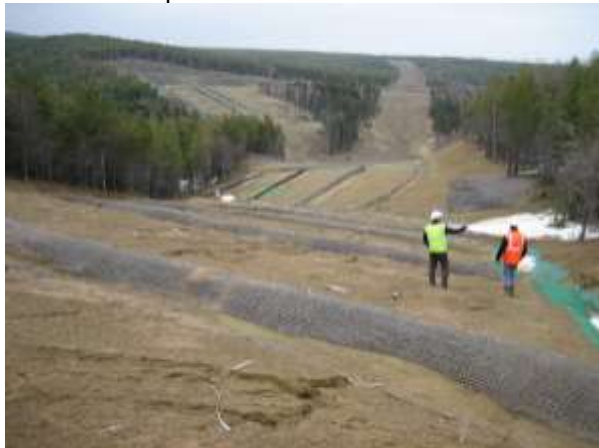
Photo 3 – washout under a slope breaker
