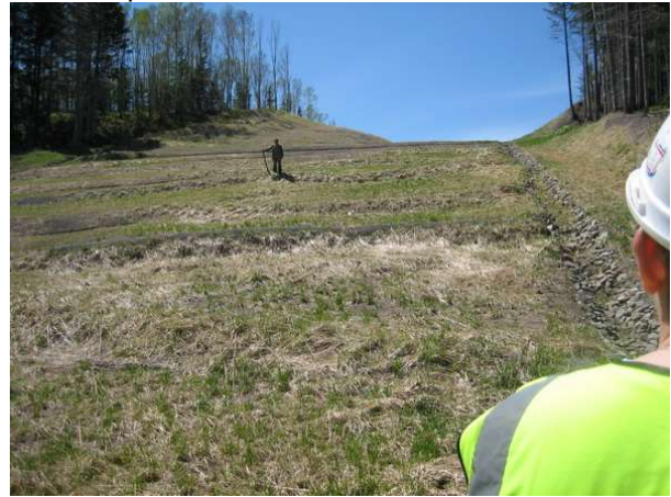
Photo 4 – Slope protection and vegetation on the south slope.
