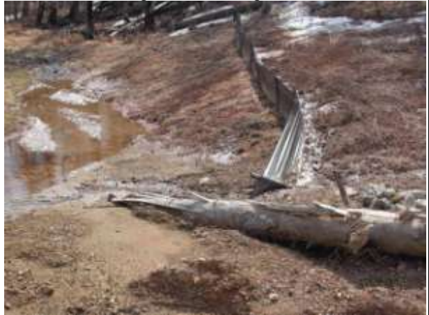
Photo 6 – Damaged silt fencing KP 20
