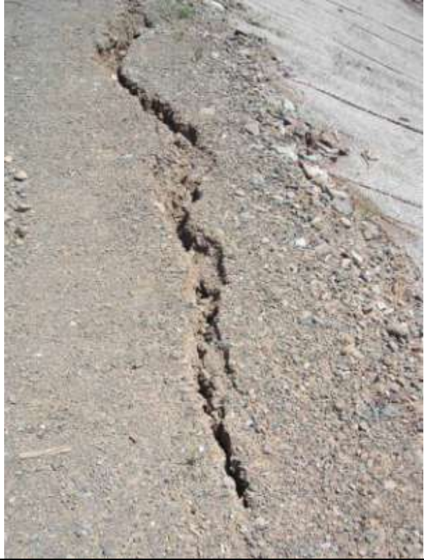
Photo 4 – Tension crack on southern bank
