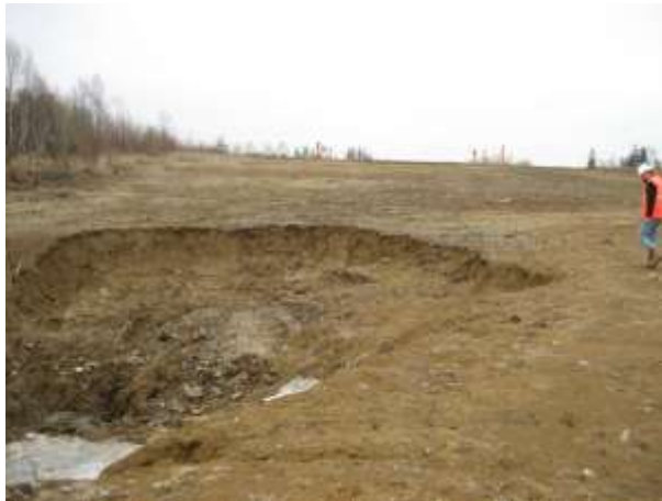
Photo 3 – Wash out at a clean out drain
