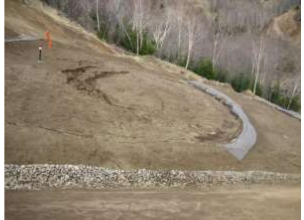
Photo 4 – View of the slopes and gabions on river banks
