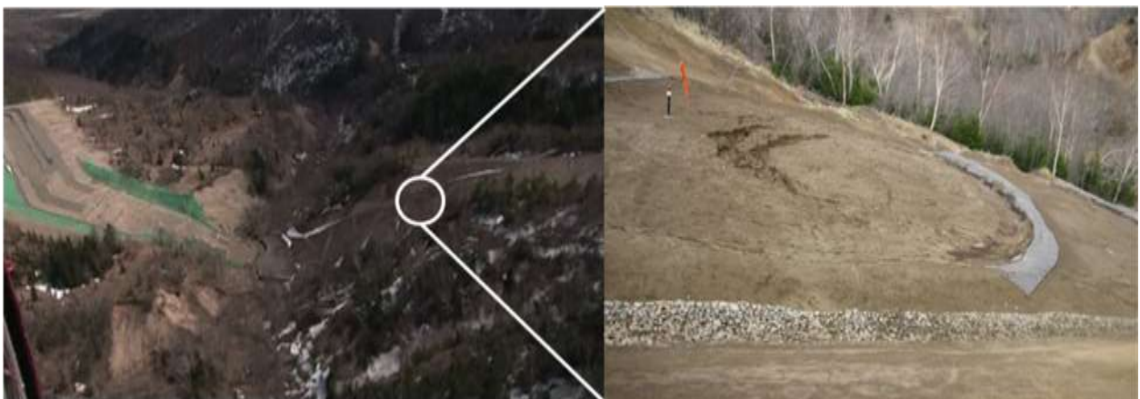
Photo 38 Video still and on-site photo of Khormovaya River Slope failure
