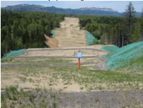
Photo 3 – Lack of vegetation and rill development
