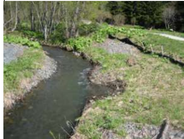
Photo 2 – View to upstream showing bank protection and subsidence on the north bank
