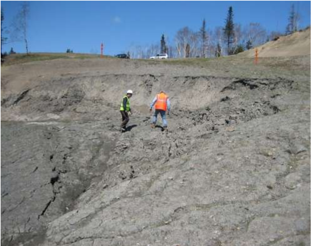
Photo 35 Slope failure at the northern slope leading to the Sedlet River KP 387
