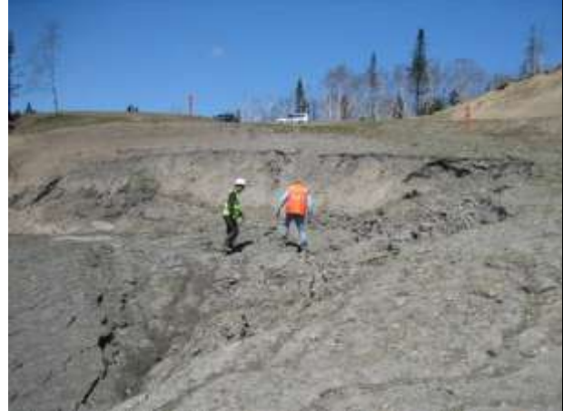
Photo 3 – View at failed ROW slope
