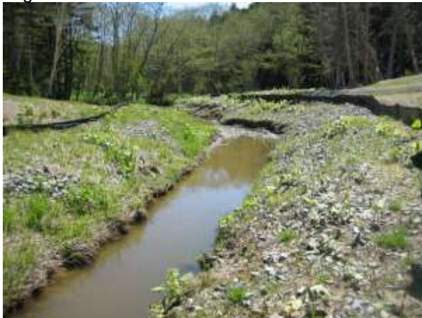
Photo 3 – Slope protection and vegetation on the near slope, lack of vegetation on the north slope
