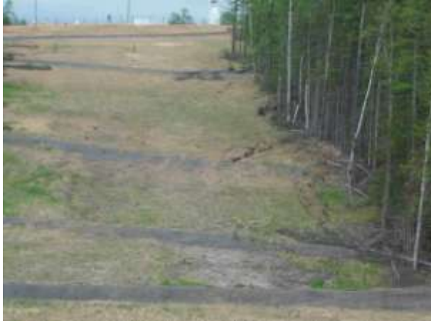
Photo 3 – Erosion rills in barren soil
