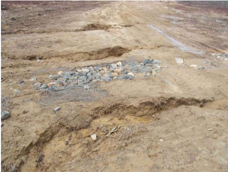
Photo 28 Erosion features in sandy RoW
