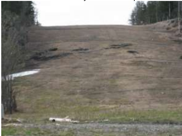
Photo 3 – Soil instability on south slope
