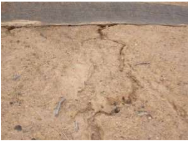
Photo 5 – Scour behind slope breaker
