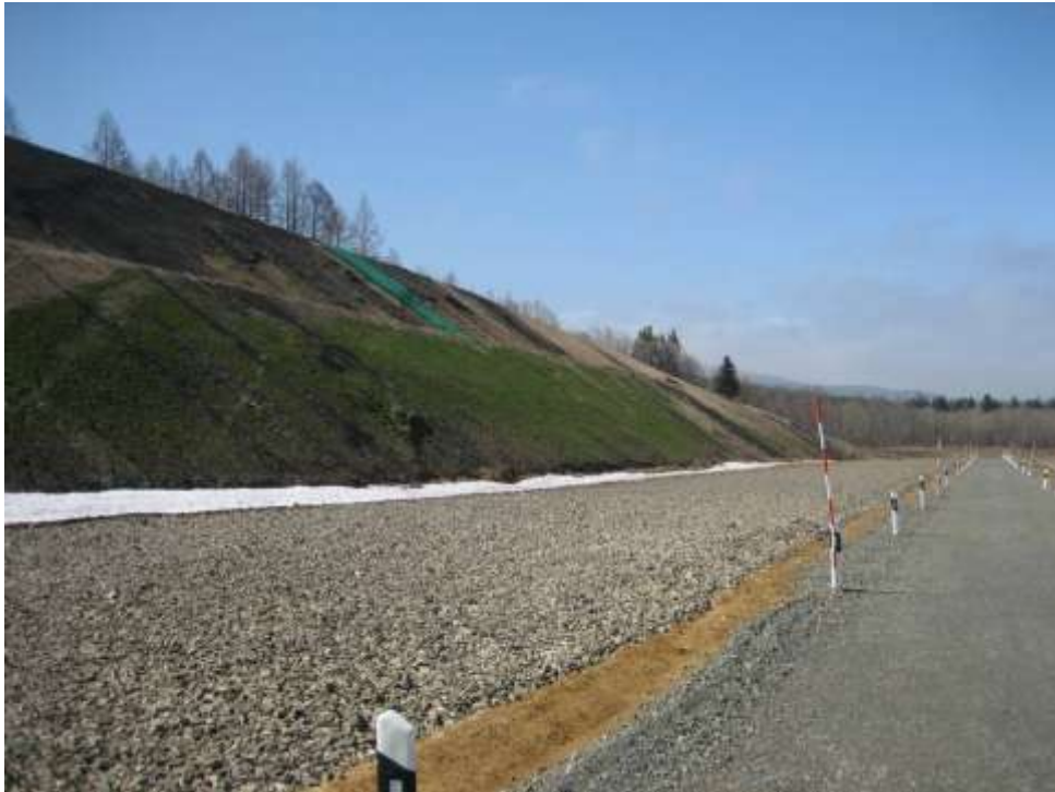
Photo 12 Partially successful use of Geotextile (Enkemat) side cuts at Fault Crossing KP 304
