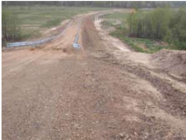
Photo 3 – Access road subsidence
