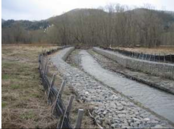
Photo 1 – View of river with gabion walls
