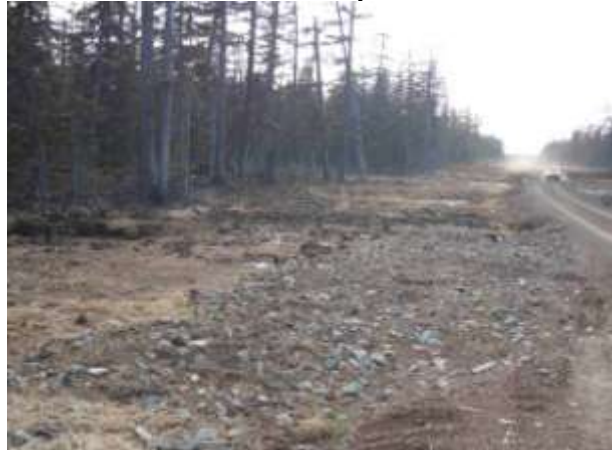
Photo 1 – South road RoW dry
