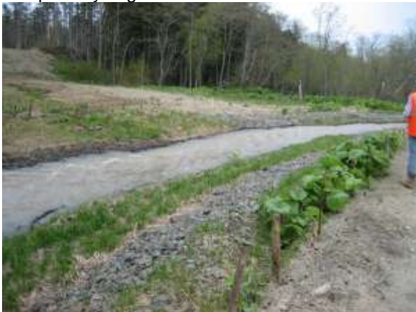
Photo 3 – RoW with sparse ground cover and erosional rills
