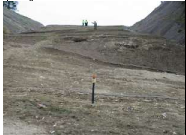
Photo 4 – South slope with soil movement and sparse ground cover
