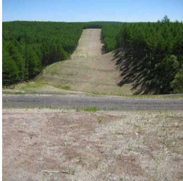
Photo 2 – Showing slopes with drainage control but with little to no vegetation.
