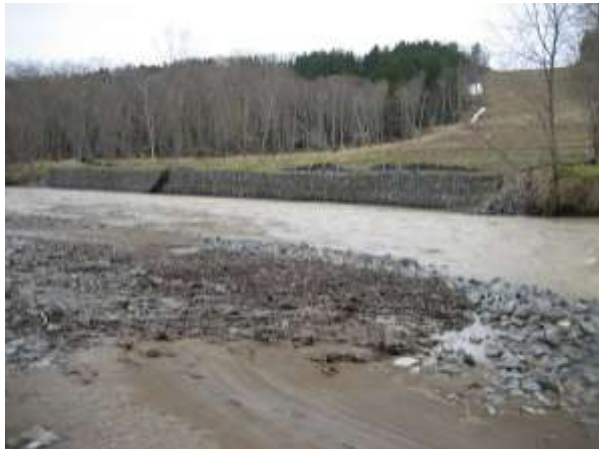
Photo 3 – Gabion wall on the south bank
