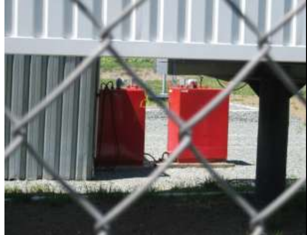
Photo 4 – Diesel day tanks without secondary containment
