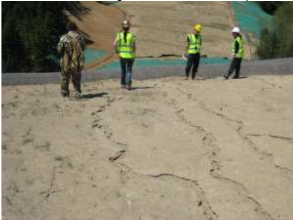
Photo 3 – Lack of vegetation and rill development
