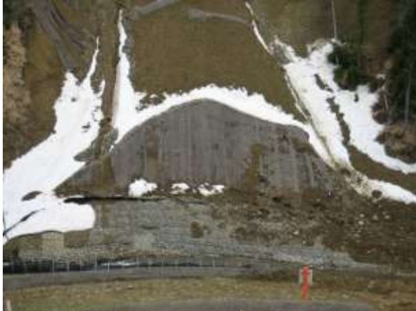
Photo 3 – View of northern slope - slope breakers
