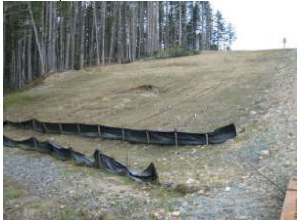
Photo 2 – View of south slope with soil movement at mid slope
