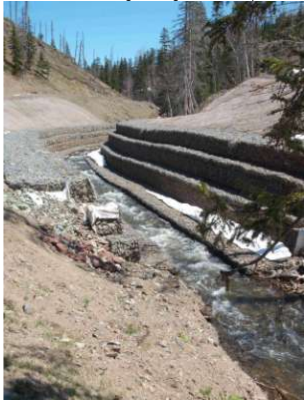
Photo 1 – Gabion engineering at toe of slopes
