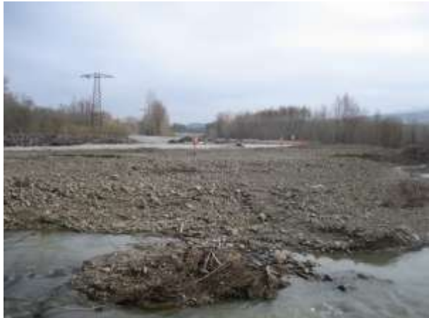
Photo 1 – View to the south bank
