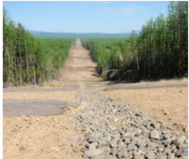
Photo 30 Sandy slopes 2010 – coco matting on slopes gone and seed stock not in evidence, no shoots showing
