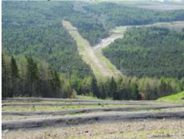
Photo 1 – View south at the Mereya slope and the ROW splitting in two at approach to LNG plant.
