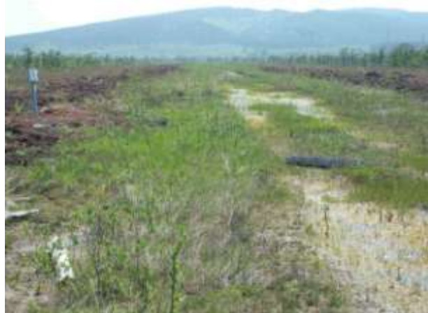
Photo 3 – Twin mounds over the pipelines
