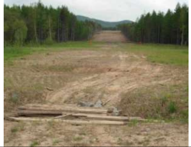
Photo 5 – Unauthorised access onto RoW
