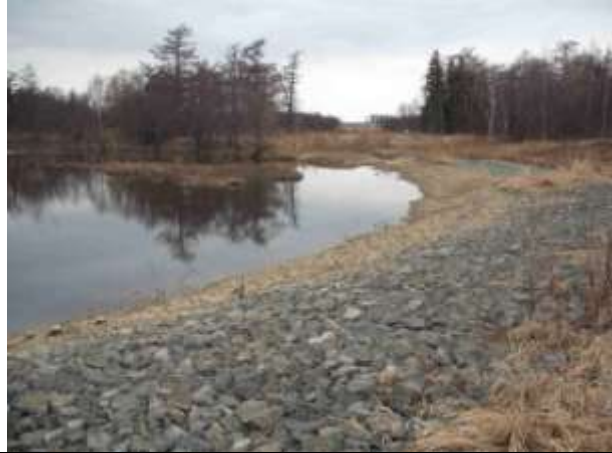
Photo 3 – North bank silting of Reno mats
