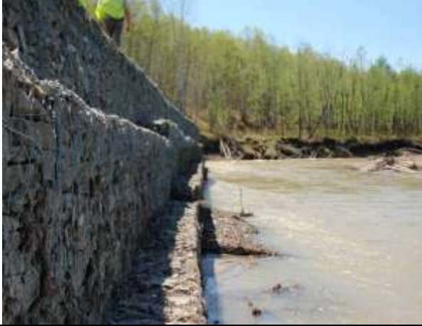
Photo 5 – River undercutting outer bank
