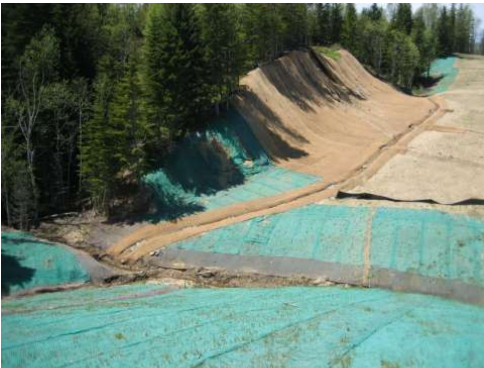
Photo 11 Geojute and Geotextile (Enkemat) on the sandy slopes KP 512
