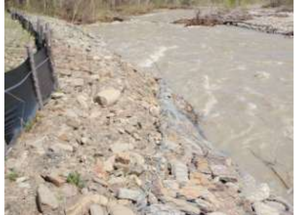
Photo 2 – Reno mats require maintenance
