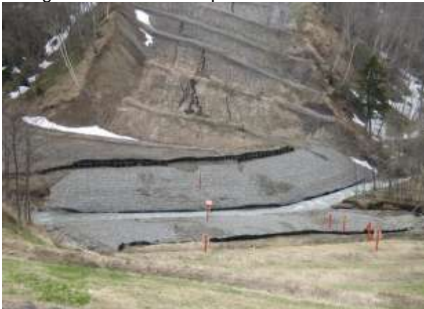
Photo 3 – View to the south at the long south slope with slope breakers
