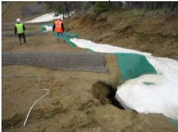
Photo 3 – washout under a slope breaker
