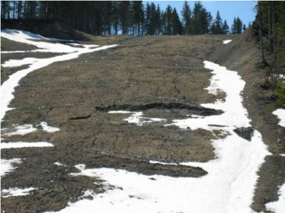
Photo 36 A start of a failure on the southern slope of the Lesnaya 3 River KP 380.6
