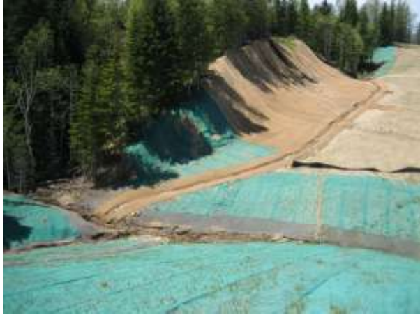
Photo 5 – Heavily protected crossing drainage, including slope breakers and geotextile
