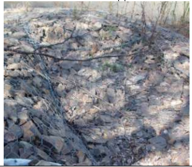
Photo 5 – Subsidence over the pipeline
