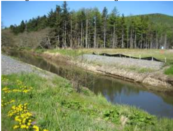
Photo 3 – View to north bank on gas pipe crossing showing Reno mats and some vegetation
