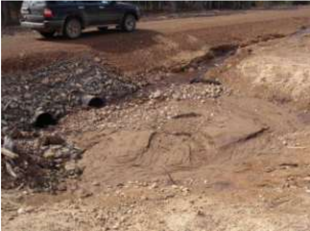
Photo 5 – Blocked drains on access road
