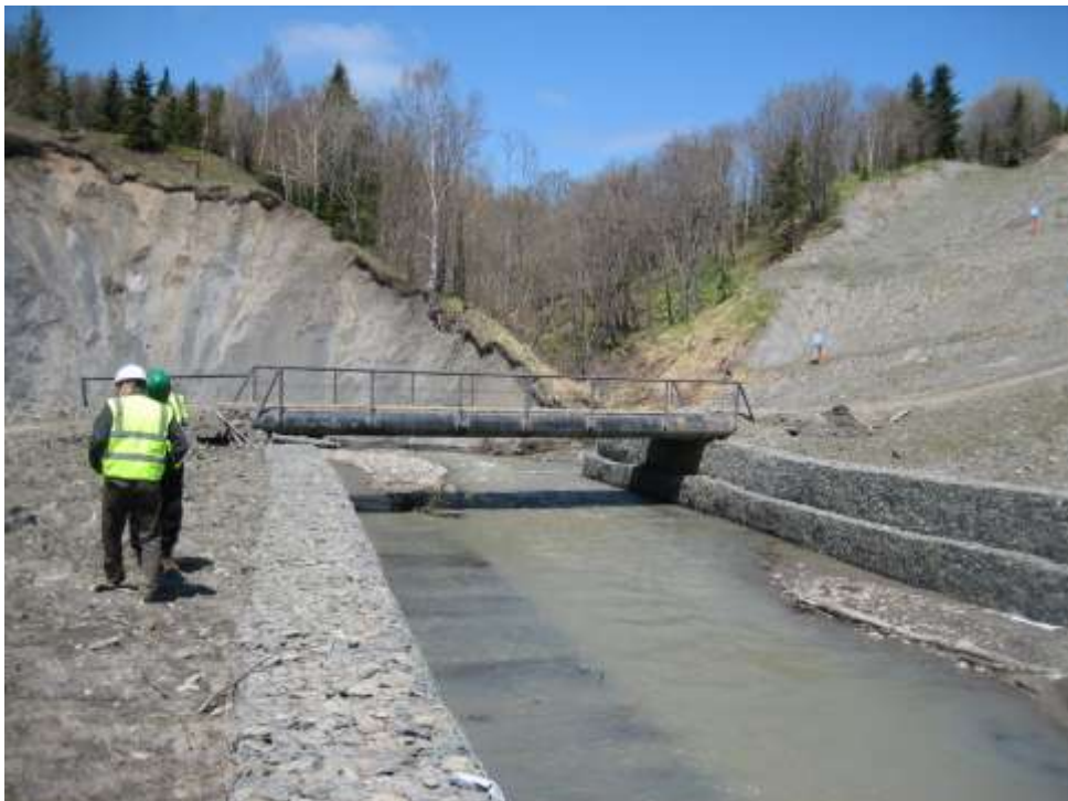
Photo 4 View of gabion walls on the banks of the Lazovaya 2 River crossing – KP 384.5
