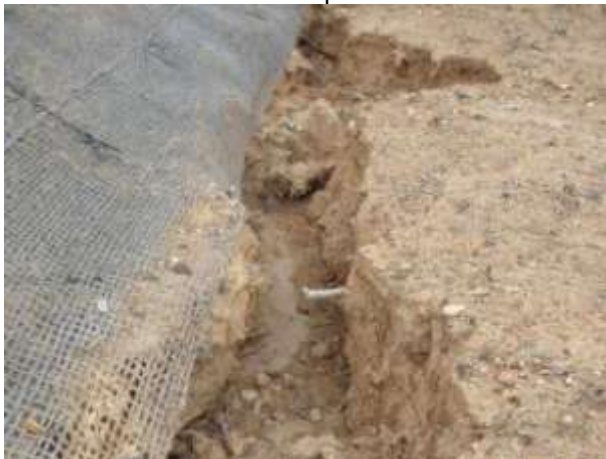
Photo 5 – Scour behind slope breaker
