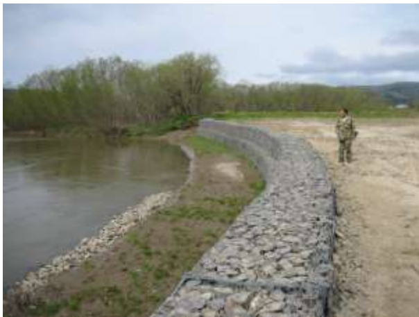
Photo 3 – View of the south bank upstream of the crossing with temporary fortified bank
