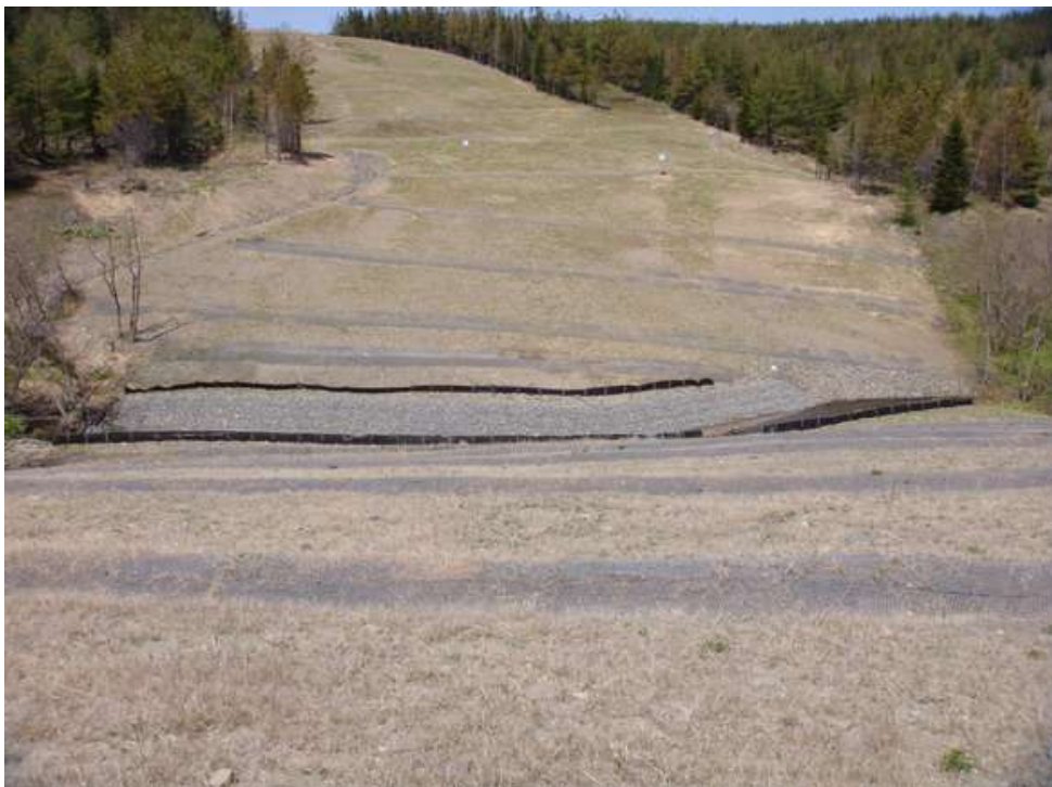
Photo 7 Well constructed slope breakers on the Vulkanka River Slopes
