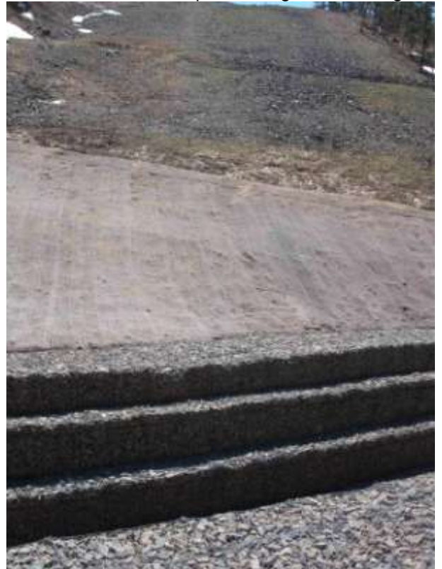
Photo 2 – Northern slope showing coco matting
