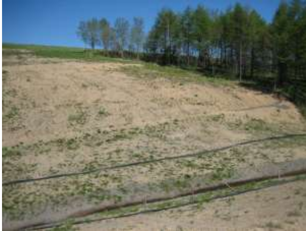
Photo 3 – View of a crossing drainage protected with geo-jute and slope breakers. However, poor grass cover.
