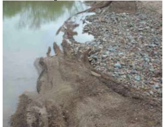
Photo 4 – Damaged bund on north bank
