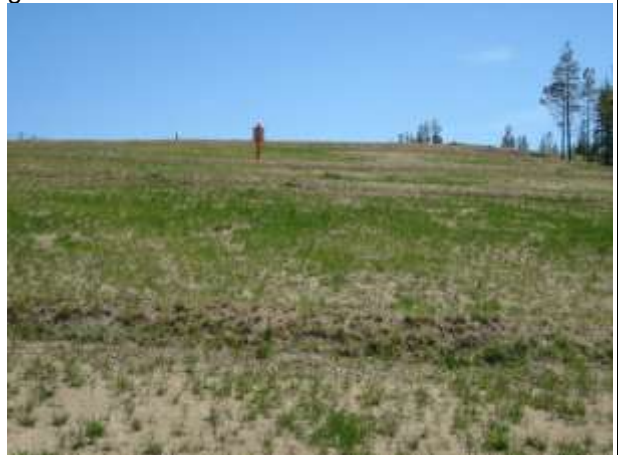
Photo 4 – RoW with erosion control but without vegetation
