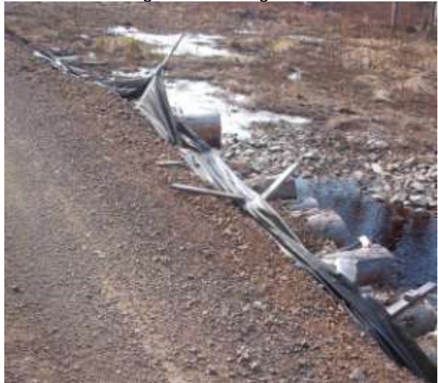
Photo 8 – Damaged silt fencing
