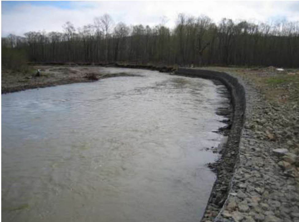
Photo 3 View of gabion wall on the Madera River - KP 373
