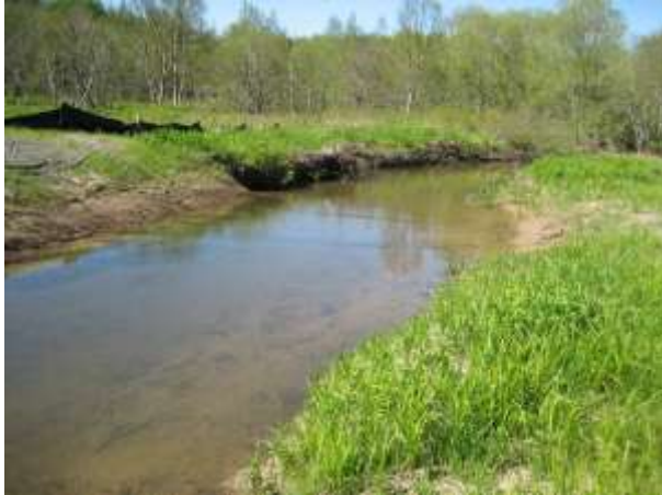
Photo 3 – View of erosional rill development between slope breakers and lack of grass cover.
