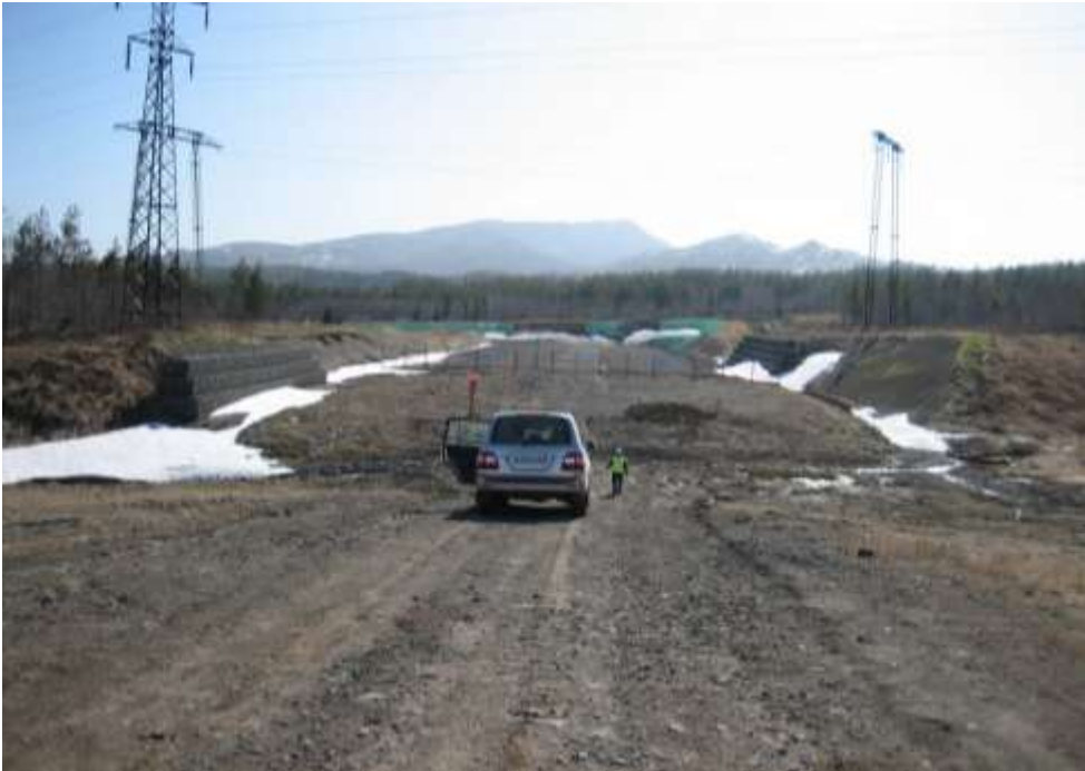
Photo 6 Side cut buttressed by a multi level gabion wall and soil backfill – KP 304
