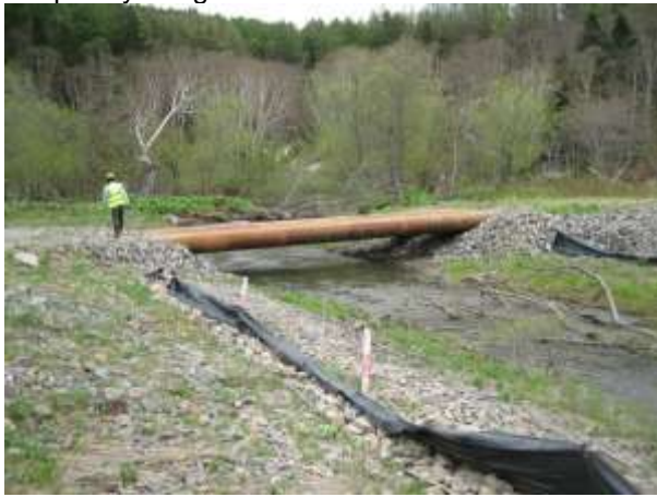
Photo 1 – View of river bank with Reno mats and temporary bridge
