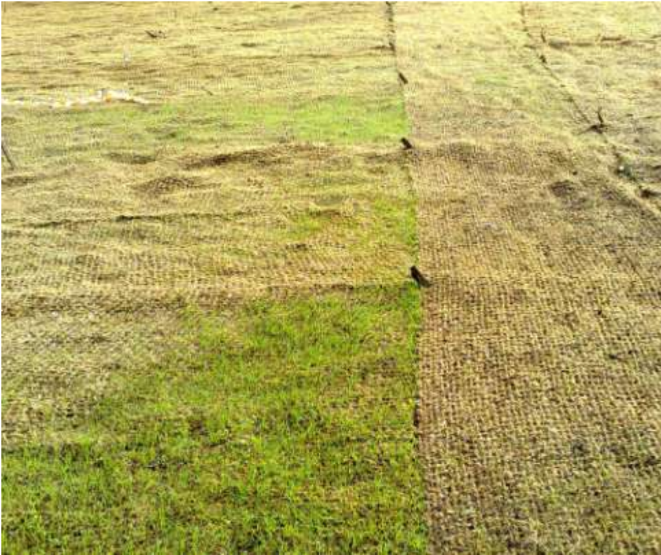
Photo 10 Geo-jute and seeding (2008) – sandy slopes KP125
