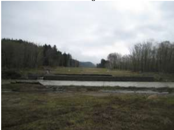
Photo 1 – View to north of gabion wall and RoW
