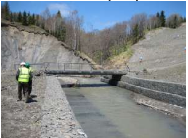
Photo 2 – Downstream – bridge and gabion walls
