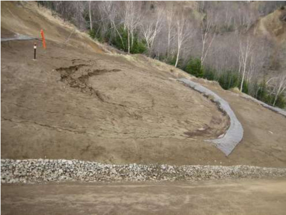
Photo 37 A start of failure at the southern slope of Kormovaya River – KP 351
