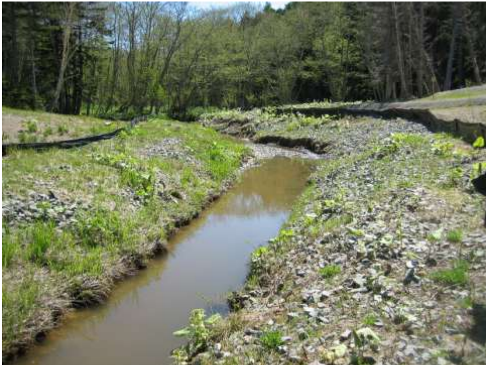
Photo 15 KP 510.4 Silt fence on the Podgorodnaya River
