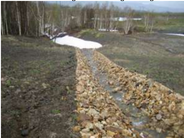
Photo 3 – Armouring of a crossing drainage
