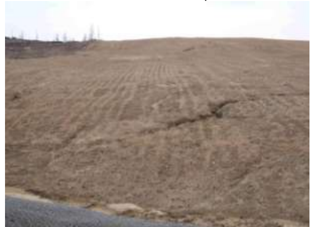
Photo 4 – Silt run-off from the RoW
