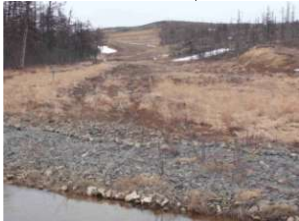
Photo 3 – Washout behind Slope Breaker
