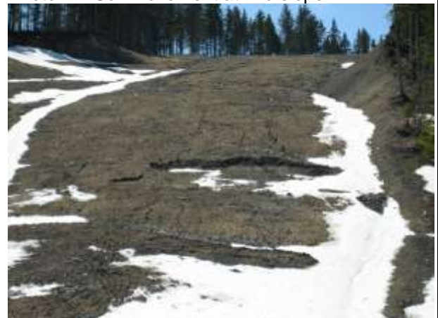
Photo 4 – Soil movement at mid slope
