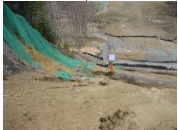
Photo 4 – Erosion of slope above the river
