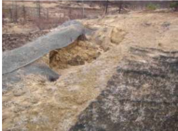
Photo 3 – Washout behind Slope Breaker
