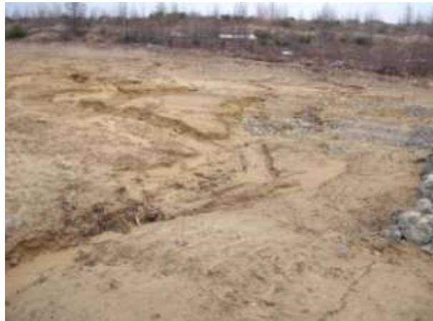
Photo 3 – Erosion runs from east to west across RoW
