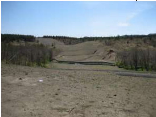
Photo 3 – View south at the RoW with poor bio-restoration and soil movement on the far slope.
