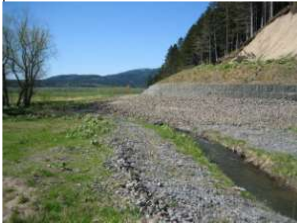
Photo 1 – View to downstream showing bank protection
