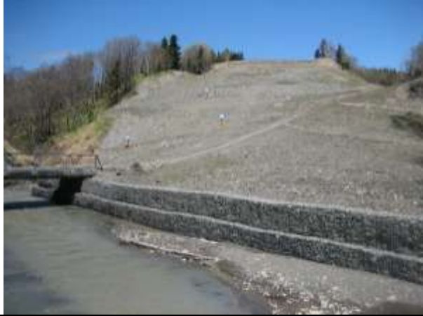
Photo 3 – Downstream – bridge and gabion walls
