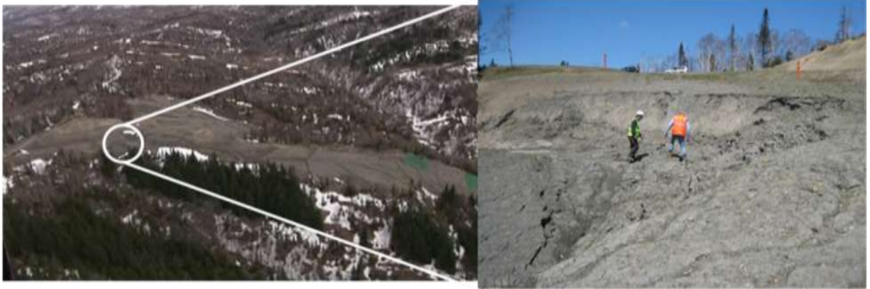
Photo 39 Video still and on-site photo of Sedlet River Slope failure
