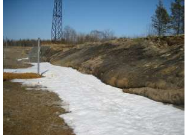
Photo 4 – Failed site cut
