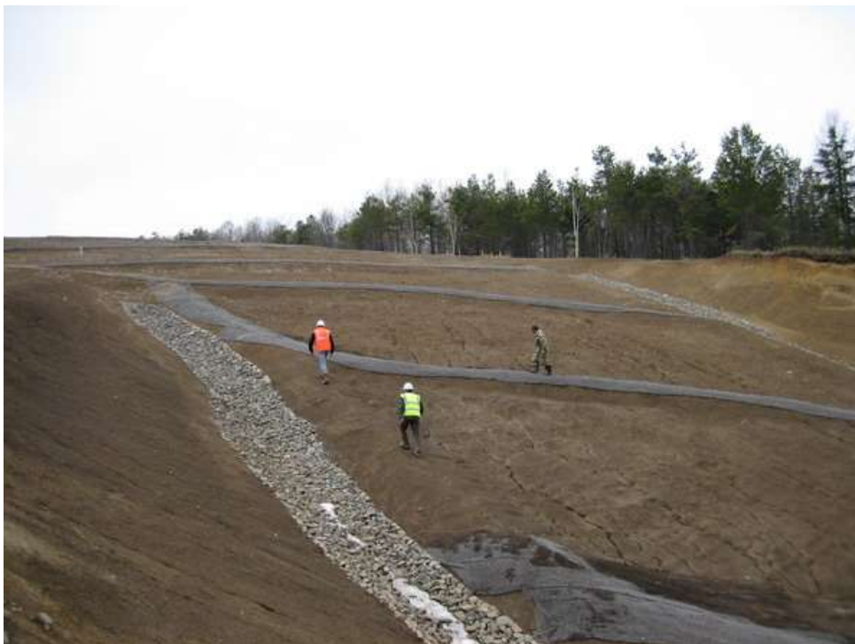
Photo 34 Heavy duty engineering works but lack of vegetation, Khormovaya River
