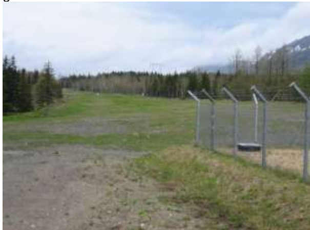
Photo 1 – View north showing RoW with good grass cover.
