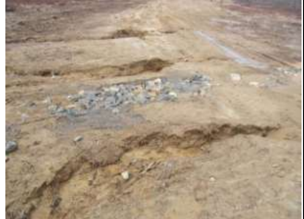
Photo 4 – Silt and sand run-off away from the RoW
