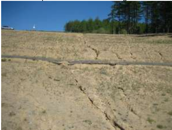
Photo 3 – View of erosional rill development between slope breakers and lack of grass cover.
