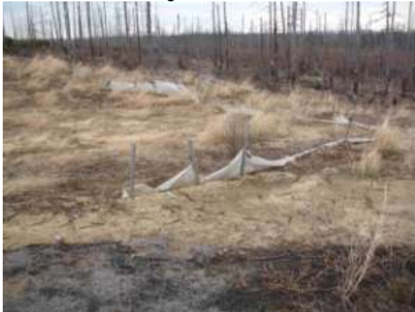
Photo 3 – Silt fencing overwhelmed
