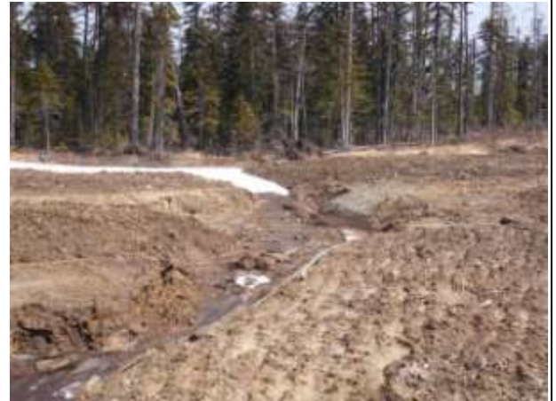
Photo 2 – Formation of erosion rills
