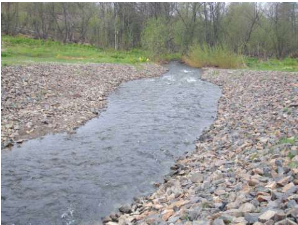
Photo 13 KP56 Svetye Stream Riprap
