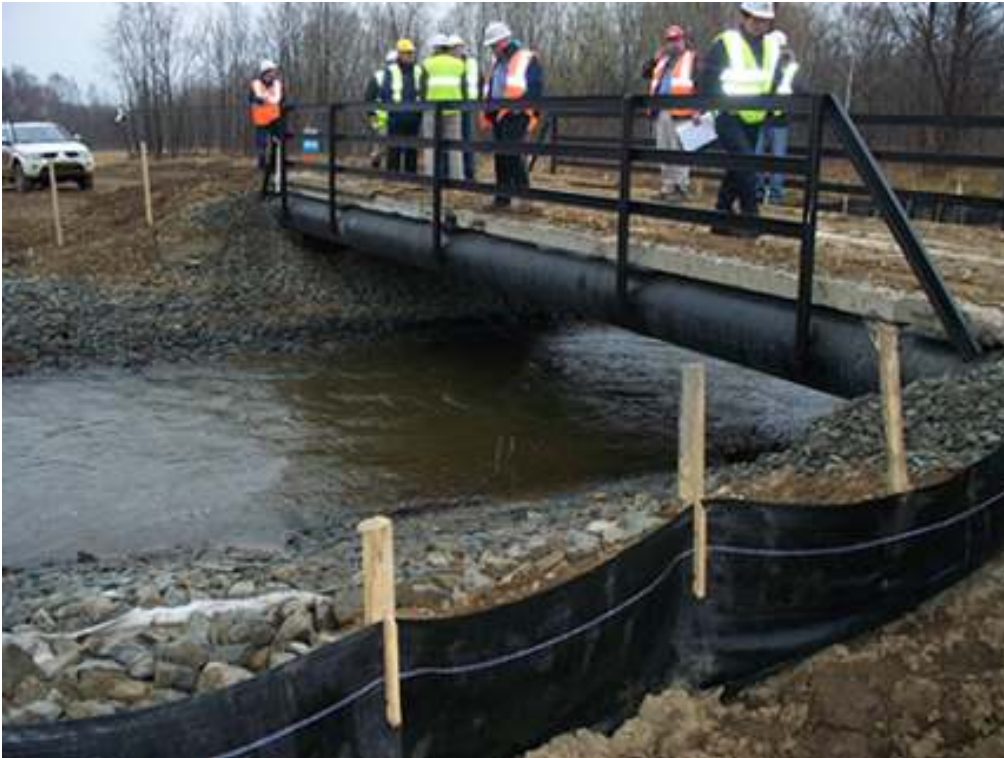
Photo 15 KP 314 Mana – Newly installed permanent bridge. Silt fence should be installed and tied into bridge until freshly disturbed soil is allowed to stabilise. Similar works remain on approximately 60 bridge sites.
