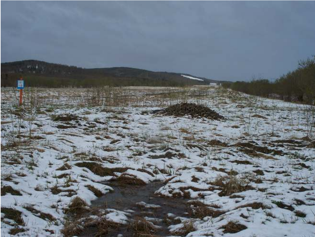
Photo 16 KP 510 Wetlands reinstatement with promising regeneration. Slight crowns over pipelines are not a current problem but will require monitoring, as noted by Sakhalin Energy.
