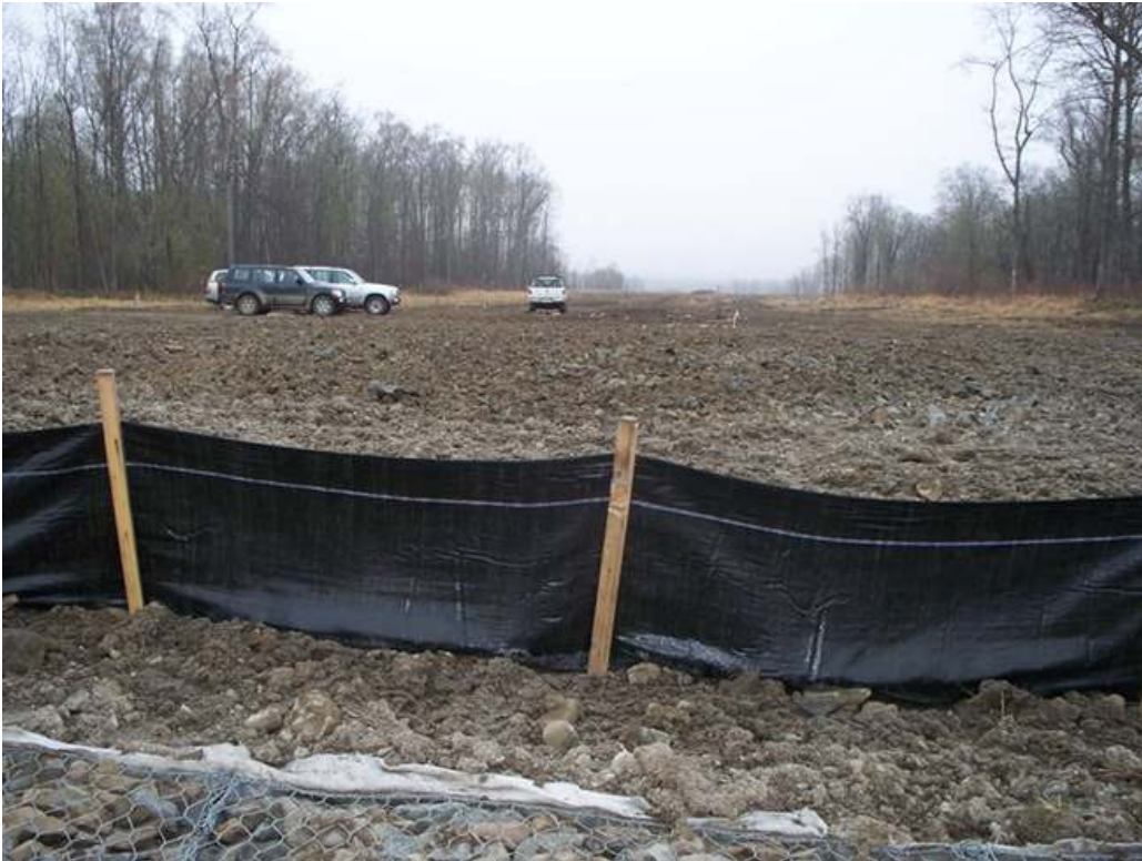
Photo 22 Technical reinstatement not complete (temporary access road still in) and biological reinstatement not complete at KP 313 Goryanka. Scheduled to be competed summer 2009.
