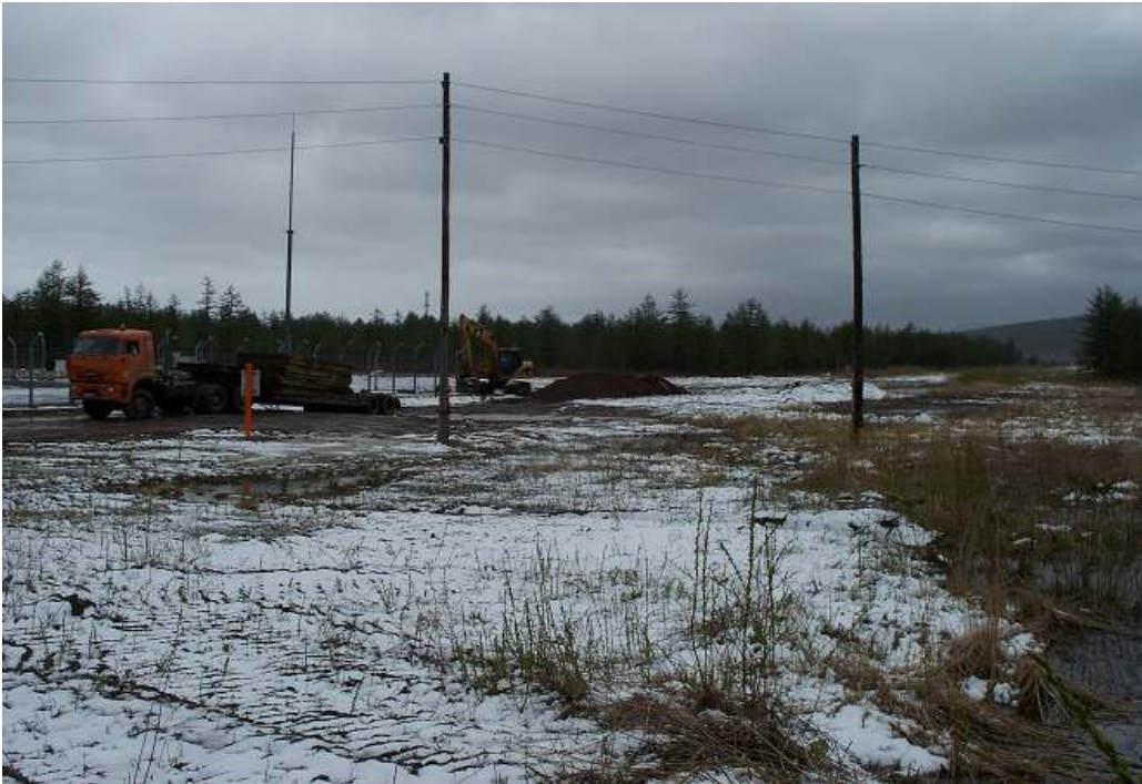
Photo 20 Operations at KP 524 (edge of Dolinsk wetlands) to correct subsidence over pipe shows active monitoring and maintenance of RoW. Bog mats used to minimize damage to wetland habitat and peat used as fill to avoid placement of foreign material in wetlands – both good practice.
