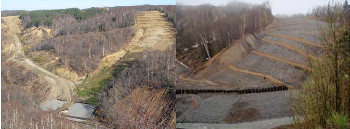
Photo 19 Comparison of KP 348 Krinka from September 2008 to May 2009 showing erosion control measures effective after spring thaw. Area will require ongoing monitoring.
