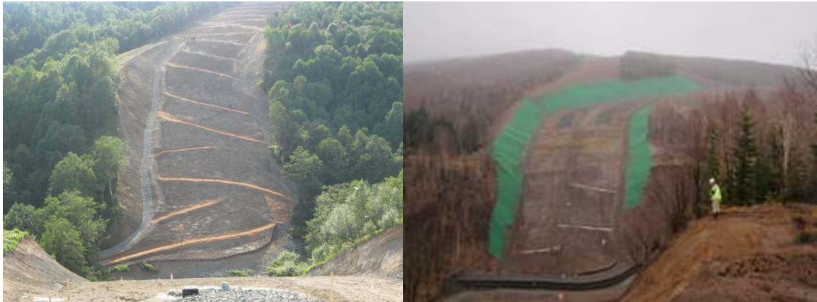
Photo 18 Comparison of KP 347 Kormovaya from September 2008 to May 2009 showing additional engineering (new slope breakers, dual side drainage channels, geotextile fabric on side cuts).
