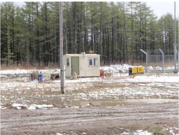
Photo 23 Insufficient secondary containment (of varying levels) at different BVSs. This has been an ongoing issue seen on all spreads.
