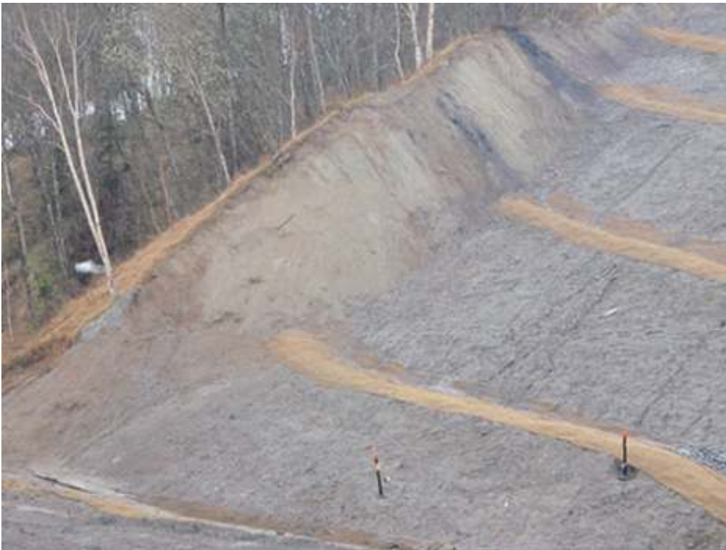
Photo 21 Lack of biological reinstatement (seeding) at KP 348 Krinka could lead to surface soil destabilisation and thus undermine properly implemented technical reinstatement.
