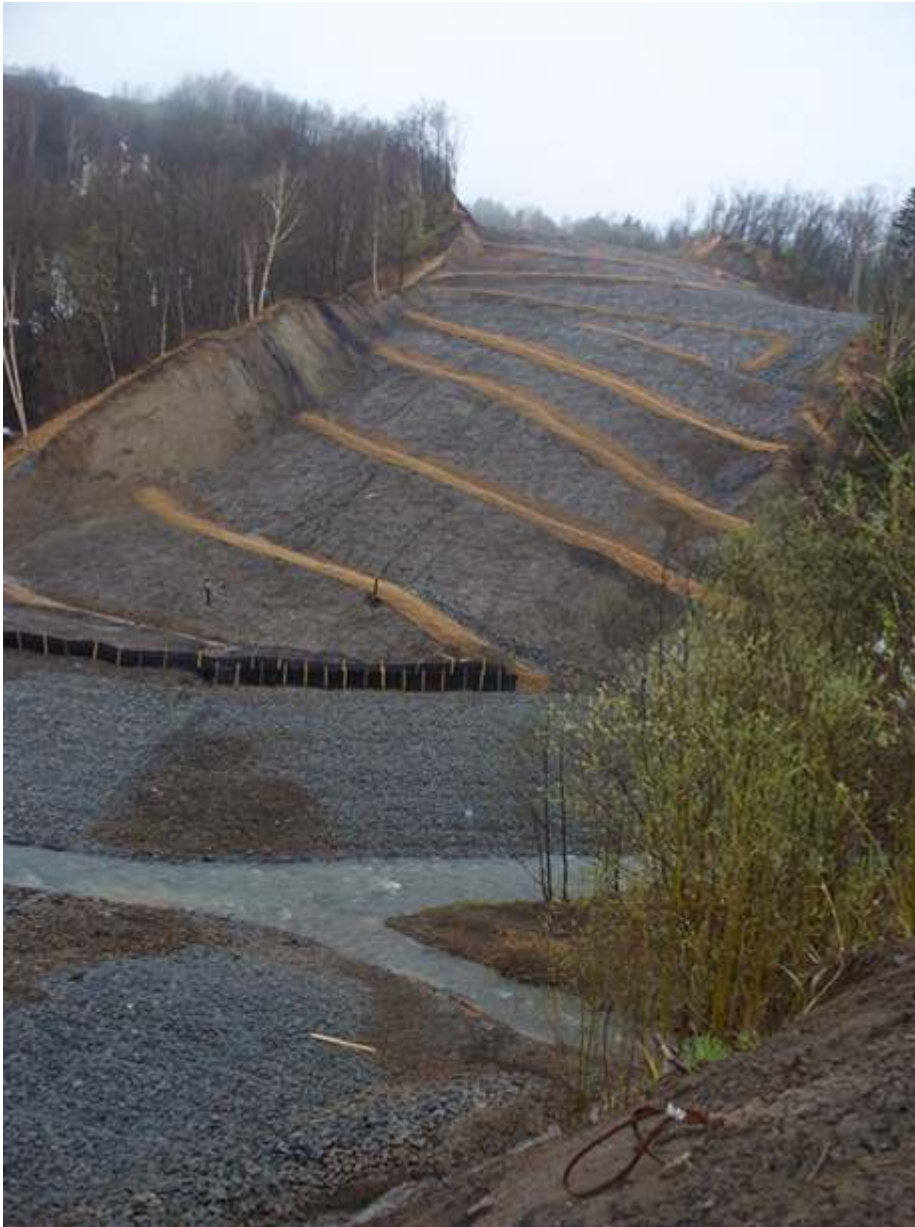
Photo 12 KP 348 Krinka – Effective slope breakers and drainage channels. Small slide on unprotected slope at left and lack of regeneration indicate need to monitor area.
