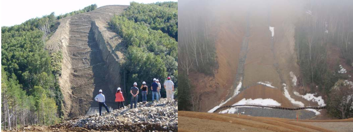
Photo 17 Comparison of KP 345 Gar from September 2008 and May 2009 showing additional geotechnical engineering (new slope breakers, dual side drainage channels, geotextile fabric on side cuts).
