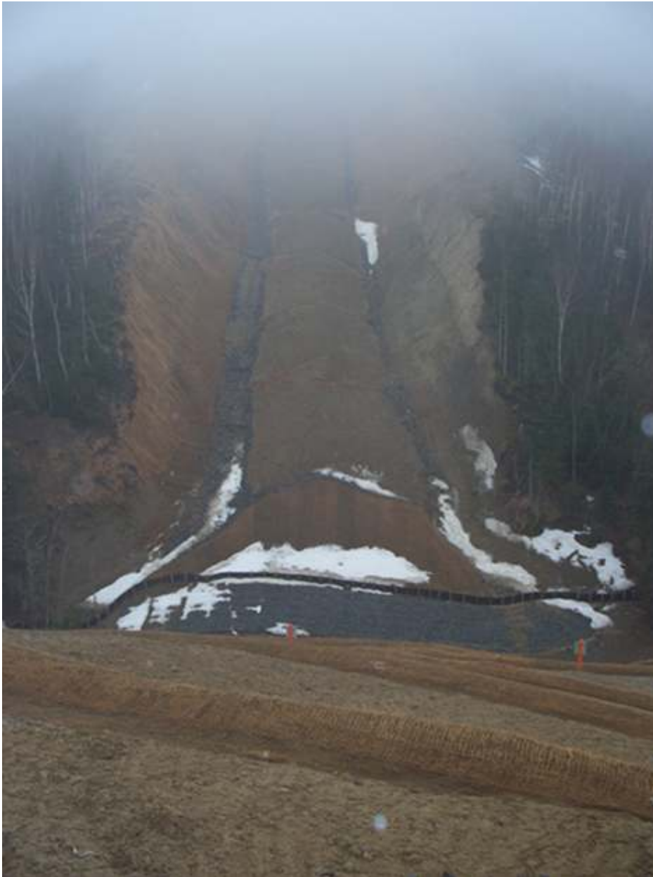
Photo 14 KP 345 Gar – Exceptional stabilisation of steep slope using slope breakers, side drains and geotextile fabric on steepest areas. Sediment visible in both side drains and slight amount of sediment entering river channel on left indicate need to monitor and maintain the area.
