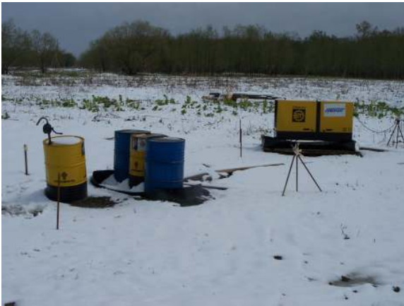
Photo 23 Insufficient secondary containment (of varying levels) at different BVSs. This has been an ongoing issue seen on all spreads.
