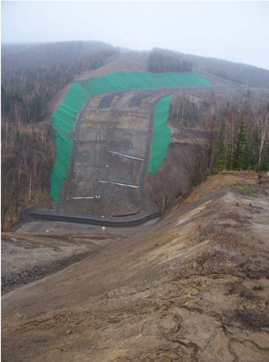
Photo 13 KP 347 Kormovaya – Effective slope breakers with cocomat, riprap side drains, side cuts with geotextile fabric. Small rills forming on unprotected side cut and drain filling with sediment indicate need for future monitoring and possible maintenance.
