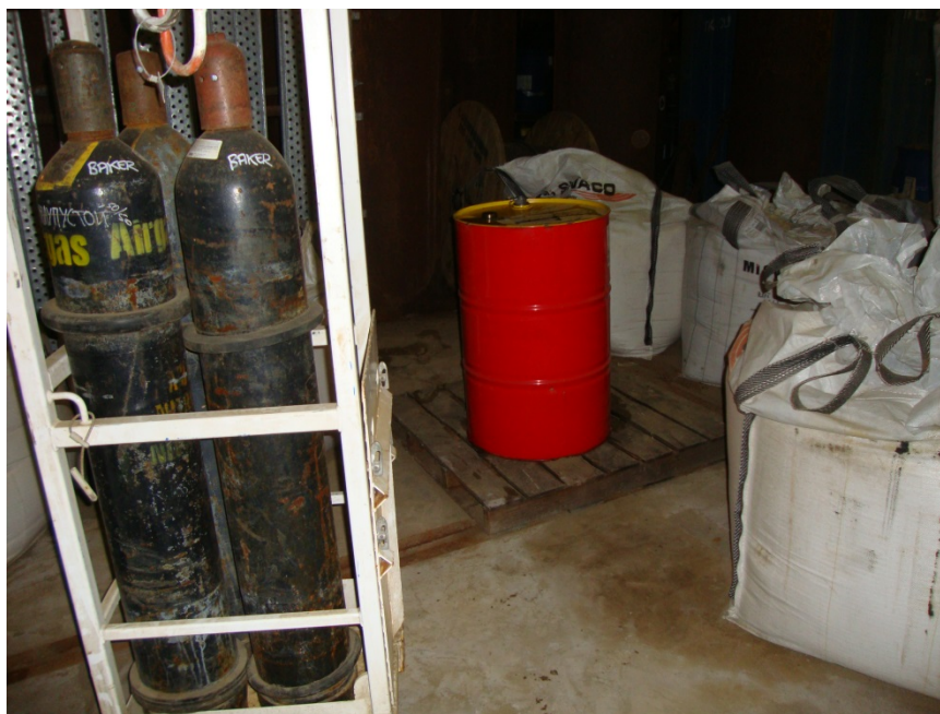
Photo 12. Drum in the 'core' without secondary containment
