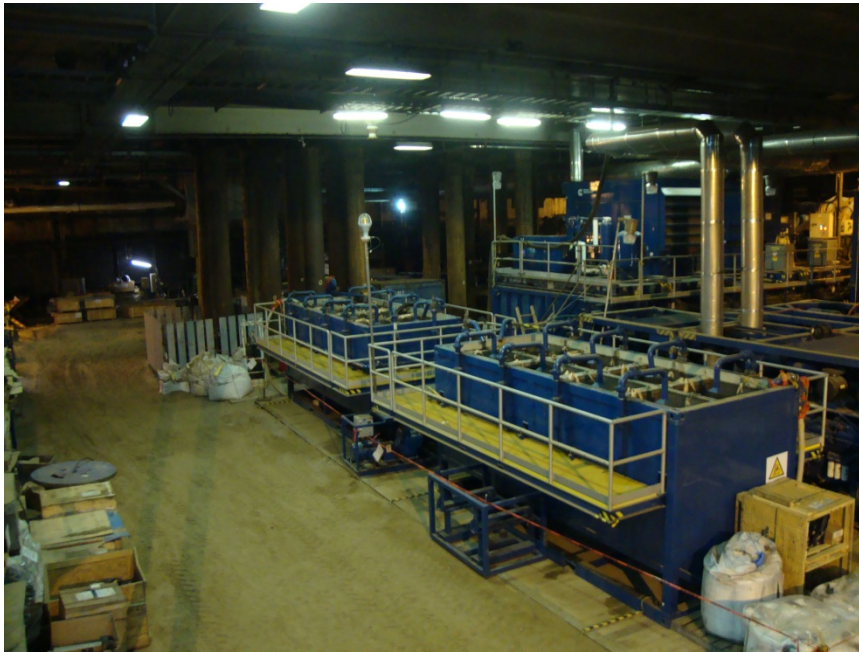
Photo 3. Exhaust ventilation fitted to machinery in the 'core'
