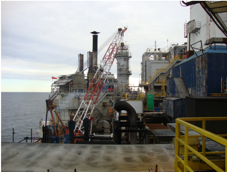
Photo 1. Generator and compressor exhausts
