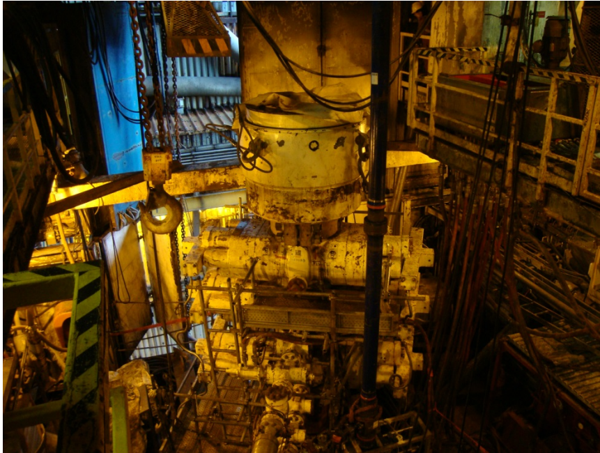
Photo 13. Blow-out preventer (BOP)
