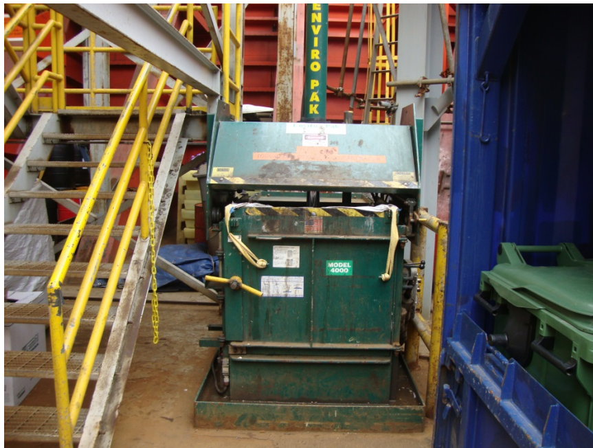
Photo 5. Waste plastic compactor on the main deck
