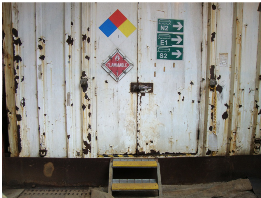
Photo 10. Exterior of main chemical store
