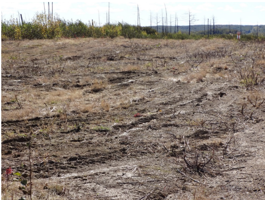
Photo 14: RoW after mechanical tree felling near KP 82
