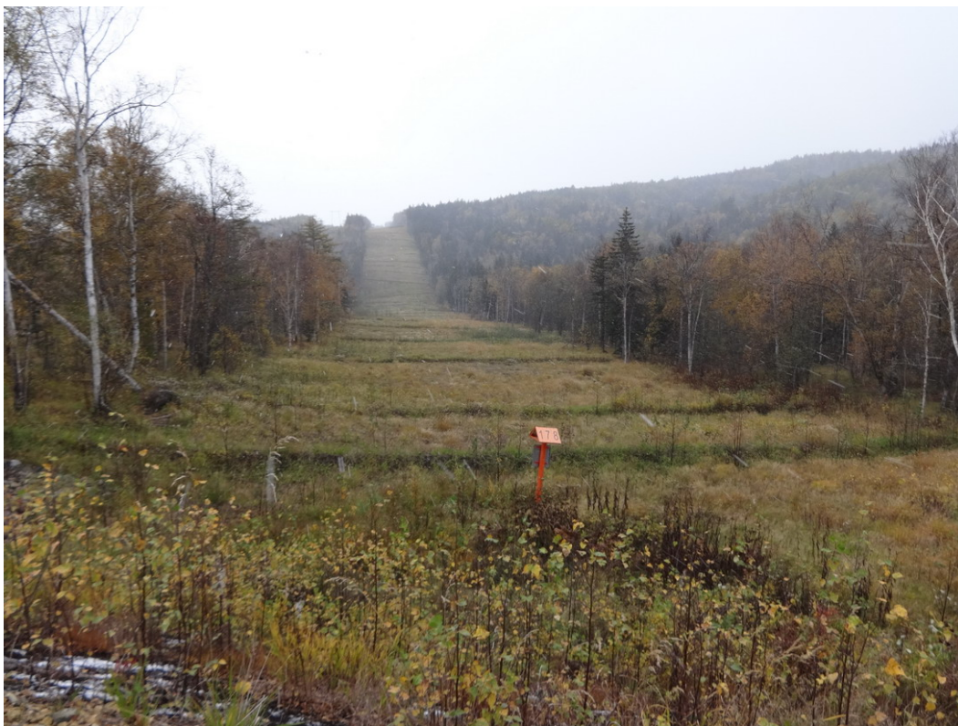
Photo 20: KP 178 Slope with good slope breakers protection
