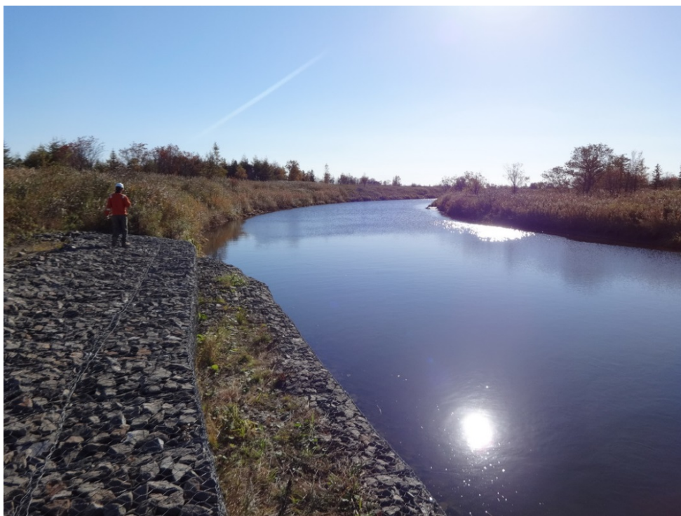
Photo 27: Gabion wall on the south bank of the R. Manui
