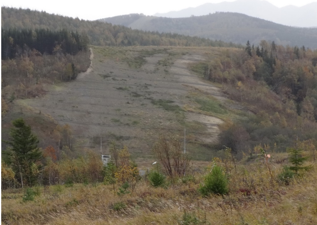
Photo 15: Steep slope at KP 419.5 showing poor vegetation cover
