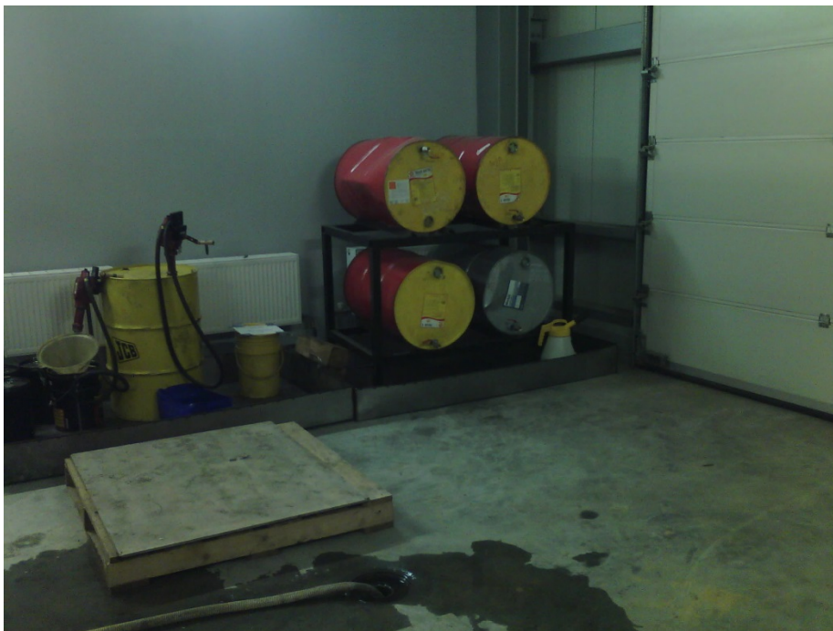
Photo 31: Lube oil and antifreeze storage in the garage workshop
