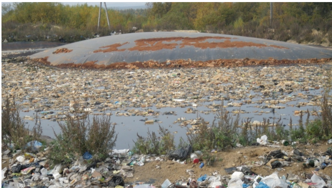
Photo 38: Bubble formed at municipal waste leachate pond
