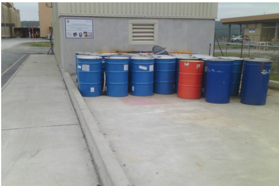
Photo 35: Storage of empty waste drums within a bunded area
