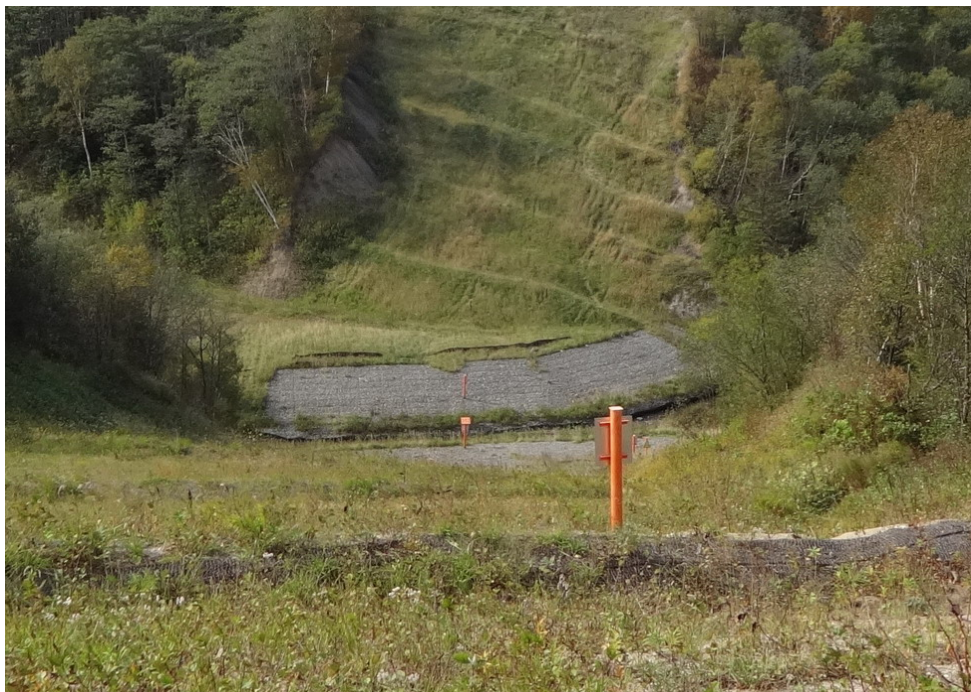
Photo 26: R. Krinka with good re-vegetation and redundant silt fence visible
