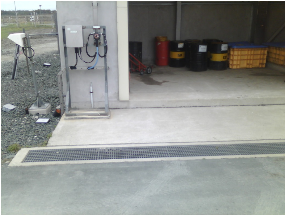
Photo 34: View of entrance to waste storage building
