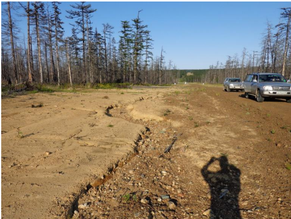
Photo 21: RoW at KP15 in September 2012 showing development of erosion
