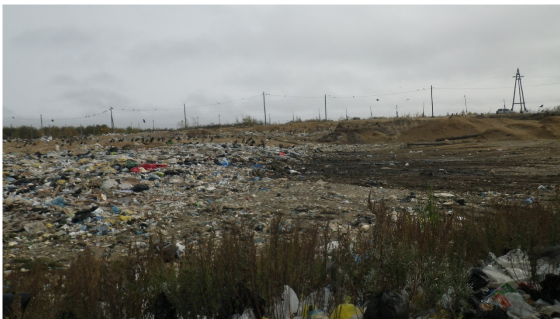
Photo 36: Inadequate daily cover at the Sakhalin Energy waste cell
