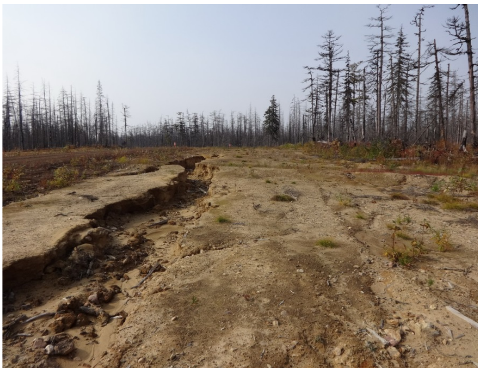
Photo 22: RoW at KP15 in October 2013 showing increased development of erosion
