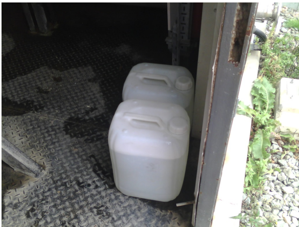
Photo 33: Containers of an unknown substance at the wastewater treatment plant with no secondary containment or MSDS
