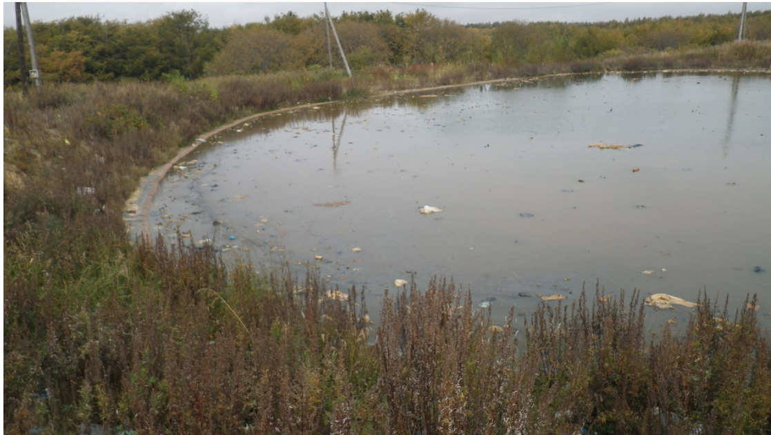
Photo 37: Overflow leachate pond at the Sakhalin Energy waste cell
