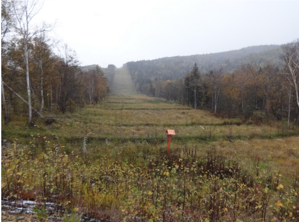
Photo 23: Slopes of the R. Devyataya at KP 178 showing dense vegetation on geojute fortified slope breakers
