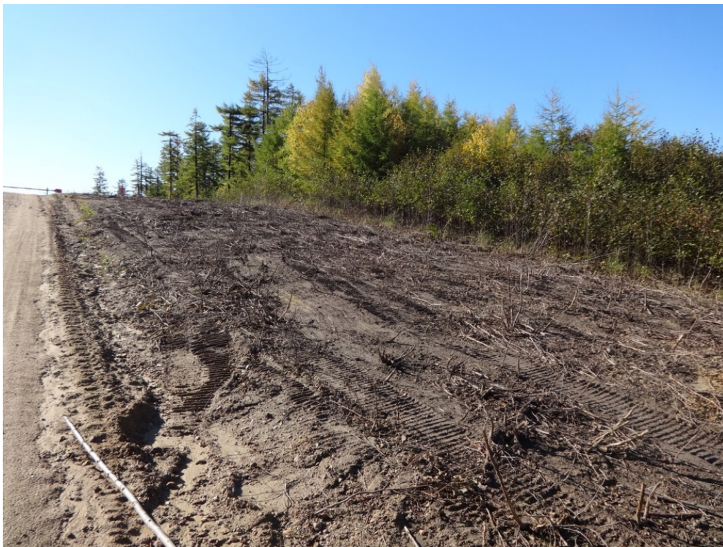
Photo 13: RoW after mechanical tree felling near KP 63
