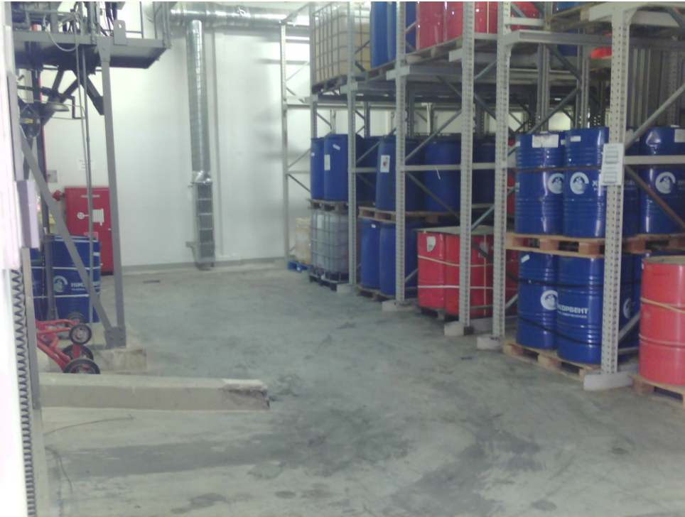
Photo 32: Lube oil storage building showing ramp down into secondary containment area
