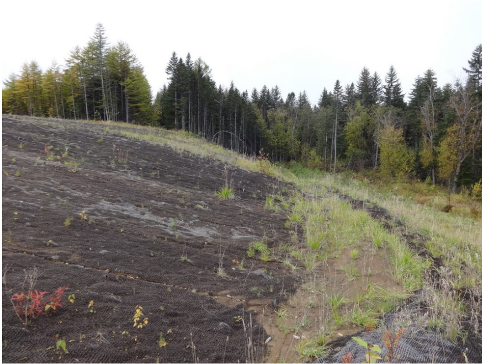
Photo 24: RoW slopes leading to an access on the at KP 180
