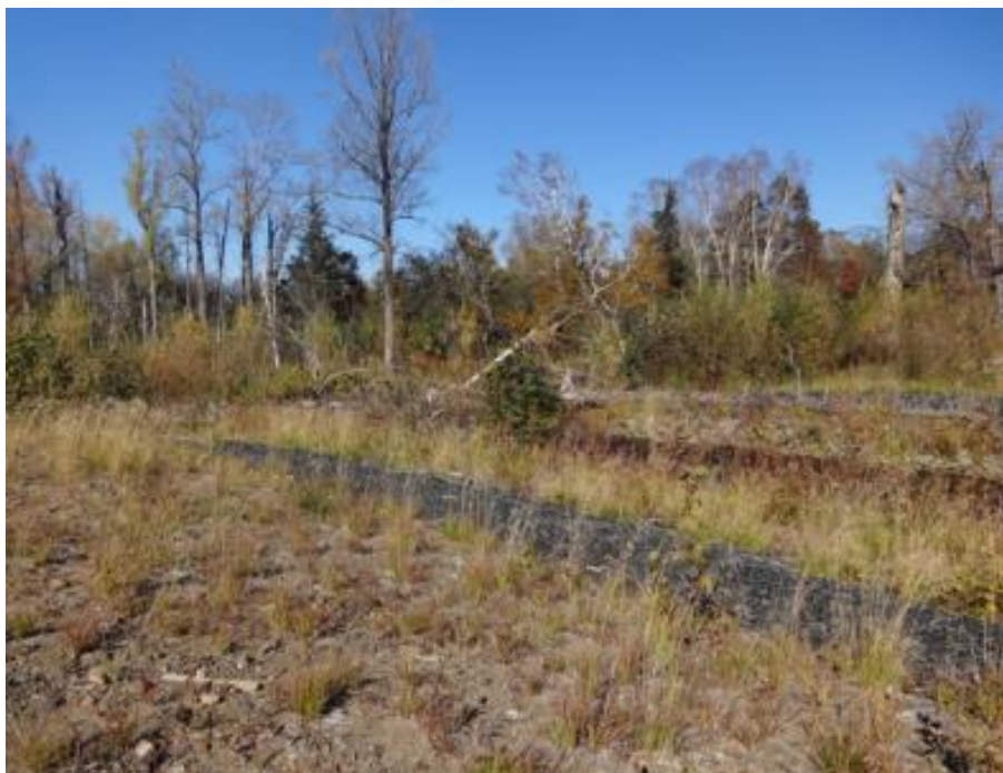
Photo 3.17: Use of Enkamat within Reno matting at the Plelyarna River
