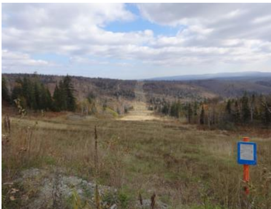
Photo 3.16: Well vegetated slopes on geojute at KP47
