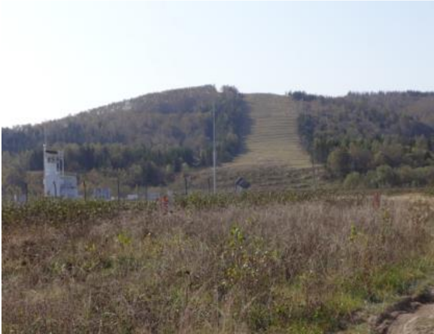
Photo 3.5: Steep slope at KP 422.5 showing good vegetation cover on steep slope
