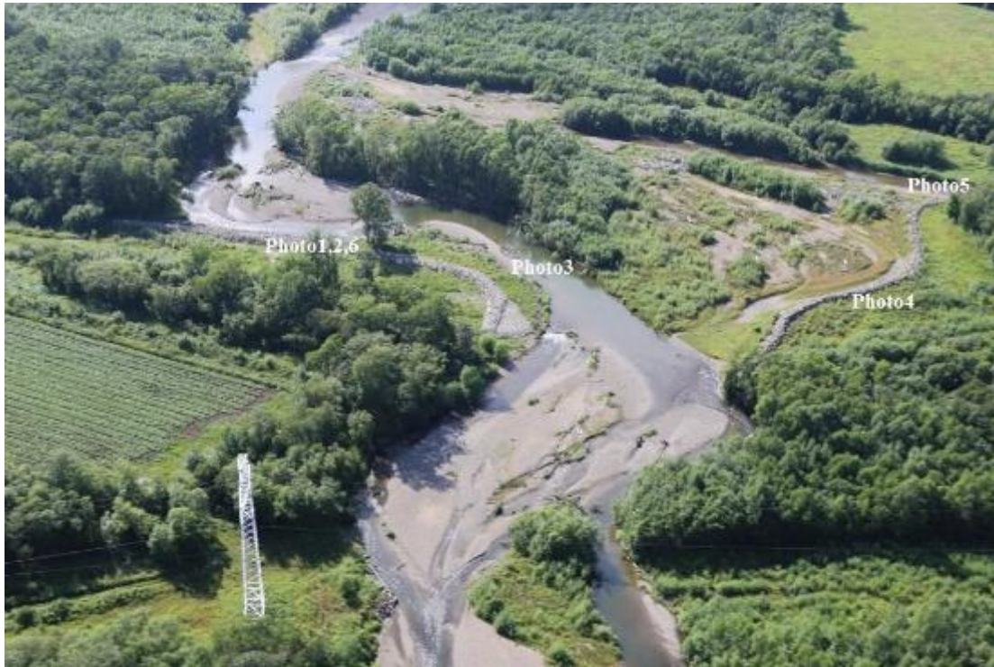
Photo 3.19: Aerial photo showing the Nitui and newly installed riprap walls
