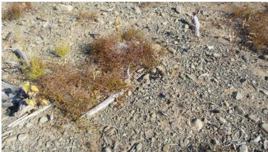
Photo 3.12 : Poorly revegetated RoW as a result of dewatering
