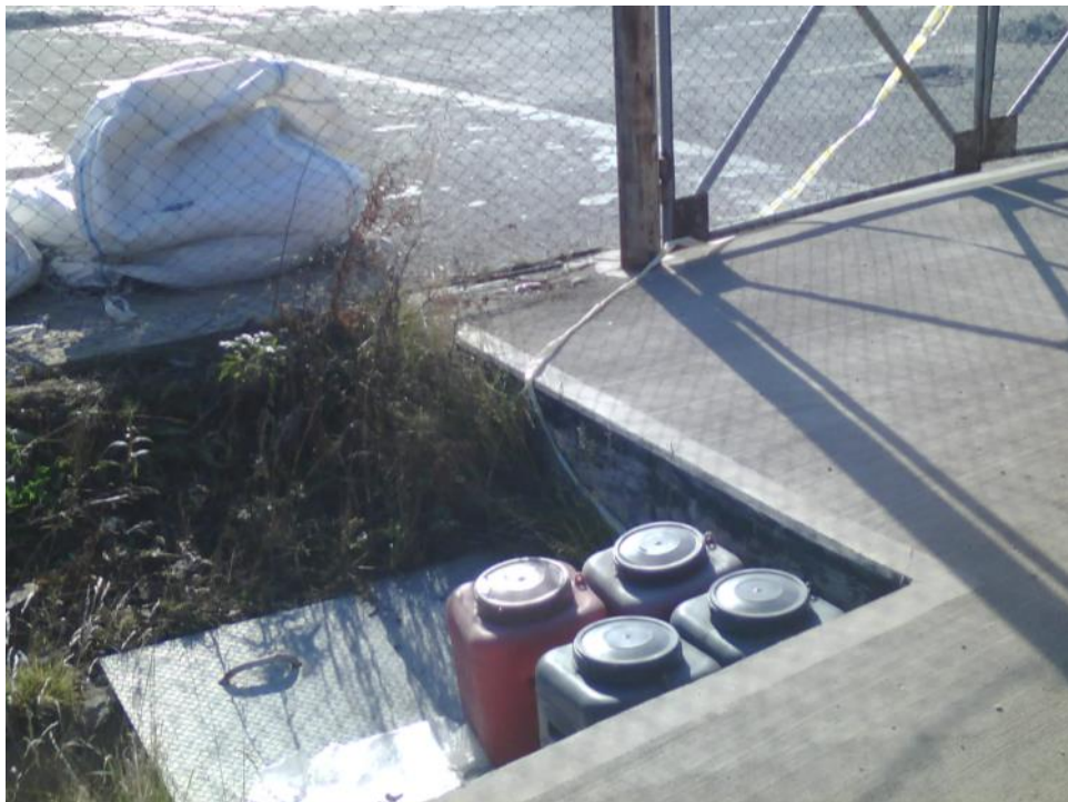
Photo 4.2 Empty PAC Containers stored above the stormwater drain
