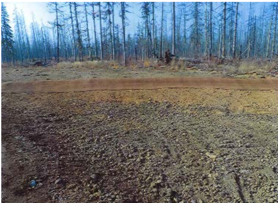
Photo 3.15: RoW at KP15 in October on 21 st October 2013 showing repair and improvement works
