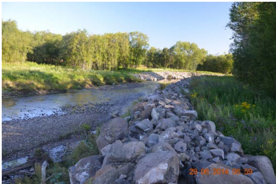
Photo 3.20: Ground photo showing the Nitui and newly installed riprap walls
