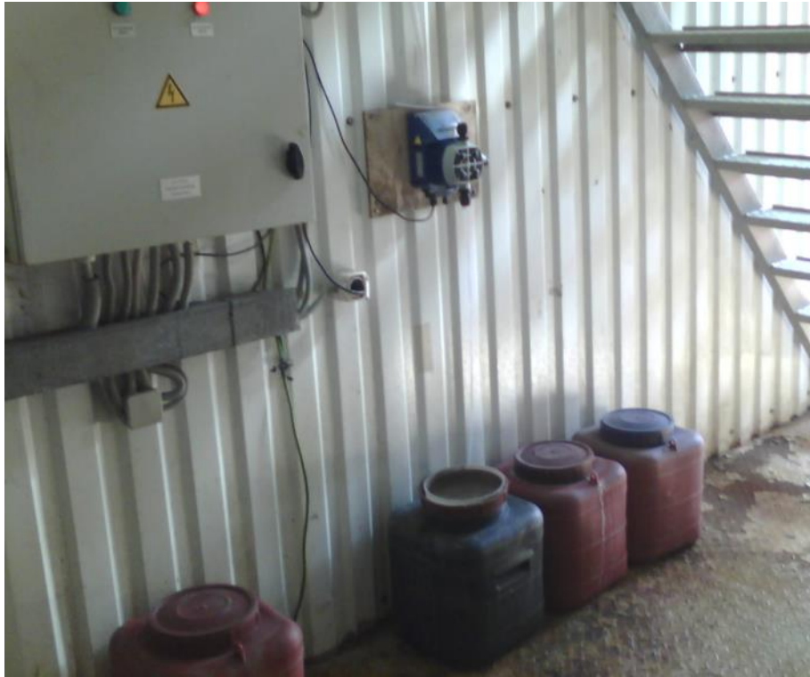
Photo 4.1 Unlabelled containers stored without secondary containment at BR-200
