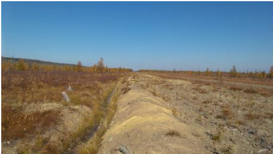
Photo 3.11 Photo 3.11: Ditch and Berm on west of RoW near KP231 preventing water from reaching RoW or wetland to east of RoW.
