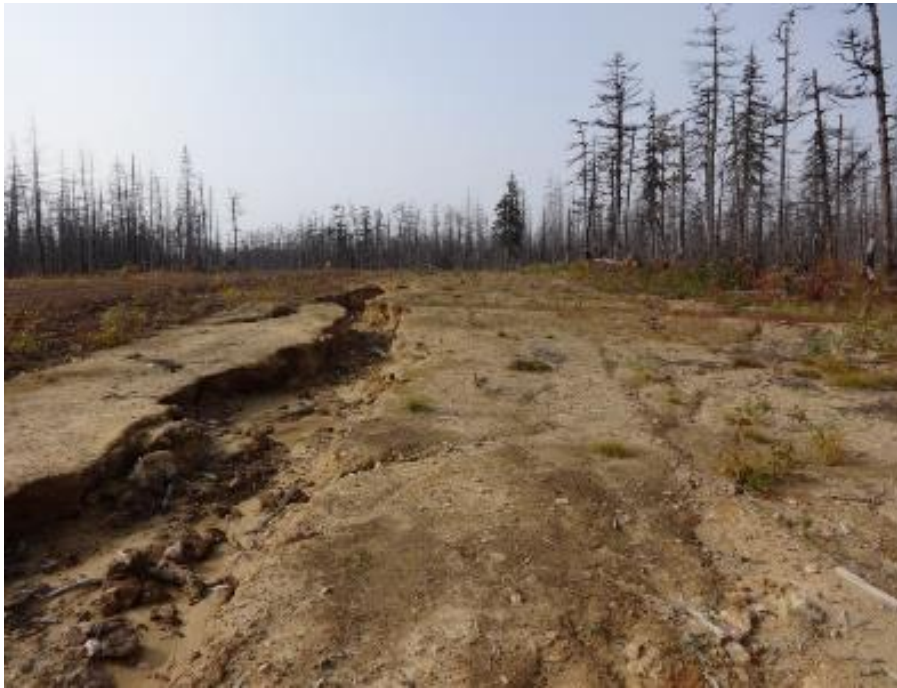
Photo 3.14: RoW at KP15 in September 2013 showing development of erosion
