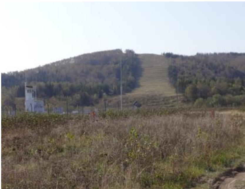
Photo 3.13: KP 422.5 Slope with good slope breakers protection
