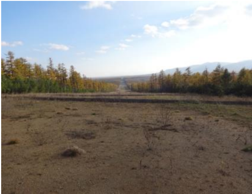
Photo 3.6: Sandy slope at KP 128 showing good vegetation cover beyond the first slope breaker
