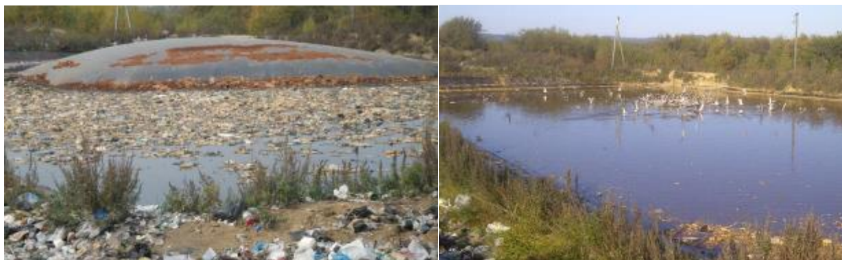
Photo 3.5 Bubble in the Municipal Cell Leachate Pond at Nogliki (Comparison of 2013 and 2014)
