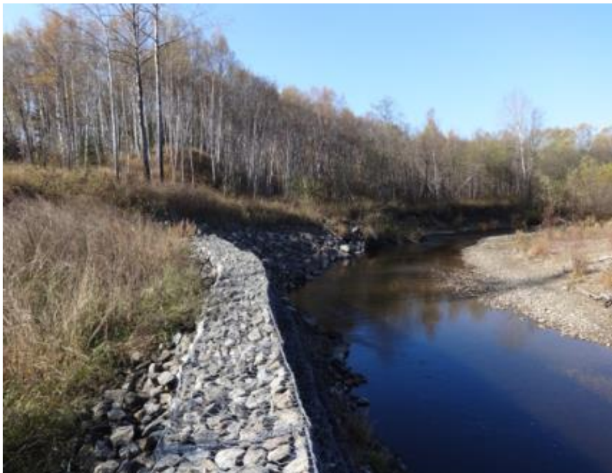
Photo 3.18: Gabion wall on the south bank of the R. Podbiedenka
