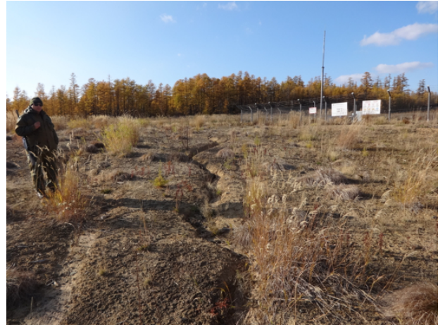
Photo 4 – Area adjacent to the block valve shows poor ground cover and erosion
