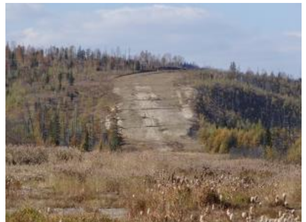
Photo 4 – View south showing RoW slope with slope breakers and erosion. Also wetland fauna in the foreground.
