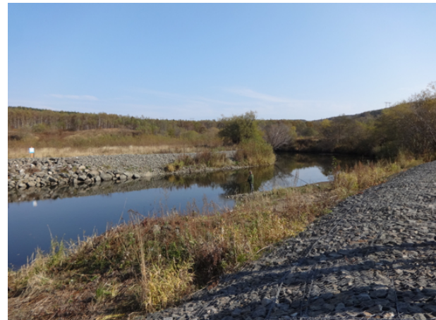
Photo 2 – View downstream showing reno matting and riprap
