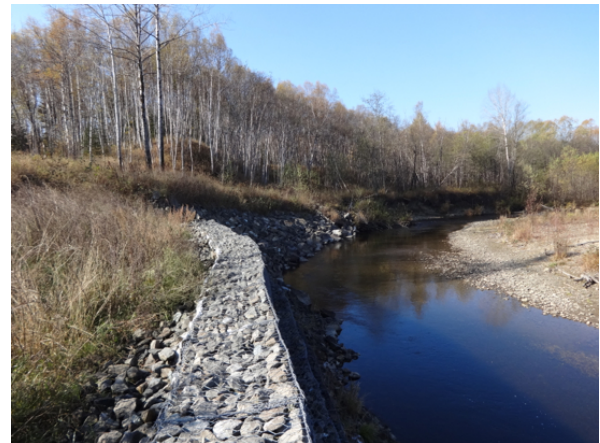
Photo 2 – View to the upstream showing gabion wall and riprap protection
