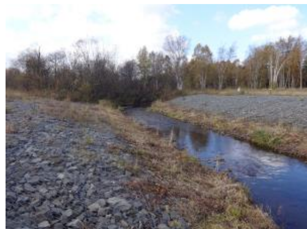
Photo 4 – View to the downstream showing reno matting on the riverbanks
