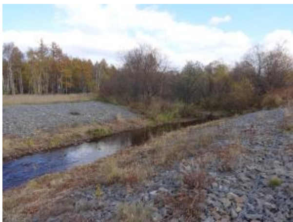
Photo 3 – View to the upstream showing reno matting on the riverbanks
