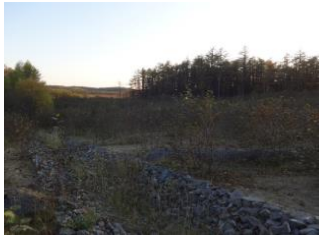
Photo 1 – View south from the Block Valve showing dense growth of Alder on the RoW
