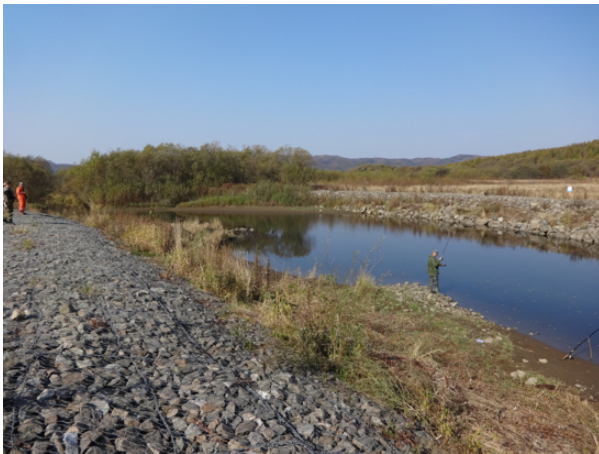
Photo 1 – View upstream showing reno matting and riprap
