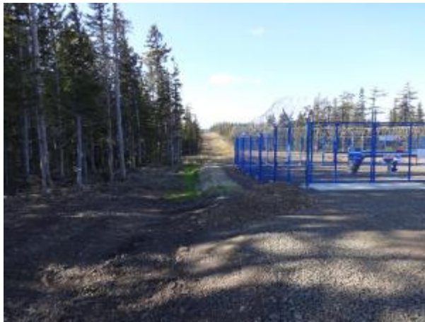
Photo 1 – View north of the east side of the Tie-In
