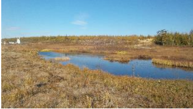
Photo 3 –Sedge fringed pool formed over pipeline
