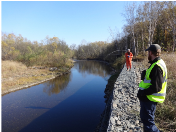
Photo 1 – View to the downstream showing gabion wall and opposite bank
