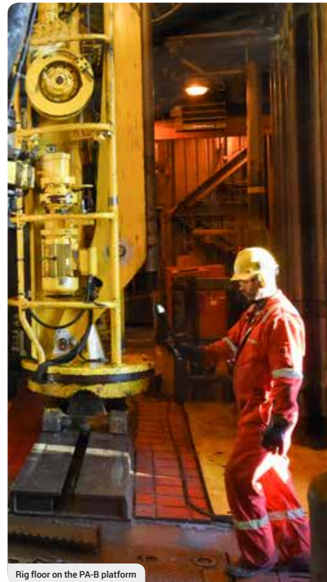
Rig floor on the PA-B platform
