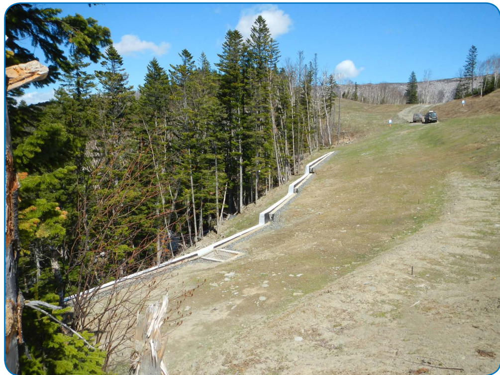
The pipeline right of way, strengthening the landslide area, Makarov district
