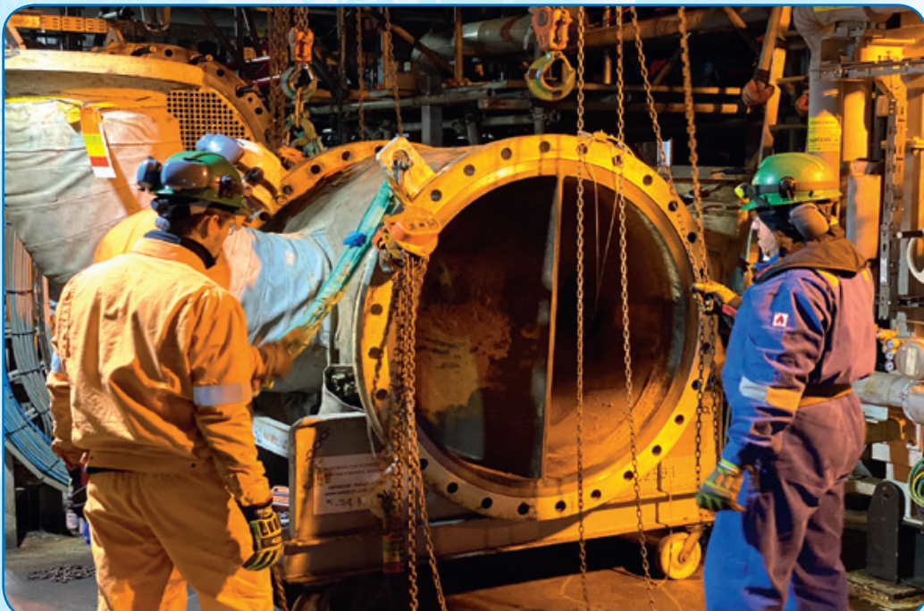
Complex lifting operations
