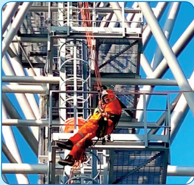
Inspections of the flare derrick structure assemblies
