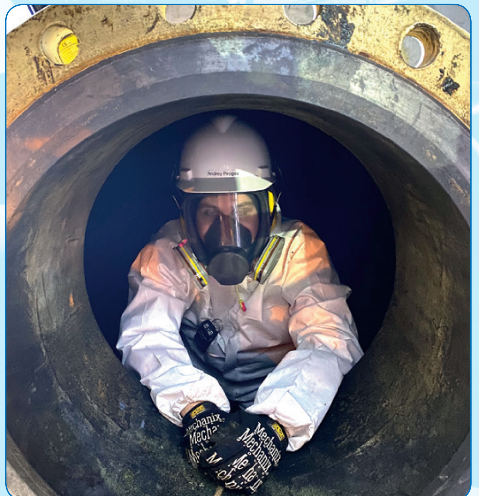
Confined space work
