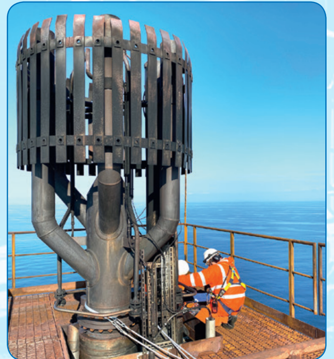
Electrical work in the flare zone
