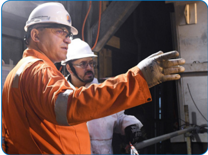
Replacement of equipment at LNG plant
