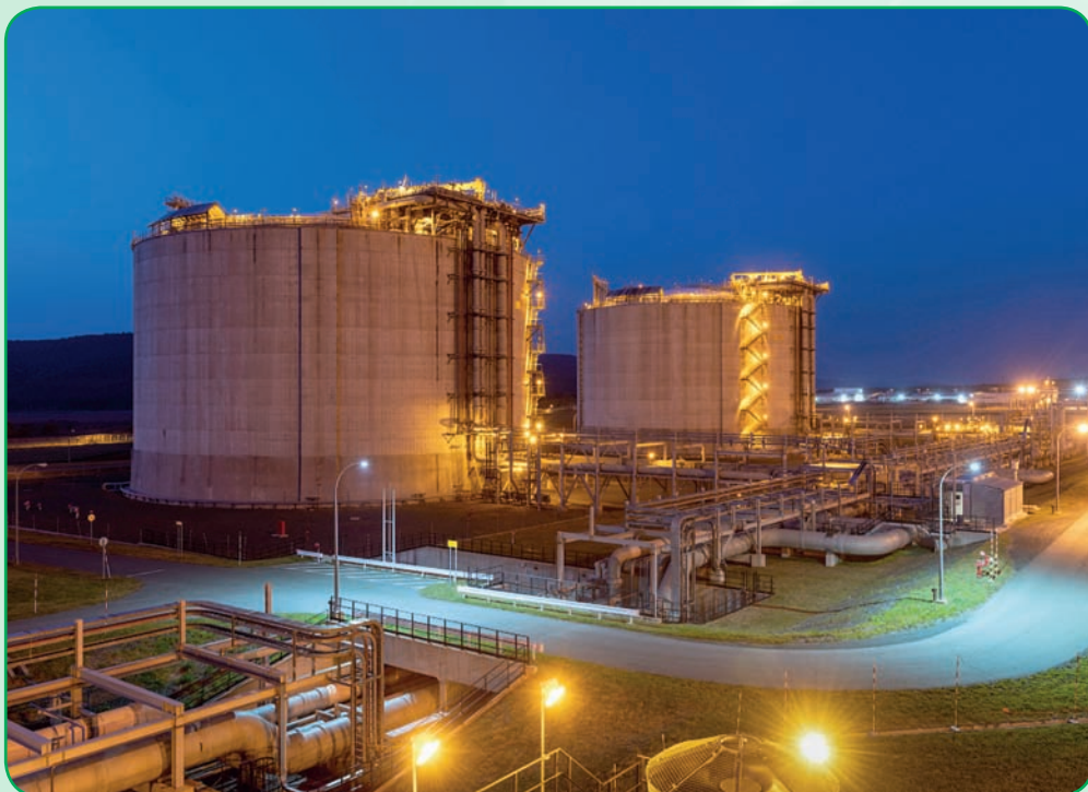
LNG storage tanks. Prigorodnoye production complex
