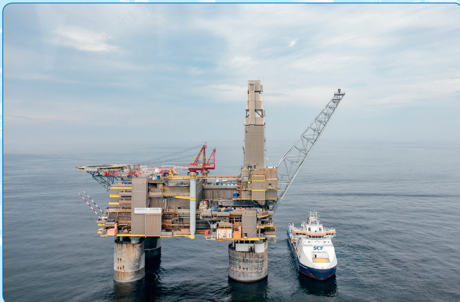
Offshore gas production platform LUN-A
