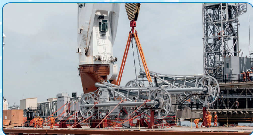
The new 77-tonne loading arms were manufactured by the Japanese company TB Global Technologies Ltd
