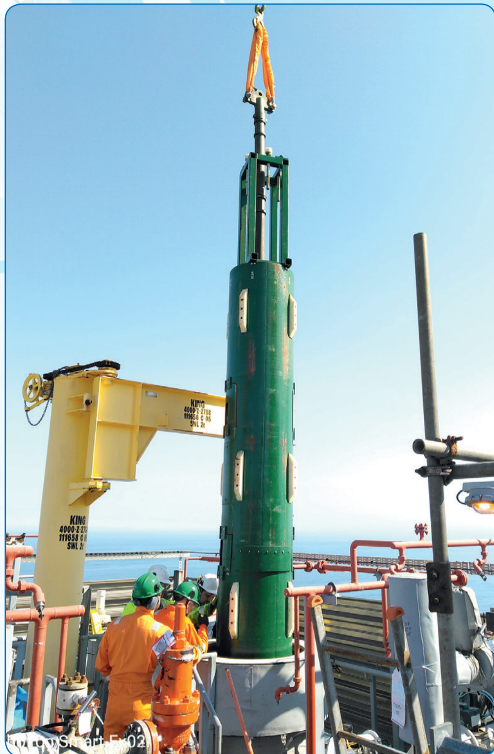
Installation of a remotely controlled isolation device Remote Techno Plug at the Lunskeye-A
