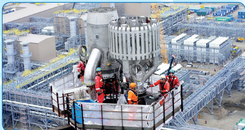
Replacement of flare tips at the OPF
