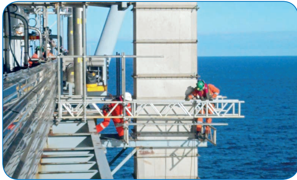
Construction of scaffolding to repair ventilation ducting on PA-B platform
