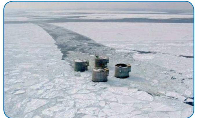
Gravity base condition monitoring, March 2005
