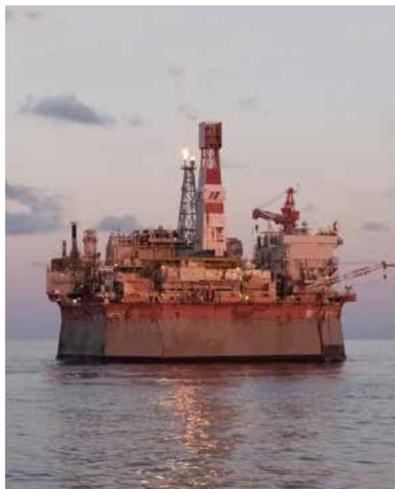
able to rotate 360 degrees, tankers can moor from the leeward side in any weather. This design allows operation of the equipment in low temperatures, storm waves, during strong wind gusts and seismic activity.
